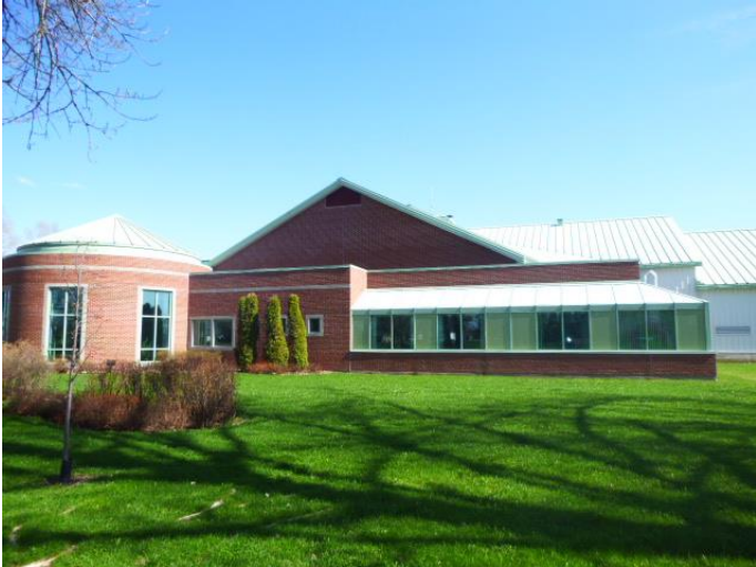
Front view – Center
