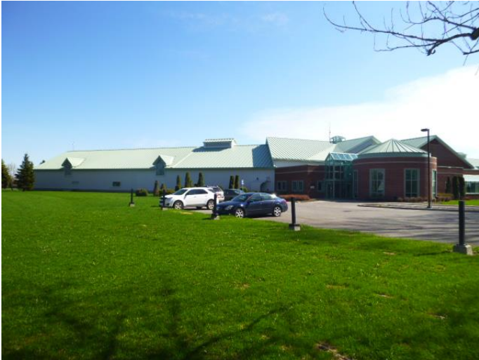
Front view – East
