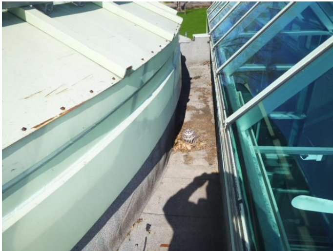
Flat roof front view – East
