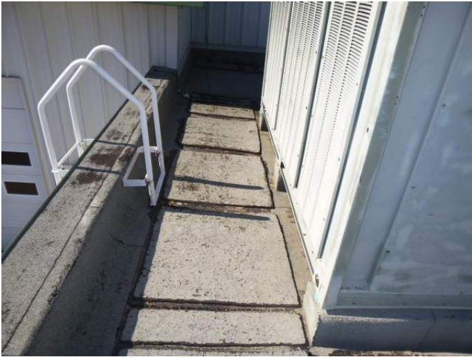
Flat roof rear view – East
