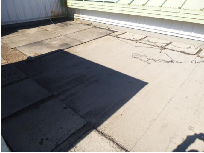
Flat roof rear view – East
