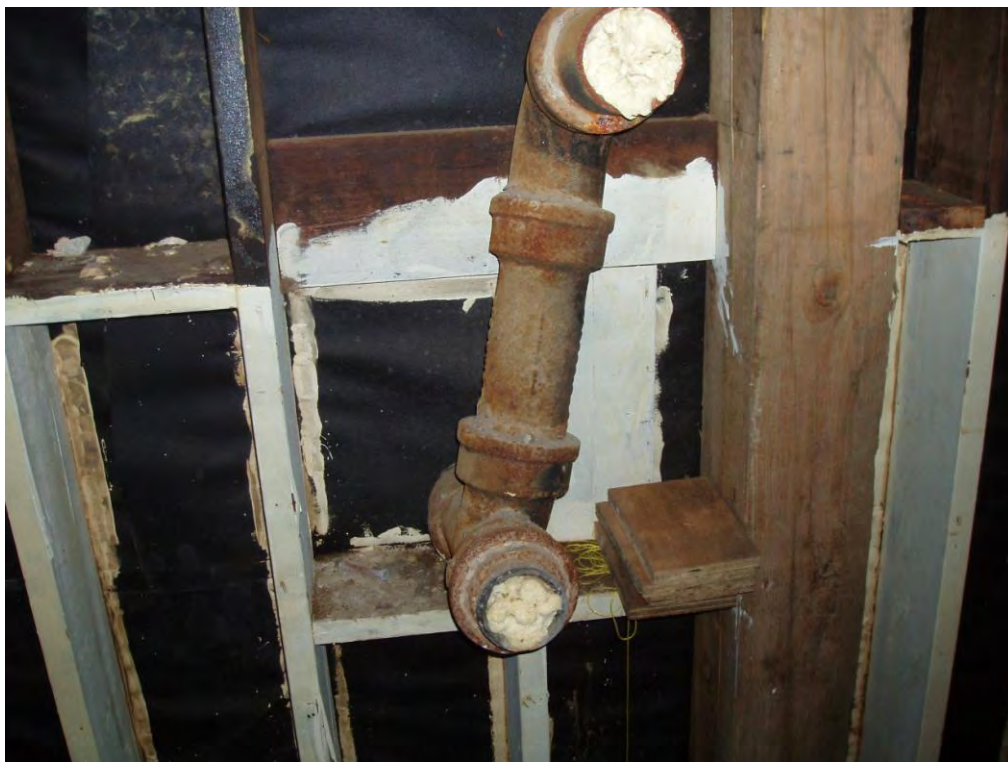
Figure 12 : Old sewer connection
