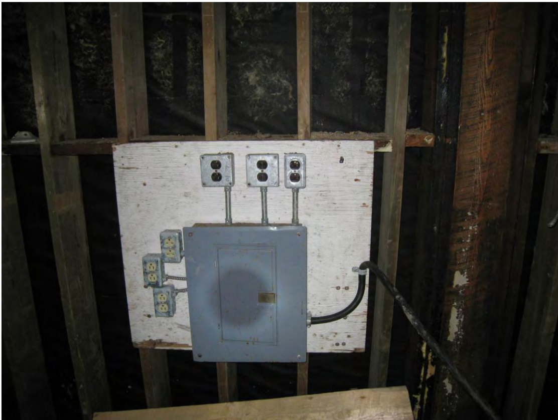
Figure 17 : Temporary Power circuit box, east wall
