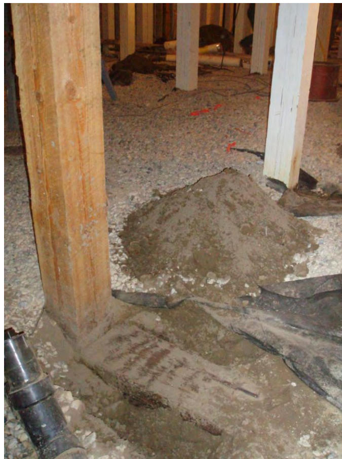
Figure 20: Buried sleeper beam supporting old column
