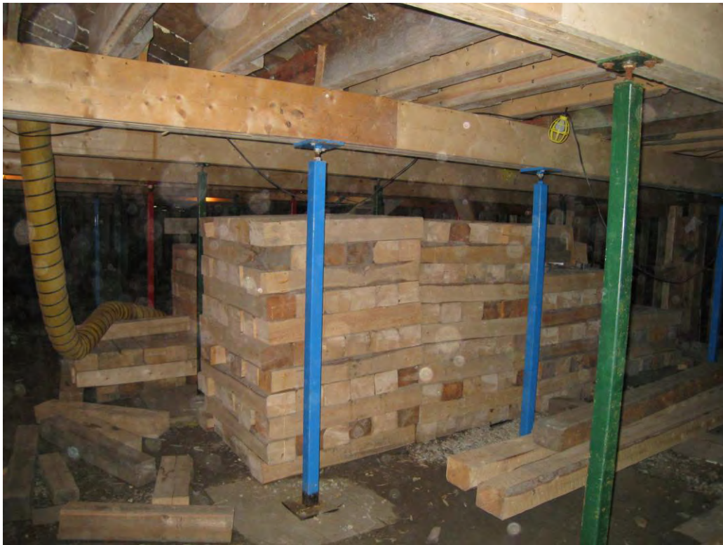
Figure 11: Blocking available in basement
