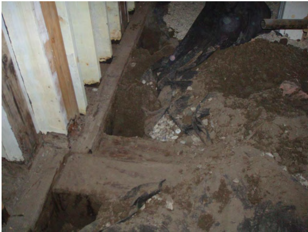
Figure 19: Buried sleeper beam at foundation wall
