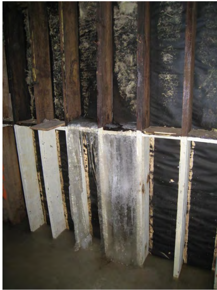
Figure 5: Spring seepage through foundation wall
