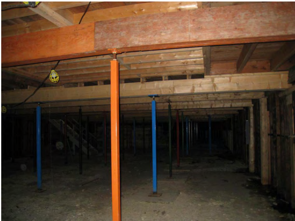
Figure 2: Basement after joist and column replacement
