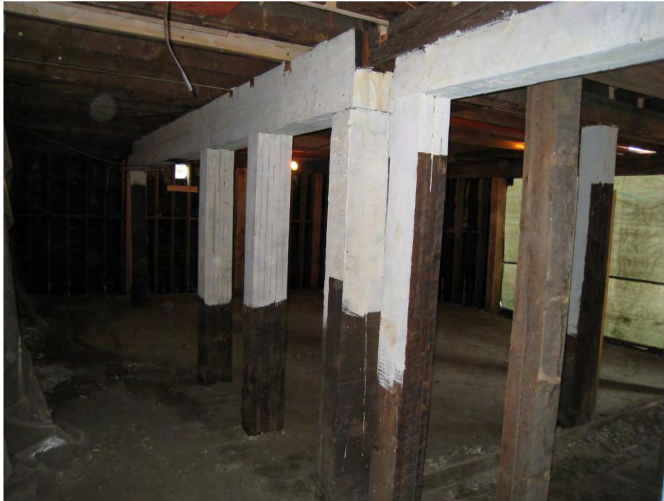
Figure 1: Basement prior to joist and column replacement
