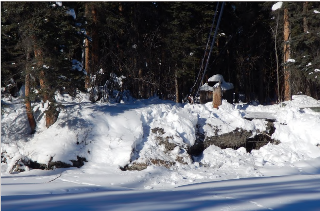
Photo 6: Overview of the north bank and the ferryway structure with the scour zone visible below. The top of bank is about 1.8 m above the ice. The scour is confined to this photo. Photo Taken March 4, 2014
