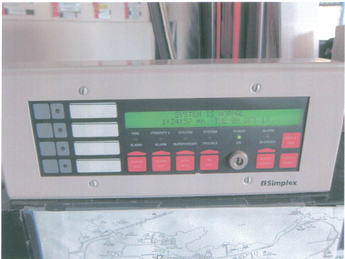
PHOTO 5 - E8 EXISTING CONSOLE RM 102 - FIRE ALARM ANNUNCIATOR
