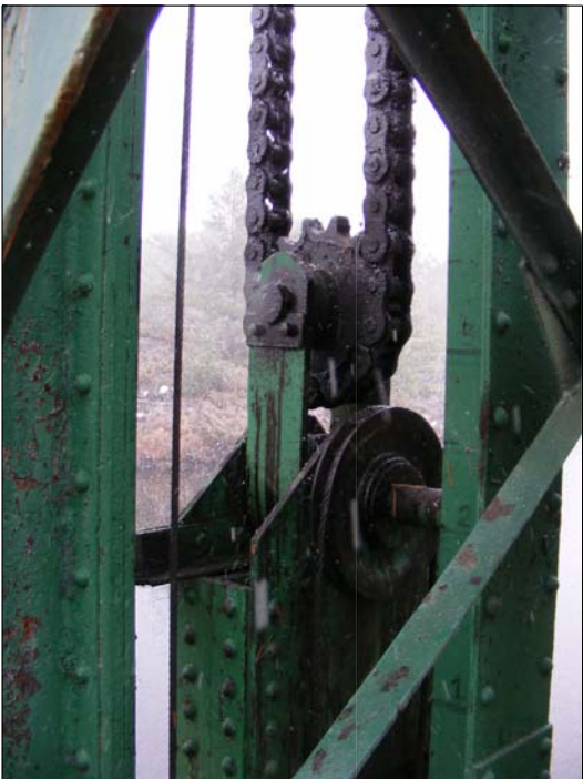
26 CHAIN SPROCKET AND GATE GUIDE ASSEMBLY H16
