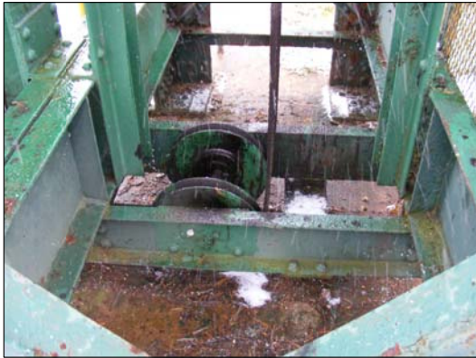
37 H16 COUNTERWEIGHT GUIDE CABLE AND SHEAVES
