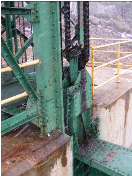
27 GATE HANGER AND CHAIN SPROCKET H16
