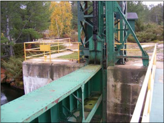
36 H16 NORTH DAM – SOUTH ABUTMENT SHOWING GATE HANGER AND TOWER
