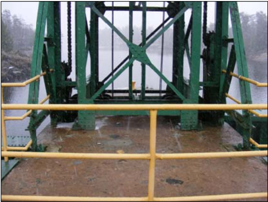
38 H16 CENTRE TOWER CROSS-BRACE WITH GATE GUIDE ASSEMBLY (TOP) AND COUNTERWEIGHT SHEAVES
