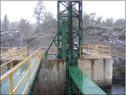
35 H16 NORTH DAM NORTH ABUTMENT SHOWING GATE HANGER AND TOWER
