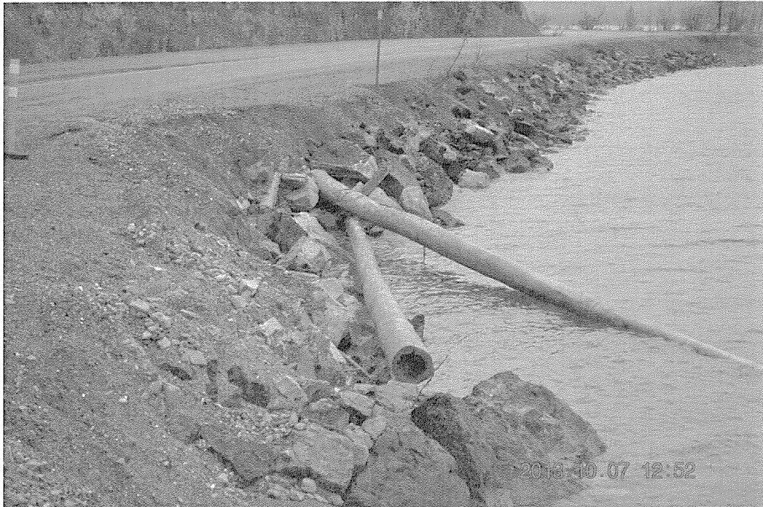
Photo 1: Looking South at Existing Riprap and Logs between Stn. 703+082 to Stn. 703+097.
