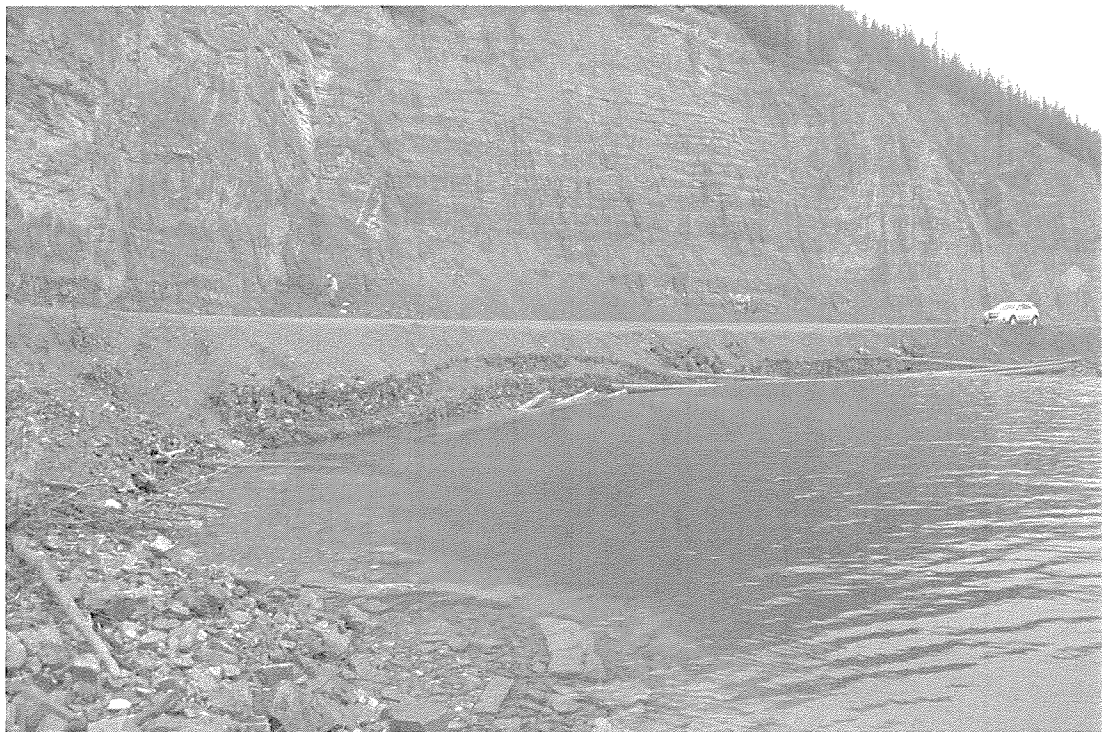
Photo 2: Looking South at Existing Gabions, Riprap, and Logs between Stn. 703+082 and Stn. 703+097.
