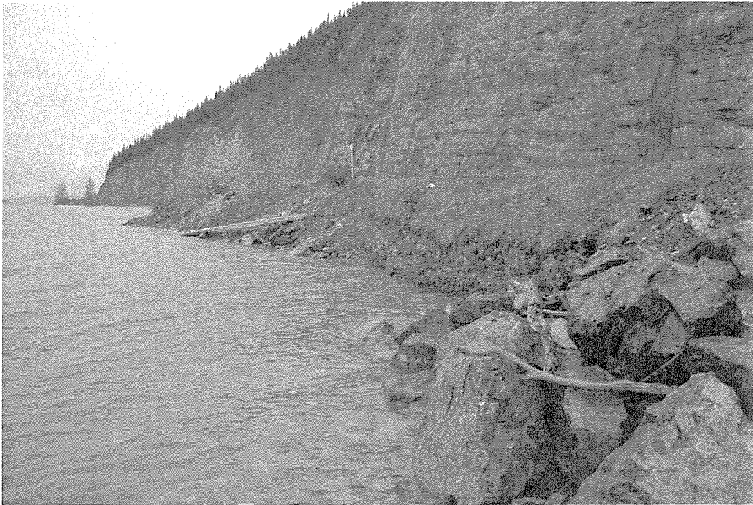
Photo 1: Looking North at Existing Gabions between Stn.701+628 and Stn. 701+646.
