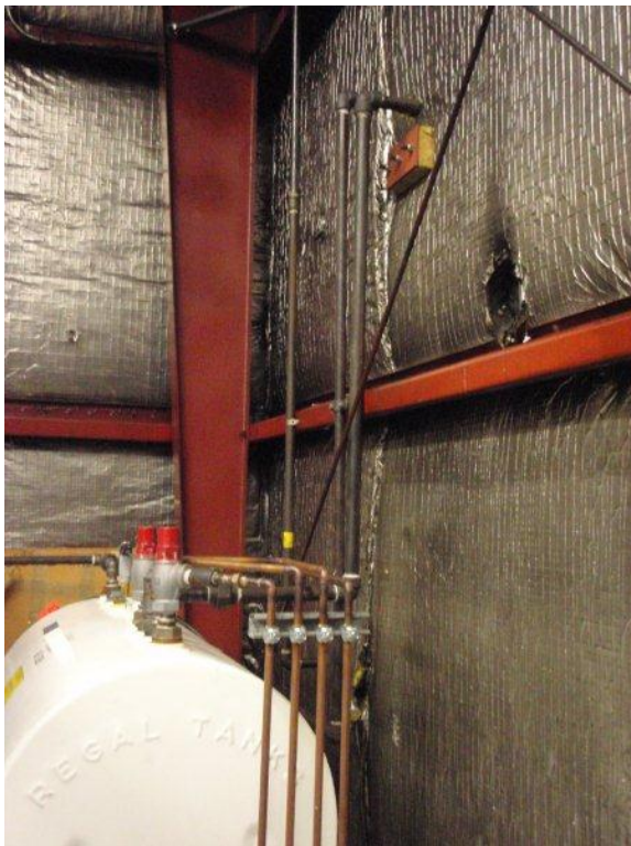
PHOTO 10: PUMPHOUSE BUILDING AND DIESEL AUXILIARY (DAY) TANK Fuel transfer and Overflow/Vent piping
