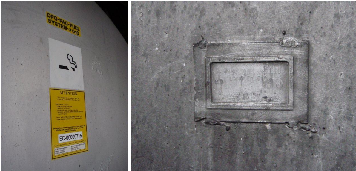
PHOTO 3 & 4: PUMPHOUSE DIESEL FUEL STORAGE TANK Tank labelling and ULC Label
