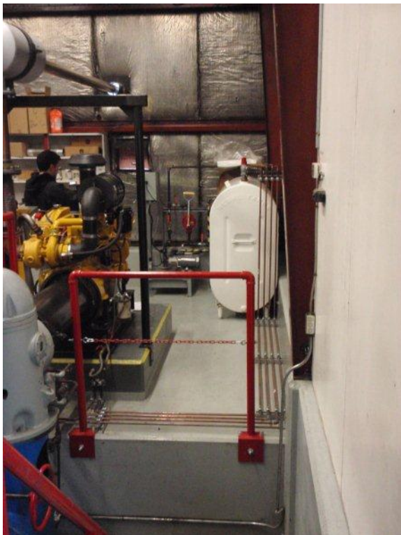
PHOTOS 12: PUMPHOUSE BUILDING AND DIESEL AUXILIARY (DAY) TANK Engine fuel supply and return piping
