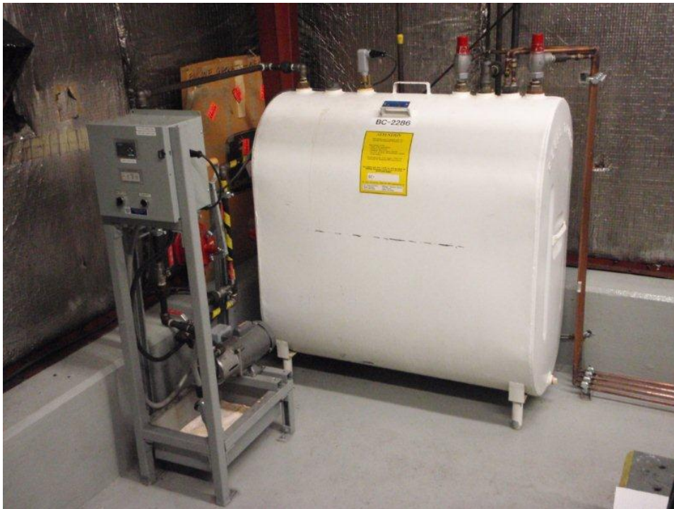
PHOTO 11: PUMPHOUSE BUILDING AND DIESEL AUXILIARY (DAY) TANK Fuel transfer pump and controls
