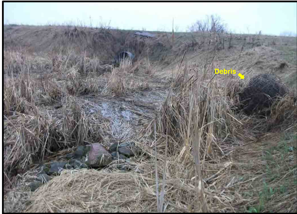
Photograph 3: Landfill #3 - south landfill slope, culvert under site road
