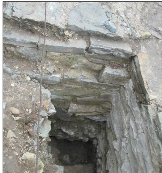
Figure 13: Photograph of the southwest foundation of the Officers' Barracks (photograph by H. Cary;131H657E).
