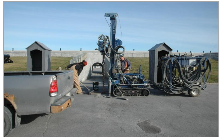
Figure 3: Continuous flight hydraulic auger advancing 131H54L
