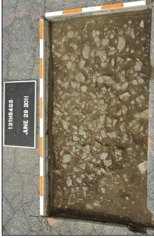
Figure 45: Post excavation plan view of 131H54G3, showing the Macadamized surface (photograph by K. Best; 131H2568E).
