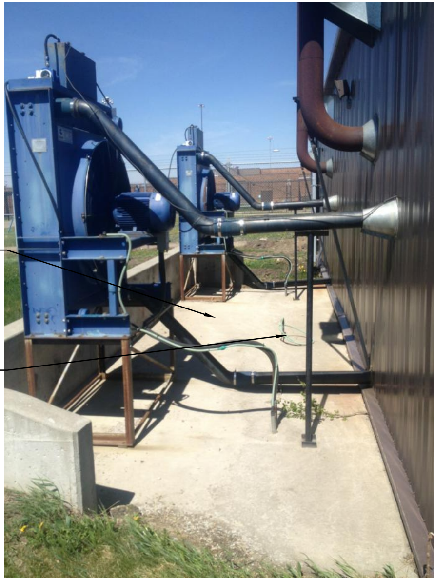
3 REMOTE GENERATOR RADIATORS (LOOKING NORTH) E1 SCALE: N.T.S.
