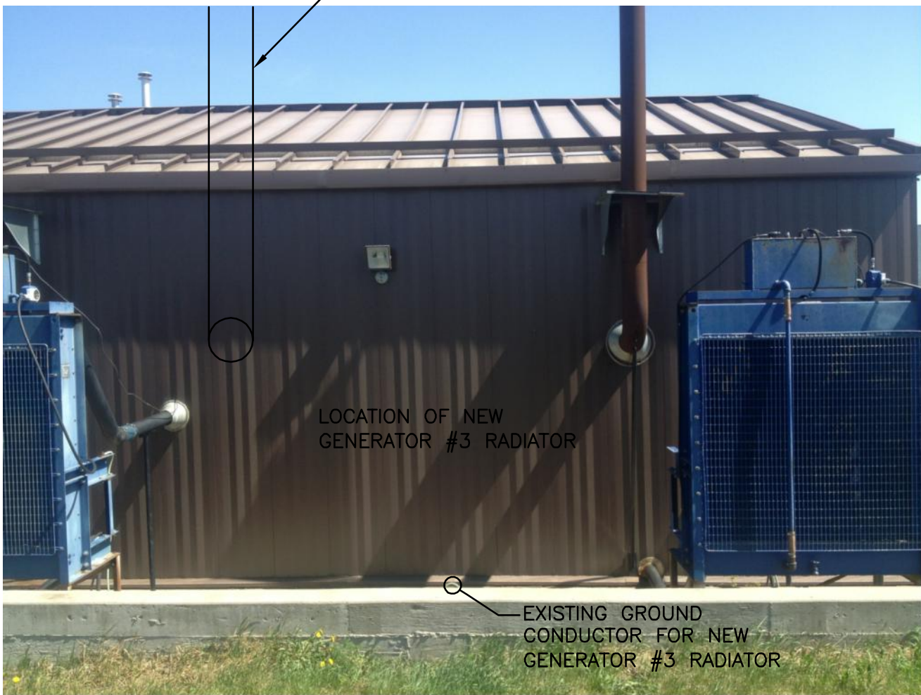
2 REMOTE GENERATOR RADIATORS (LOOKING EAST) E1 SCALE: N.T.S.
