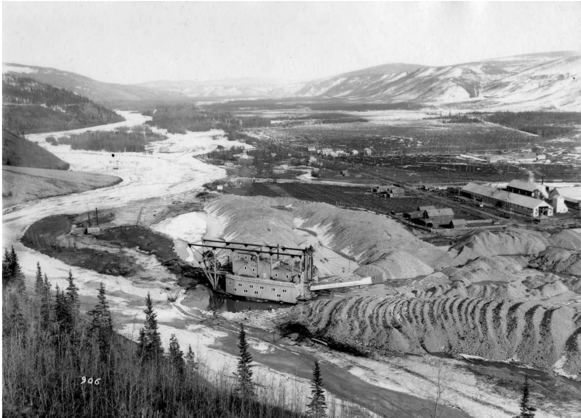
Figure 1: Dredge #4 operating shortly after construction (circa 1914)
