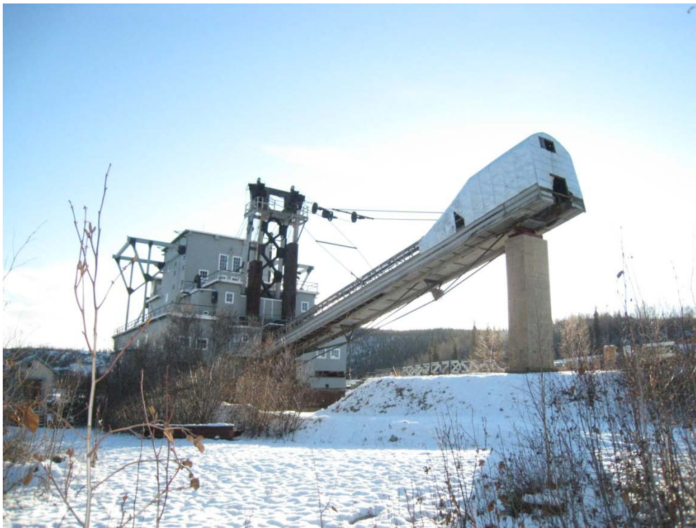
Figure 4: Stacker Arm support
