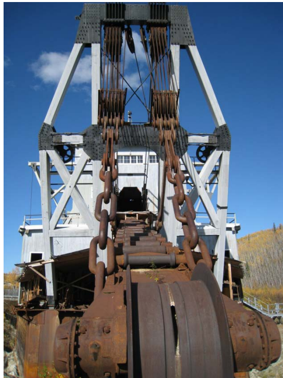
Figure 2: Bow Gantry and Digging Arm
