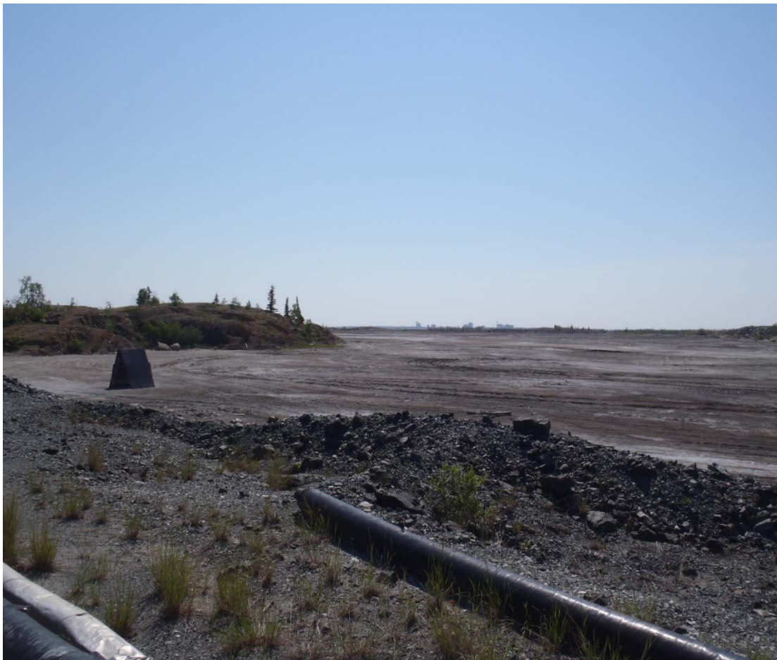
Photograph 1: North end of South Pond, Looking South – July 9, 2013
