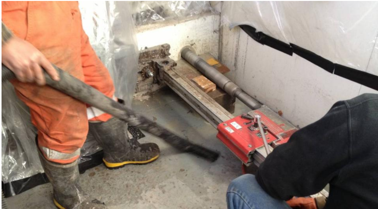
Photo 3: View of CH13-01 advanced through foundation wall.
