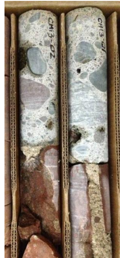
Photo 5: Core of interior concrete curb and foundation wall.
