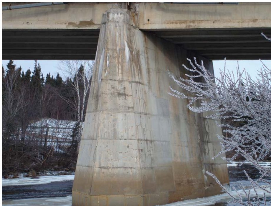
Photo 74 - South End of Pier. Note deteriorated concrete at top.
