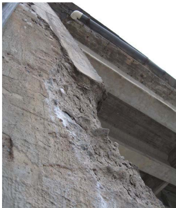
Photo 66 - Severe spalling in South-West corner of West Abutment.
