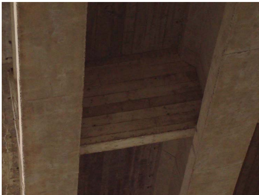
Photo 49 - Typical cast-in-place concrete diaphragm between girders.
