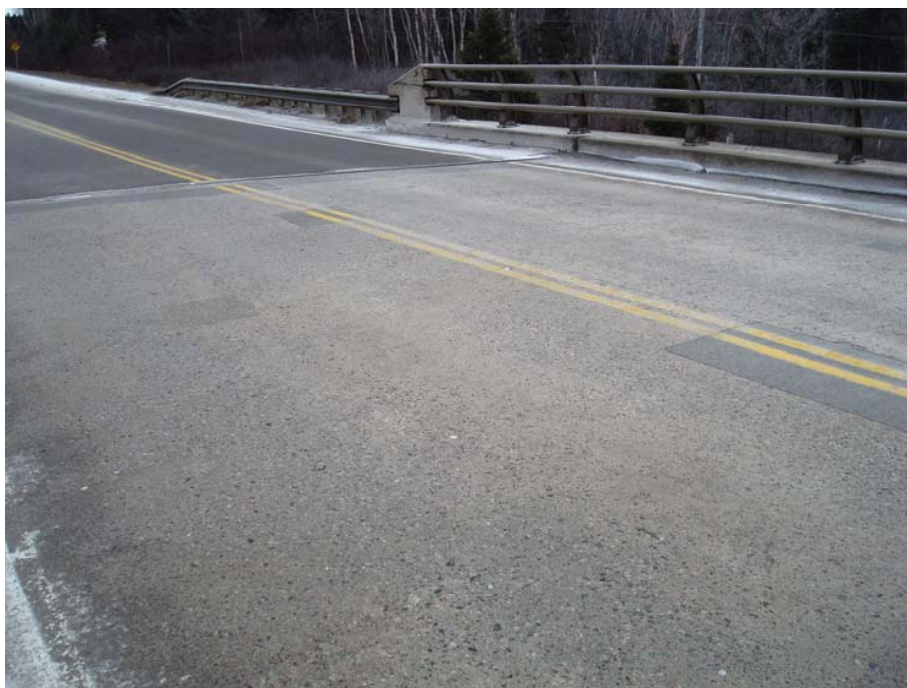
Photo 12 - Exposed concrete deck as wearing surface.
