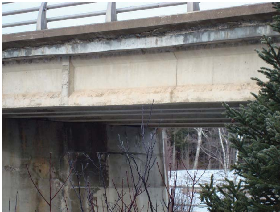
Photo 51 - Side view of typical exterior precast concrete girder.
