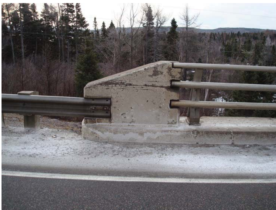
Photo 26 - Elevation view of typical end wall. Note notching for bridge railings and for guardrail.
