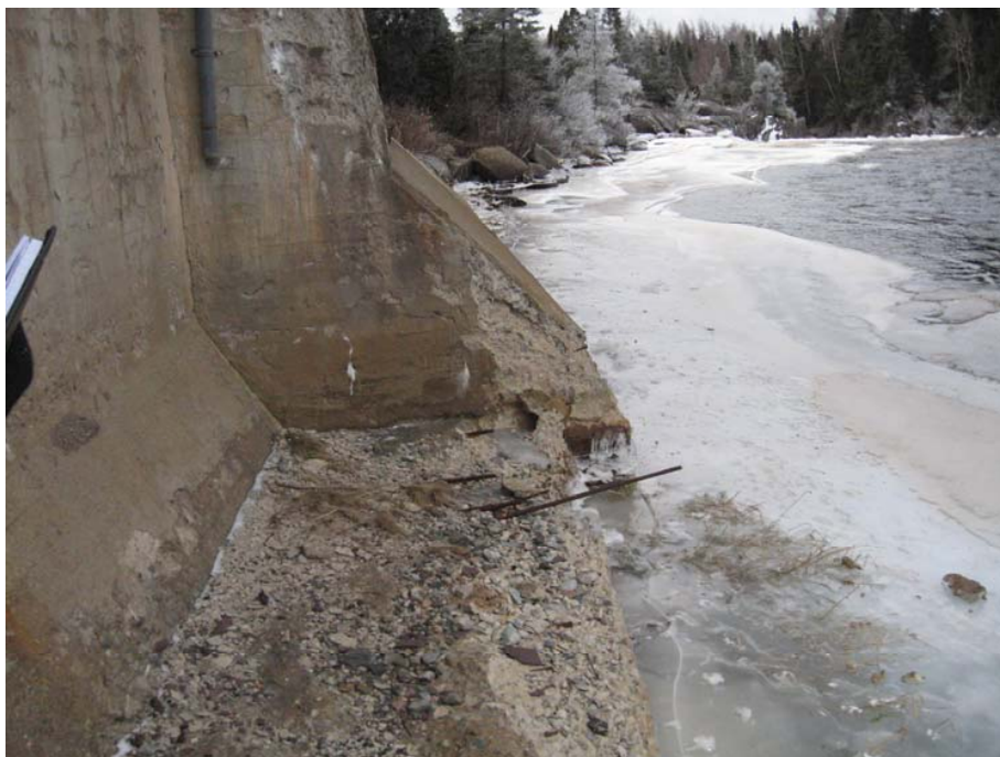
Photo 69 - Very severe erosion of South-West Retaining Wall footing.
