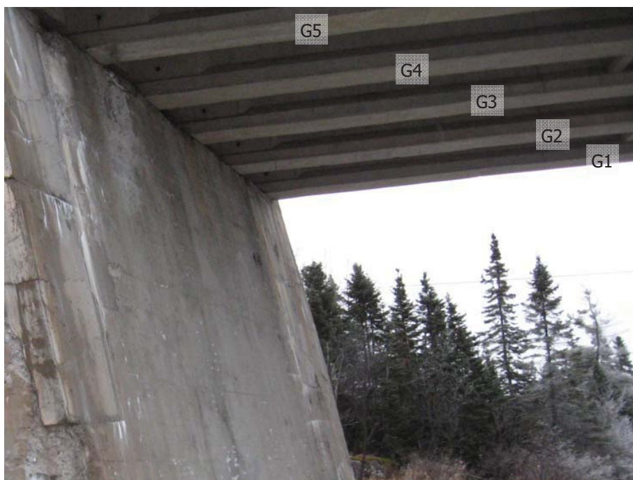
Photo 56 - Girders bearing on West Abutment.
