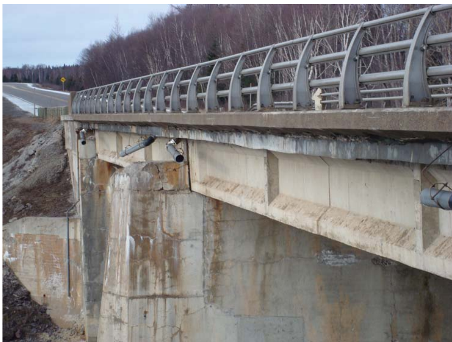
Photo 36 - Deck drain pipes on North (downstream) side of structure (similar on South side).
