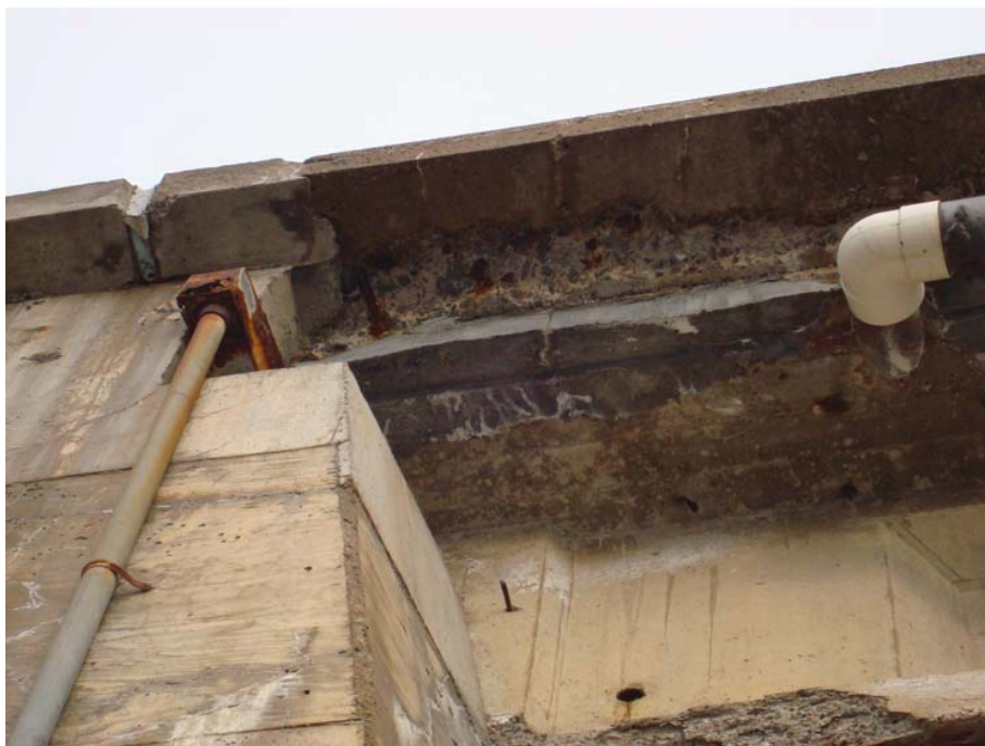
Photo 17 - Deck soffit outside girders near abutment.
