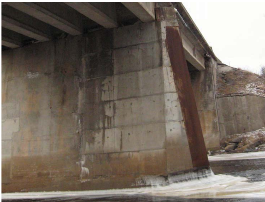
Photo 73 - Steel face plate on upstream end of pier. Rusted.
