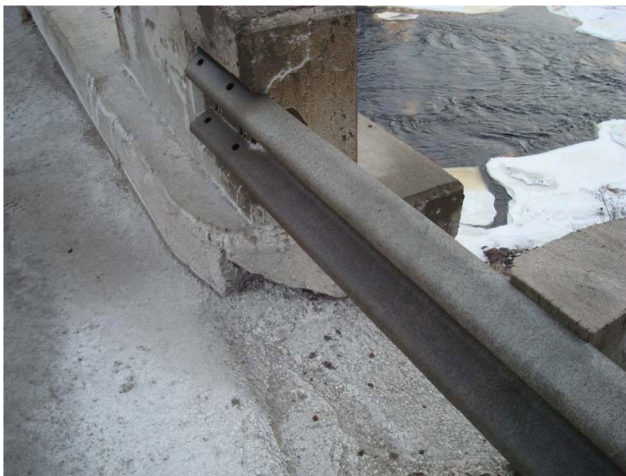
Photo 4 - Connection of galvanized steel approach guardrail to bridge structure.
