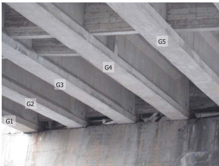
Photo 52 - Girders bearing on west side of Pier.
