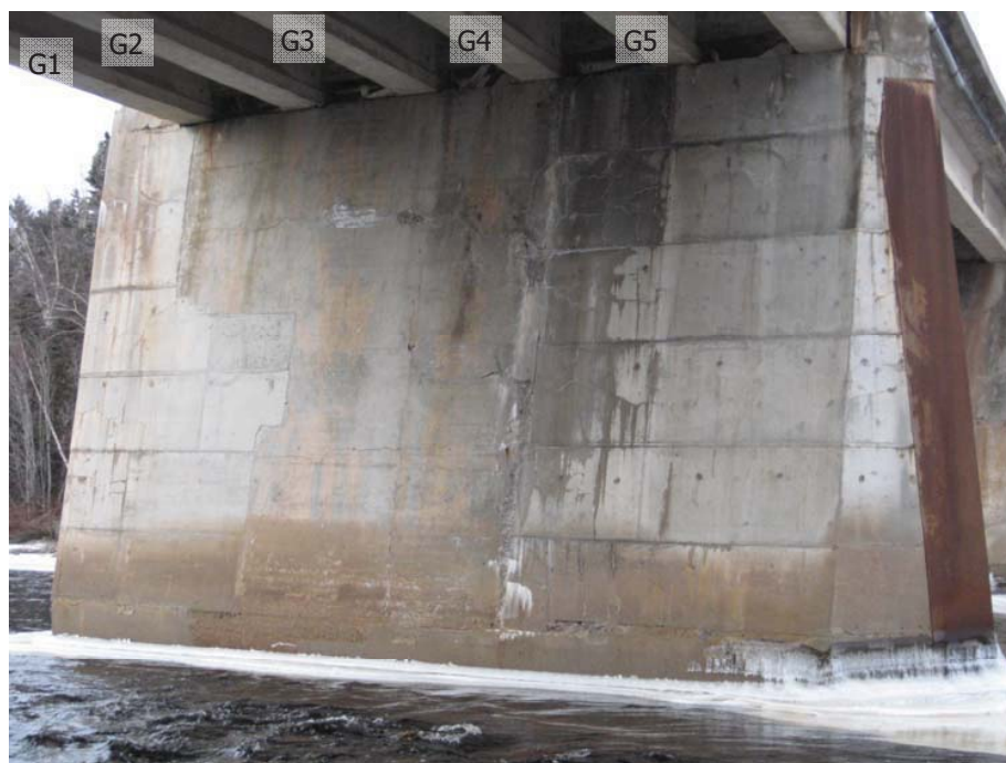
Photo 72 - West face of Pier showing vertical crack with efflorescence staining originating between girders G4 and G5.
