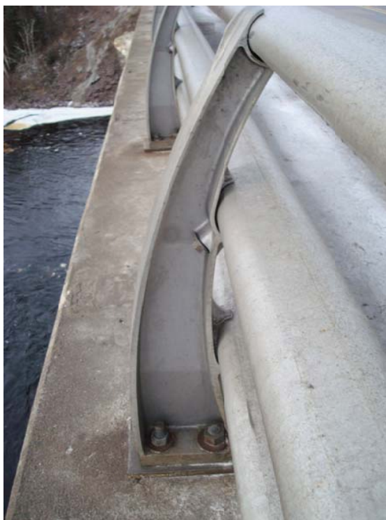
Photo 29 - Typical aluminum bridge rail post.
