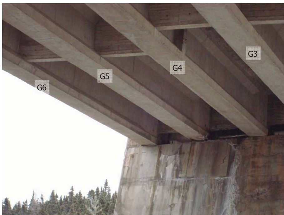
Photo 46 - Girders bearing on East side of pier.
