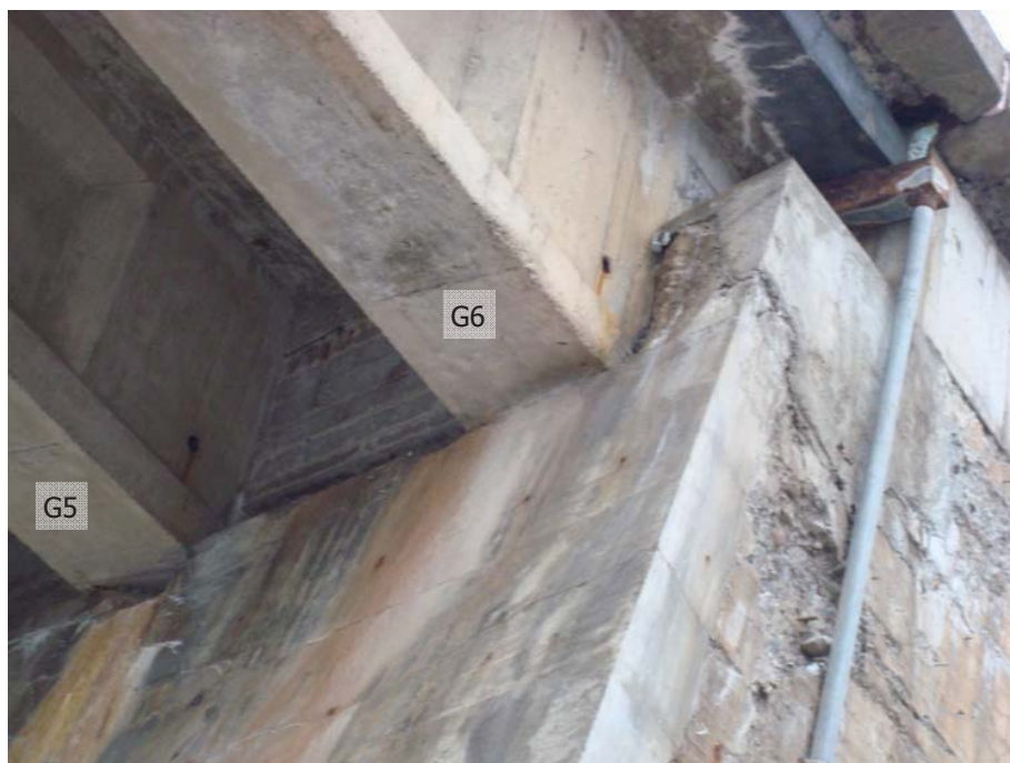
Photo 43 - Girders bearing on East abutment.
