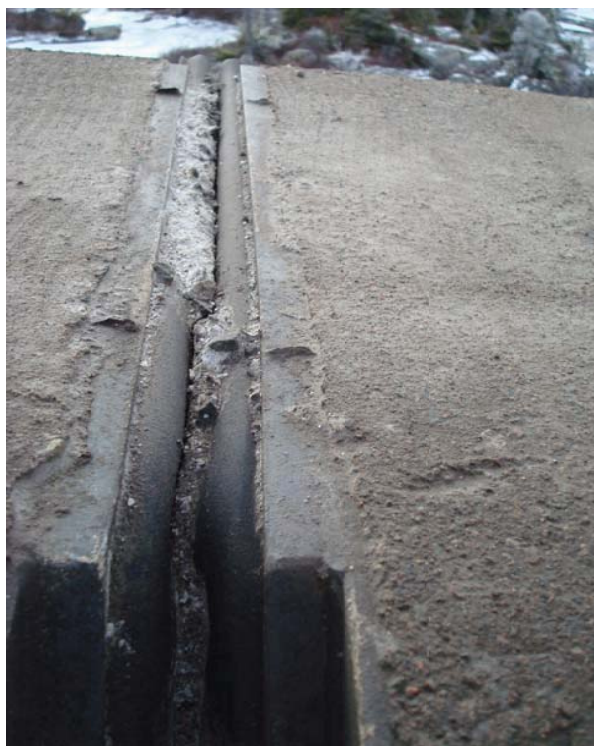
Photo 21 - Centre deck joint at curb.
