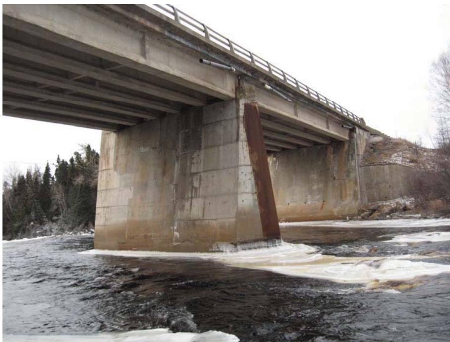
Photo 10 - Flowing water and ice build-up on upstream (South) side of pier and abutments.
