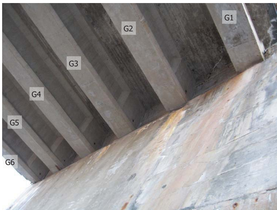
Photo 42 - Girders bearing on East abutment.
