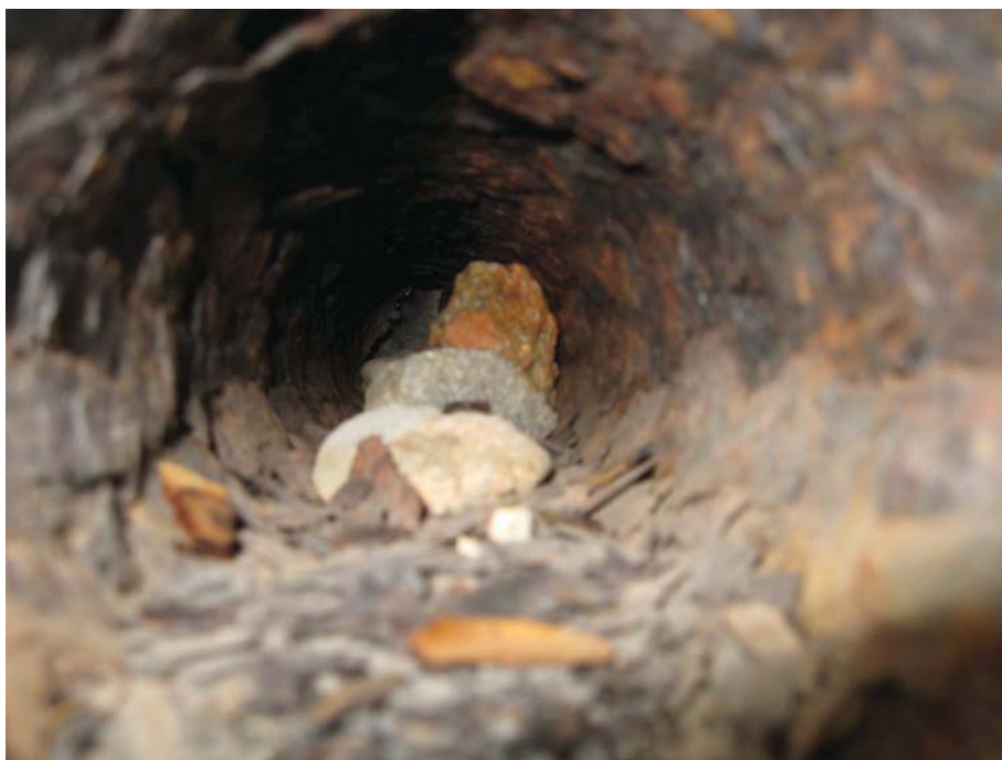
Photo 70 - View inside typical retaining wall and abutment drainage port.
