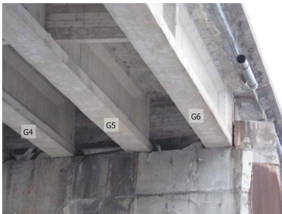
Photo 54 - Girders bearing on west side of Pier.
