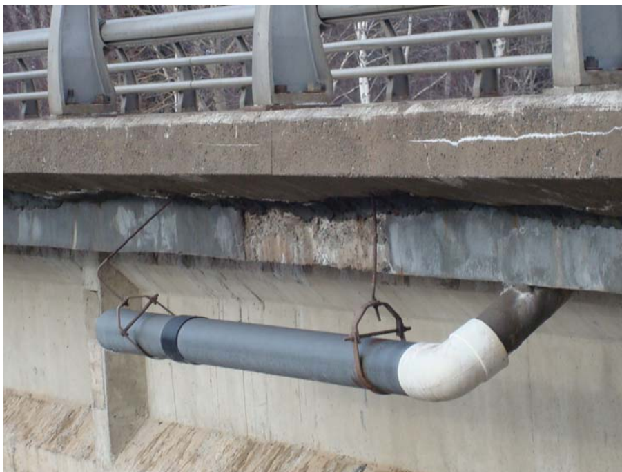
Photo 37 - Typical deck drain pipe.
