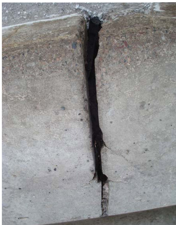
Photo 19 - East expansion joint at curb.
