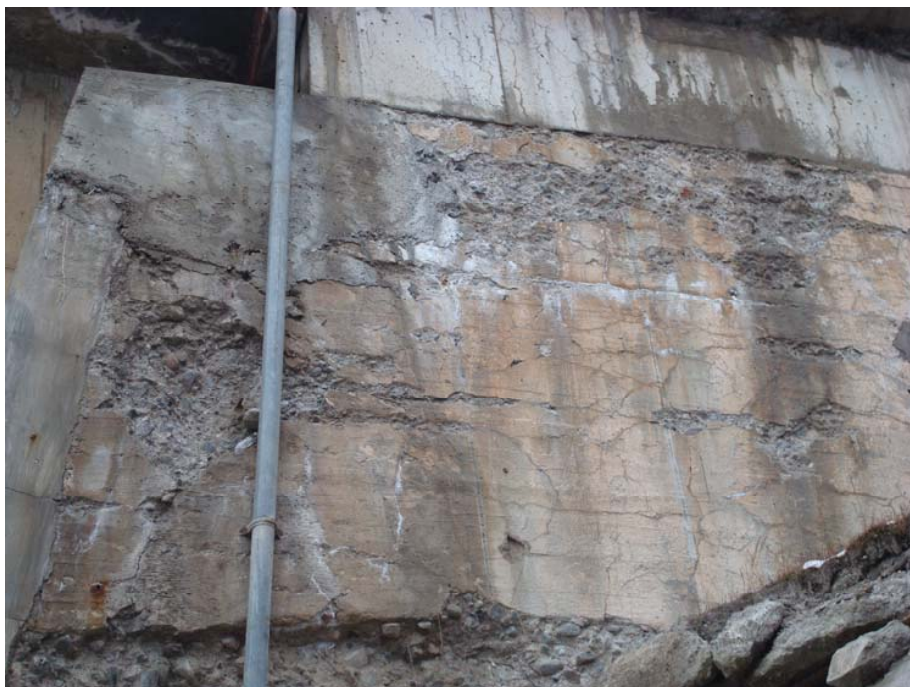
Photo 61 - Upper section of South-East Wing Wall showing significant pattern cracking and concrete spalling.
