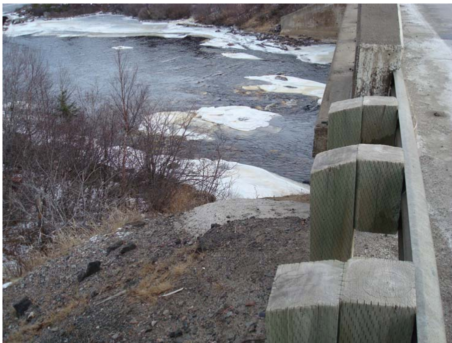
Photo 5 - Timber members supporting approach guardrail.
