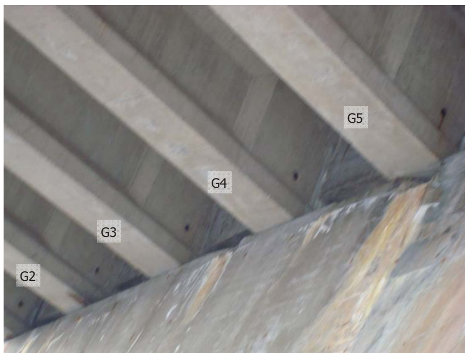
Photo 44 - Girders bearing on East abutment.
