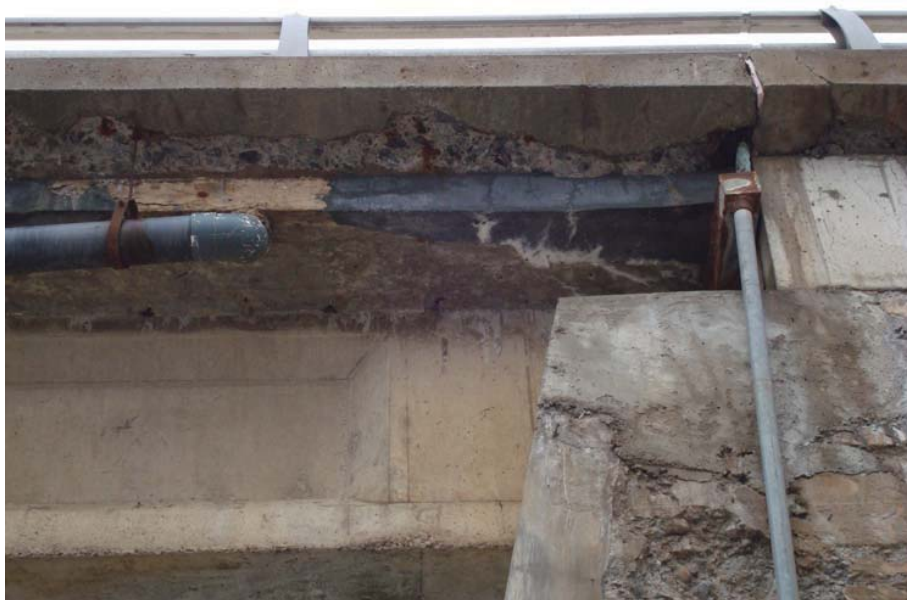
Photo 34 - Deteriorated concrete at curb soffit near abutment.
