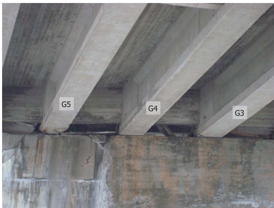
Photo 48 - Girders bearing on East side of Pier.
