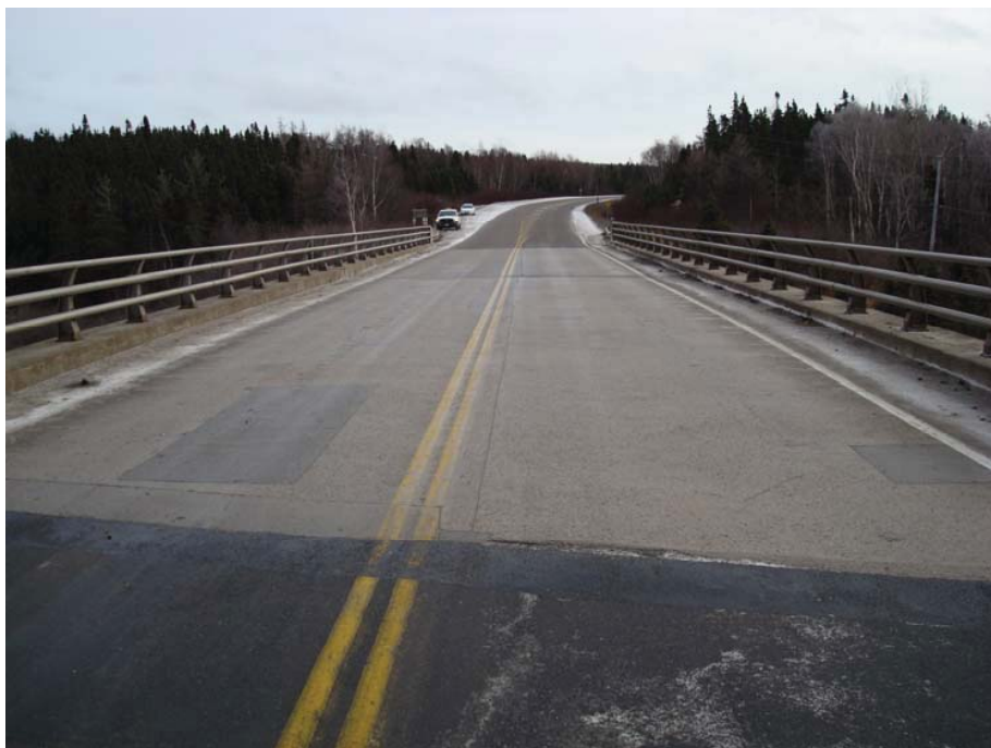
Photo 13 - Exposed concrete deck as wearing surface.
