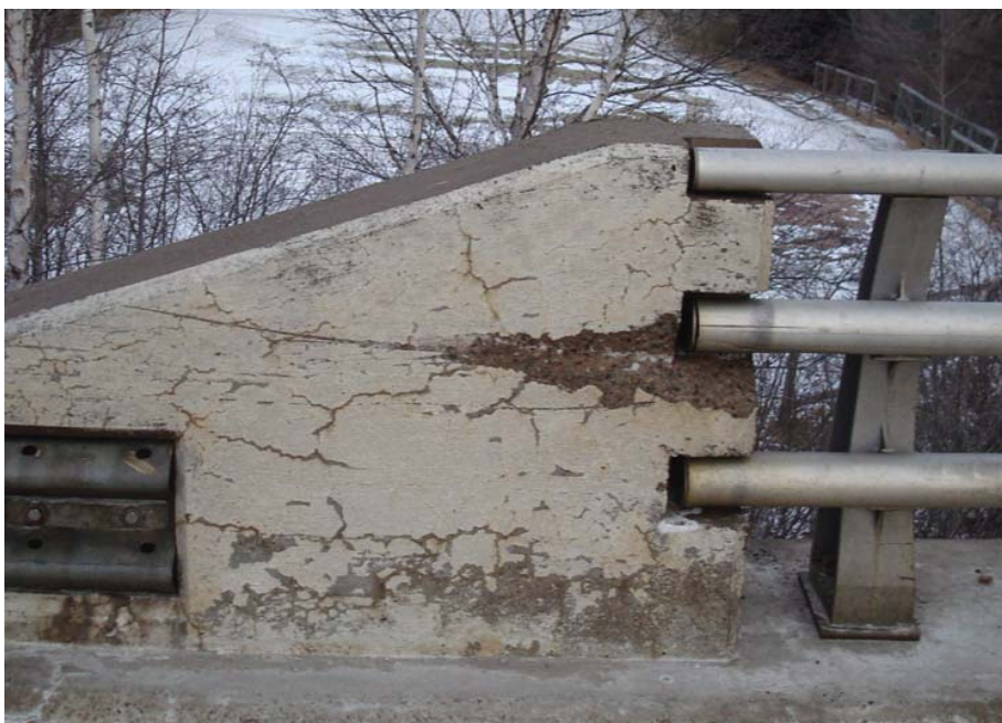
Photo 32 - Scratched bridge rail due to possible impact at south-east endwall.
