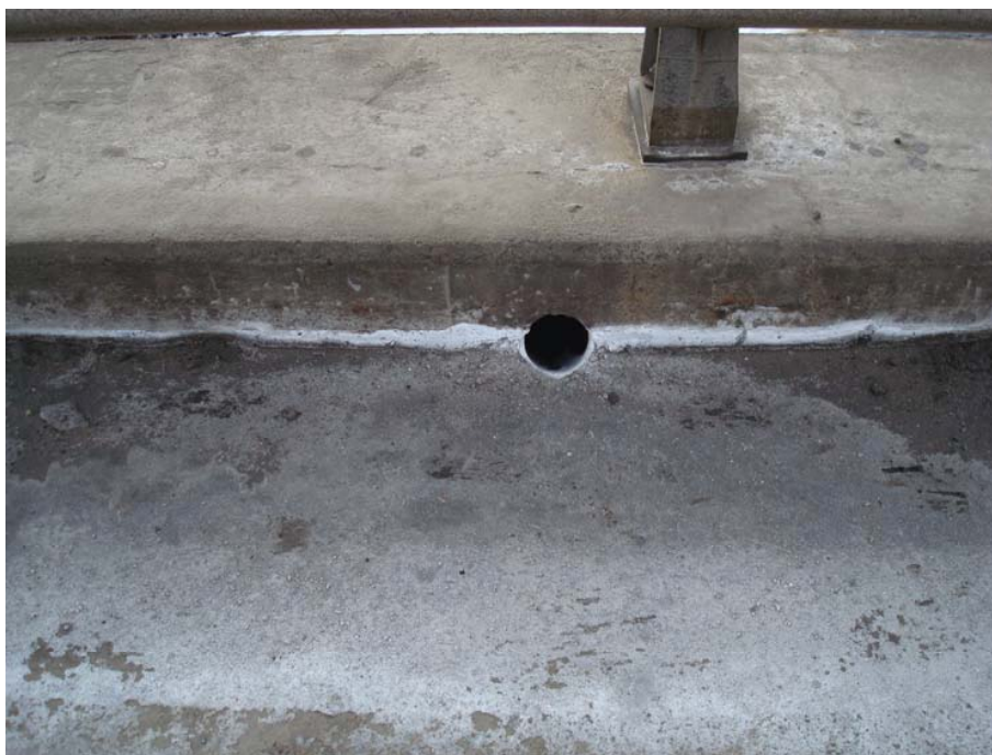
Photo 38 - Typical deck drain from above.
