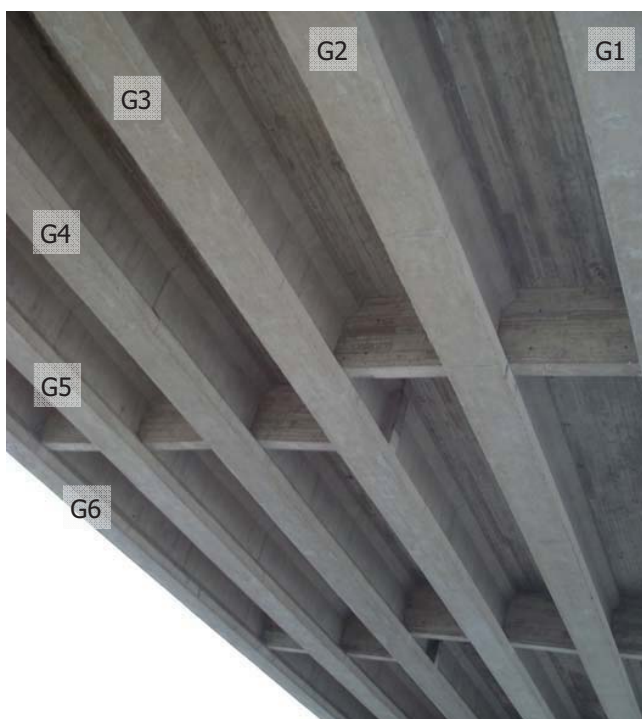
Photo 41 - Concrete girders from below (East span).
