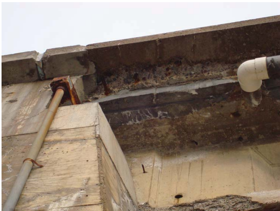
Photo 35 - Deteriorated concrete at curb soffit near abutment.
