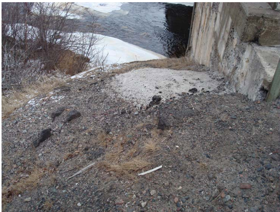
Photo 9 - Embankment behind abutment retaining walls. Lean concrete applied to reduce localized erosion.
