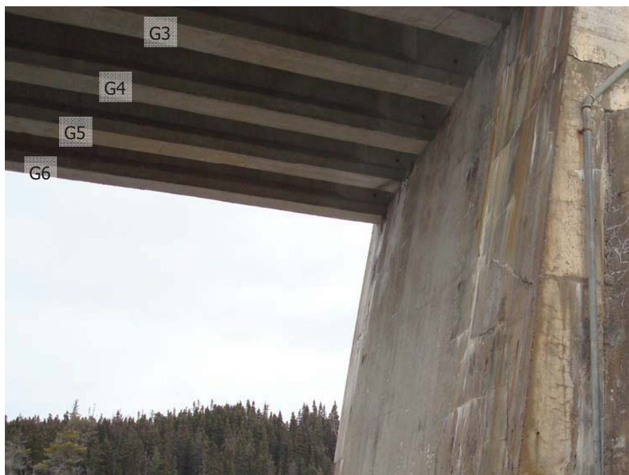
Photo 57 - Girders bearing on West Abutment.
