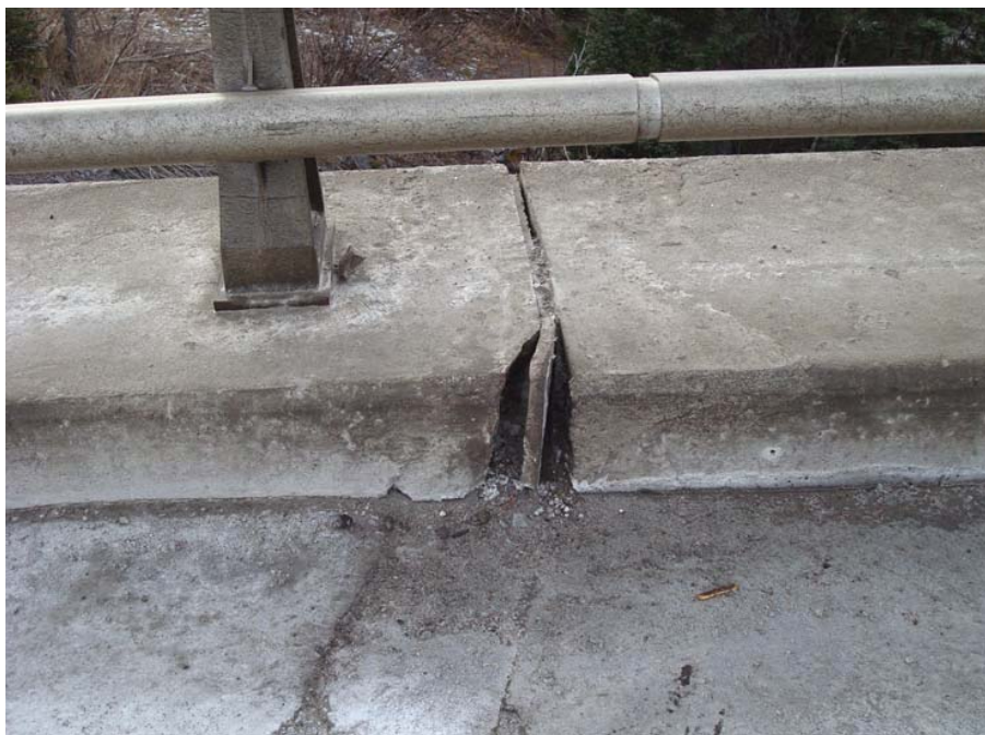
Photo 25 - Curb at west expansion joint.
