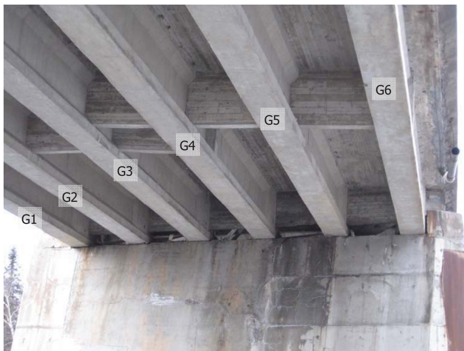
Photo 55 - Girders bearing on west face of Pier.
