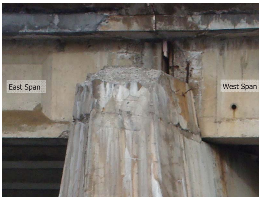
Photo 53 - Spalling and delamination on side face of Girder G1 (West Span) over pier.
