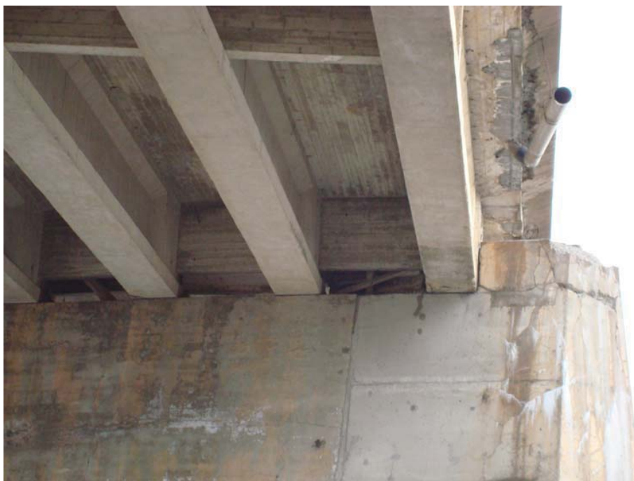
Photo 76 - Deteriorated concrete at top of pier end with delamination, cracking, efflorescence and rust stains.
