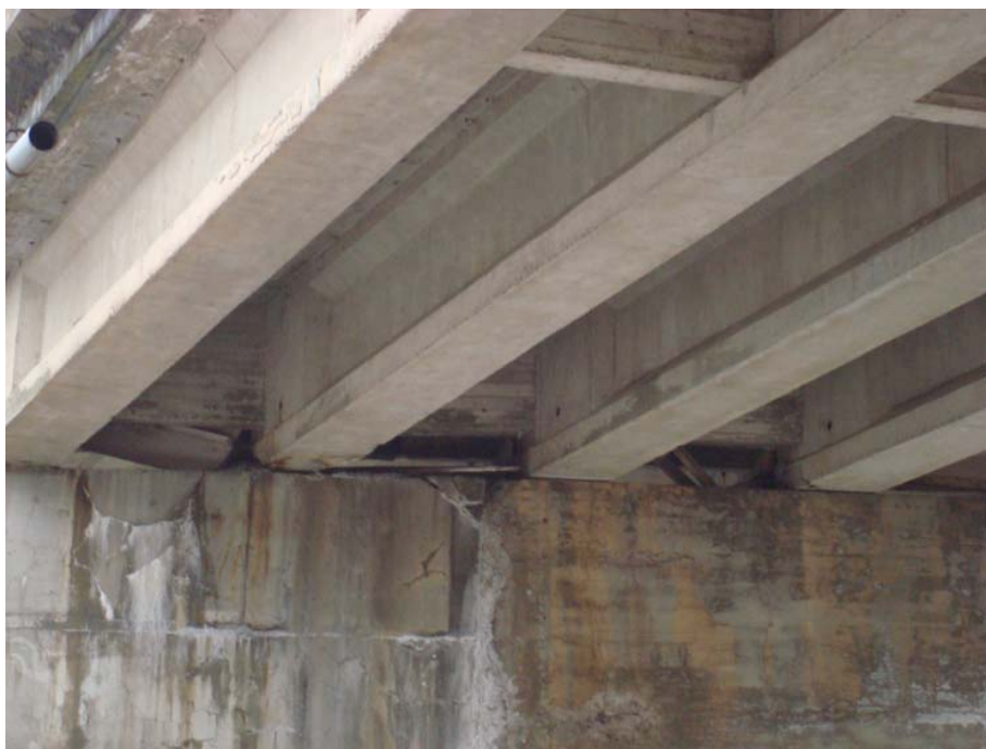
Photo 22 - Debris and signs of significant water infiltration through centre joint above.
