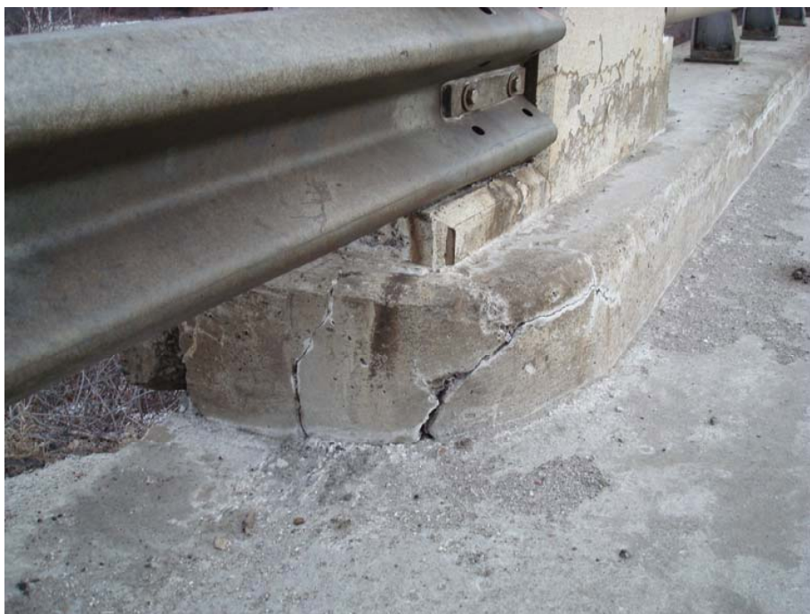
Photo 28- Cracked and damaged concrete at rounded curb ends under end walls.
