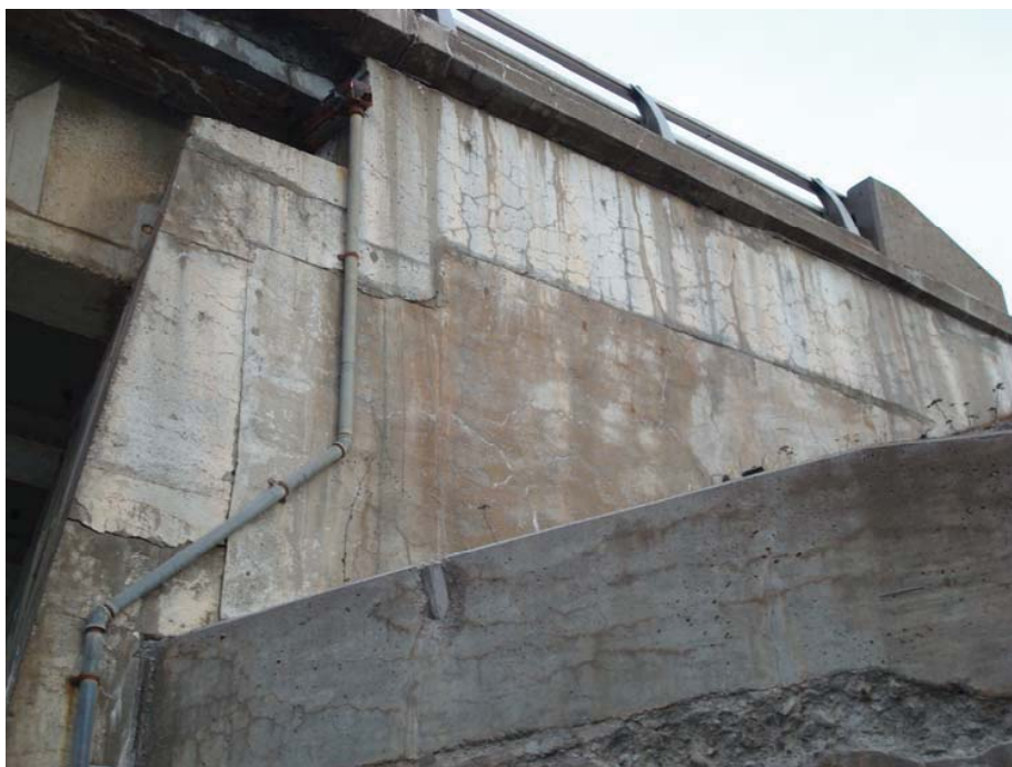
Photo 40 - Abandoned drainage pipe leader (typical at both sides of each abutment).
