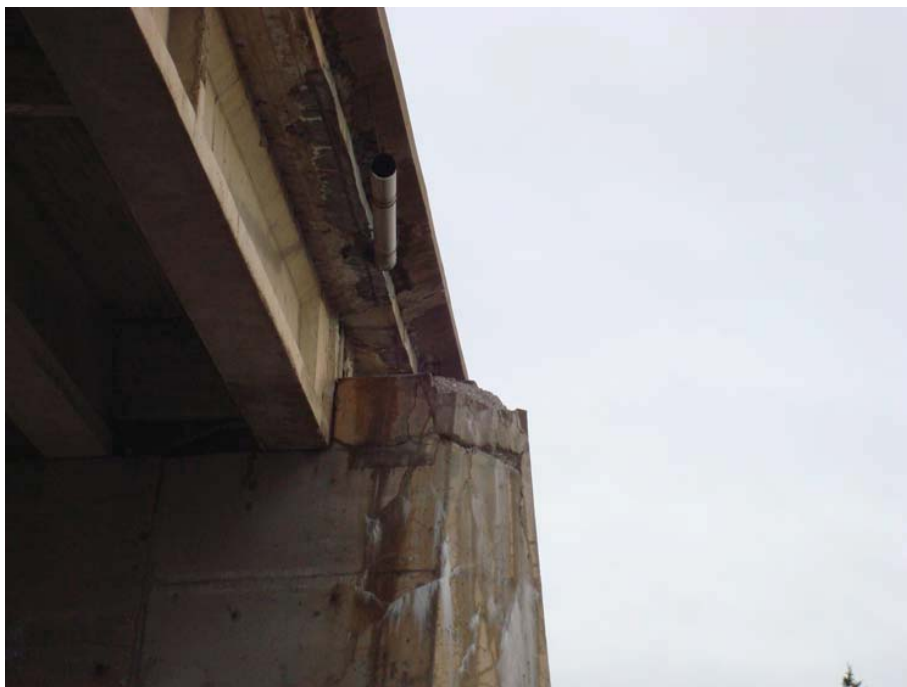
Photo 75 - Deteriorated concrete at top of pier end with delamination, cracking, efflorescence and rust stains.
