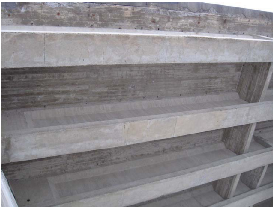
Photo 14 - Deck soffit between girders (typ.).
