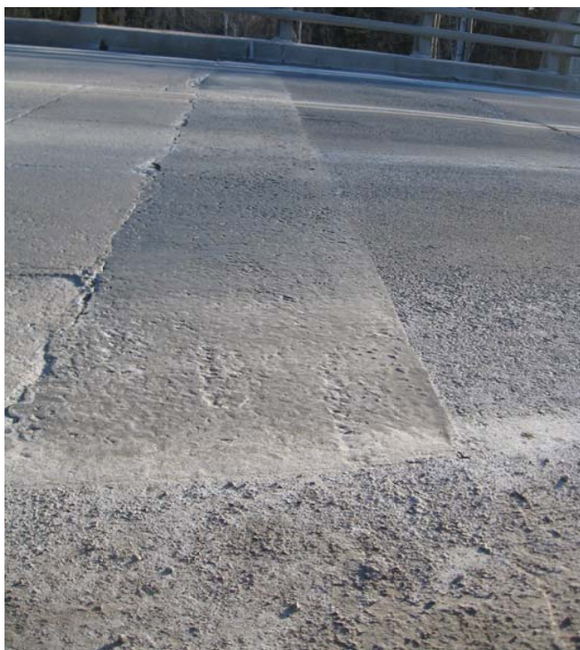
Photo 18 - East expansion joint paved over with flexible material (asphalt plug).
