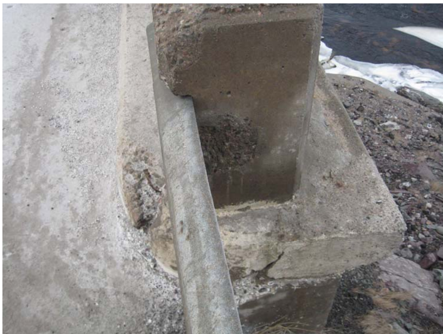
Photo 27 - Damaged concrete at end wall.
