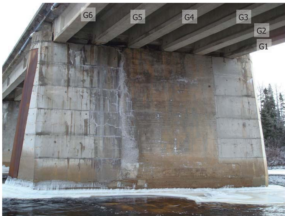
Photo 71 - East face of Pier showing vertical crack with efflorescence staining originating between girders G4 and G5.
