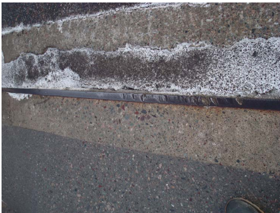
Photo 24 - Missing steel edge (one side) and asphalt patching at West expansion joint.
