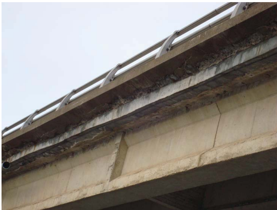
Photo 33 - Deteriorated concrete at curb soffit.
