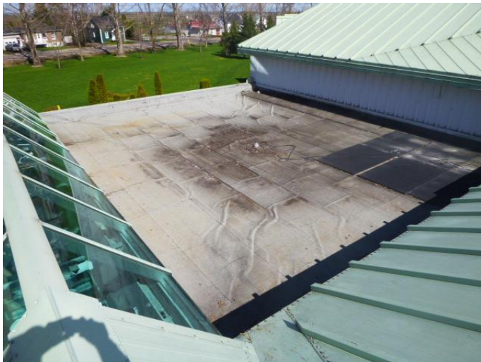
Flat roof front view – East
