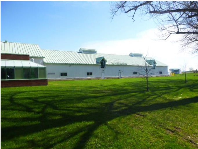
Front view – West
