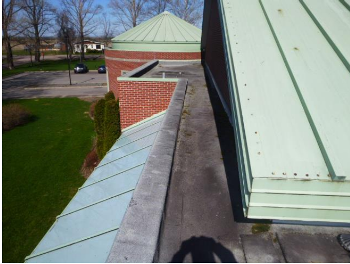
Flat roof front view – West
