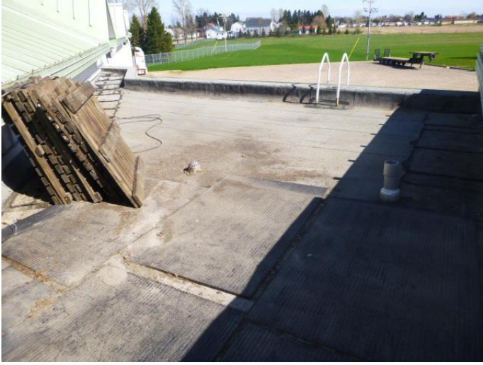
Flat roof rear view – East
