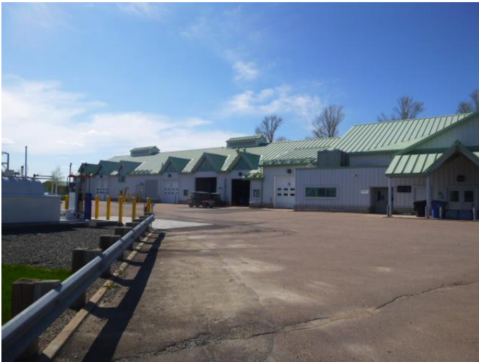
Rear view – West
