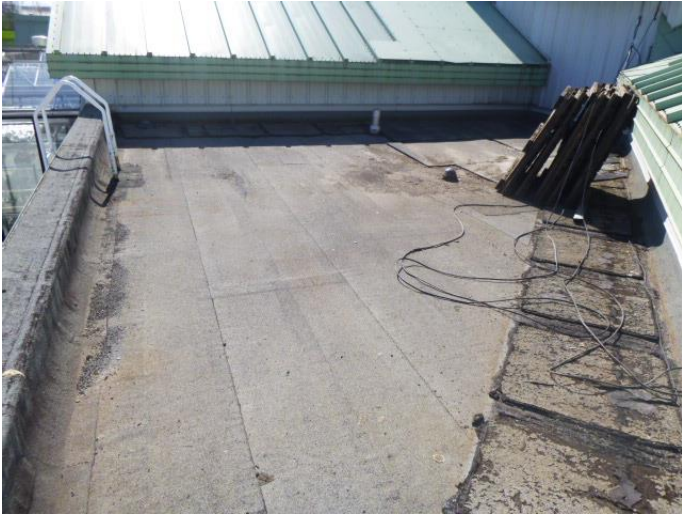
Flat roof rear view – East
