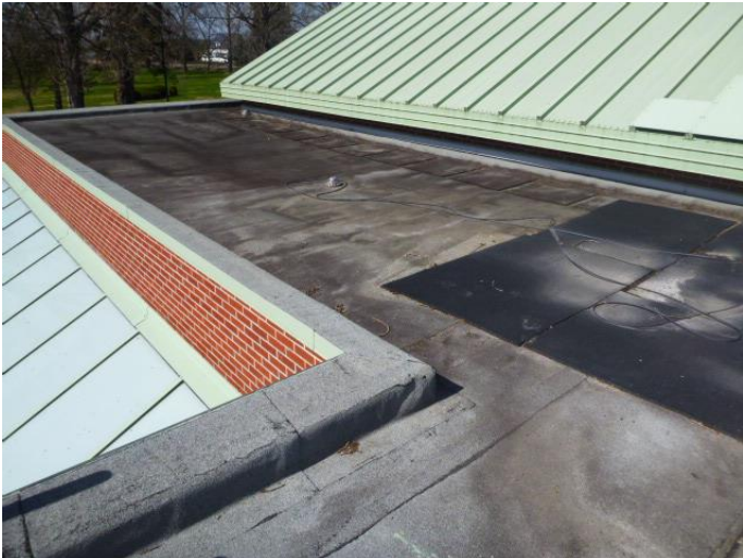
Flat roof front view – West
