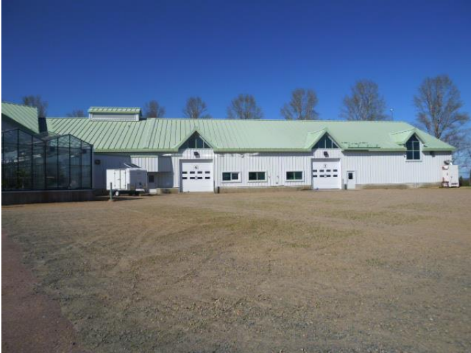
Rear view – East
