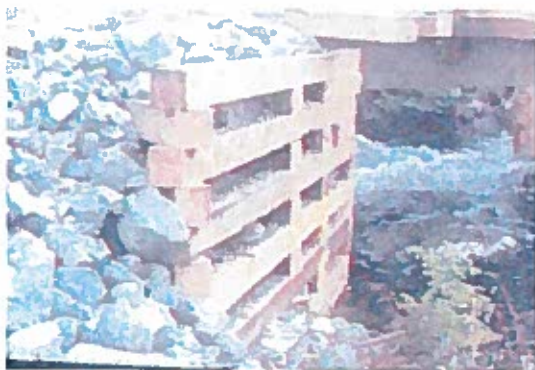
Figure 1: Infill material for timber cribs should be blocky, angular and free of fines or sediment.
