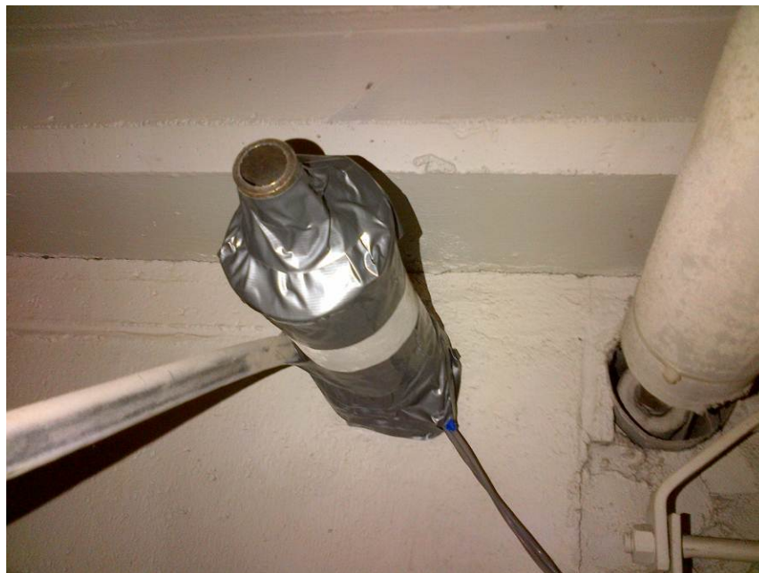
Approximately one foot section of damaged asbestos-containing straight pipe insulation – Corridor outside the fan room on the 2 nd floor.
