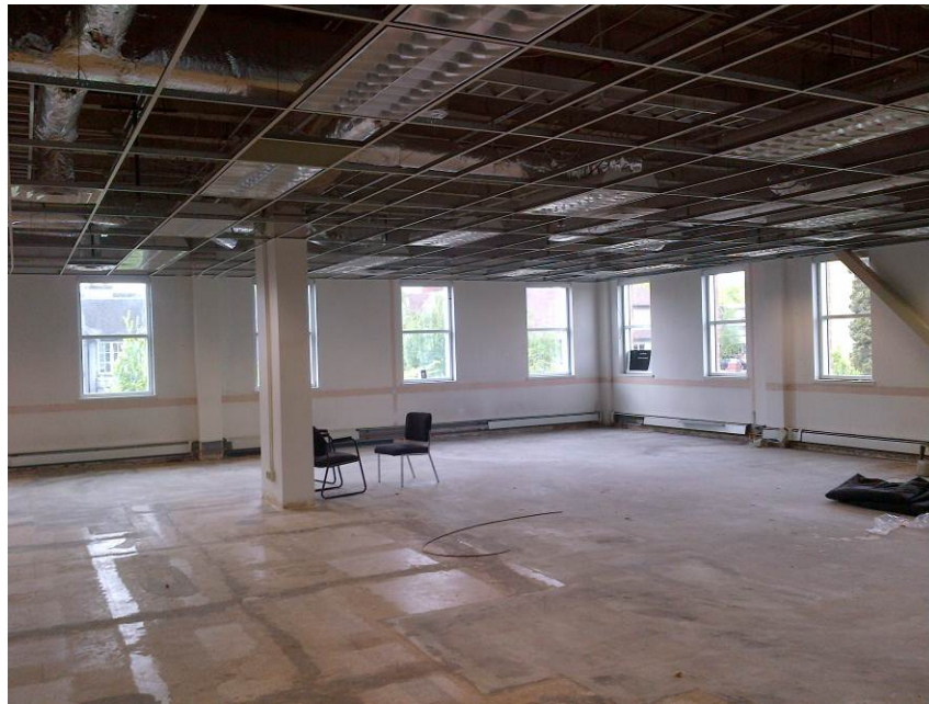
Asbestos-containing wall plaster on exterior walls – West end of the 3 rd floor.
