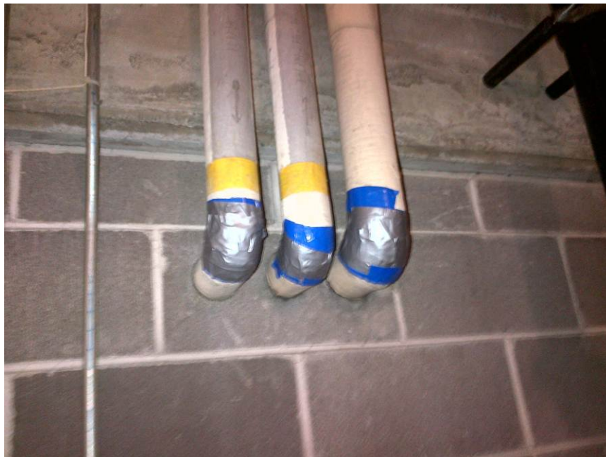
Damaged asbestos-containing mechanical pipe insulation on three fittings – Parkade
