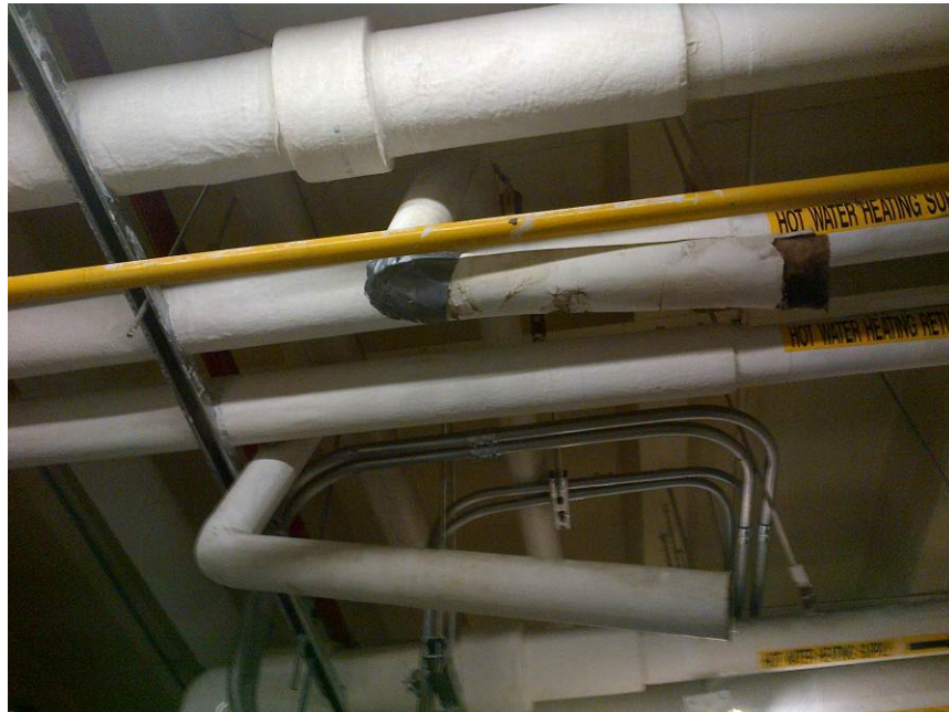
Damaged asbestos-containing mechanical pipe insulation on approximately four fittings on an abandoned pipe – Boiler room
