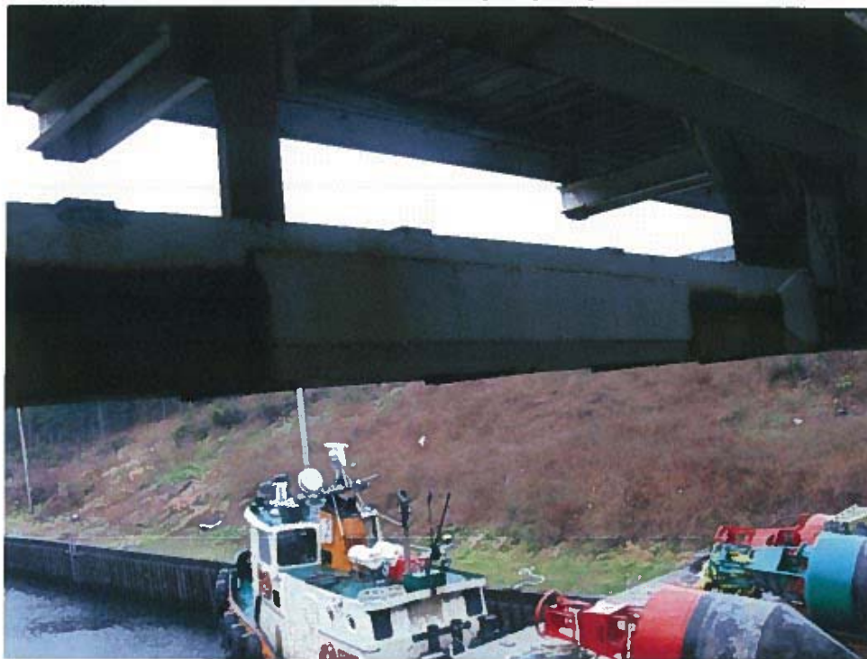
Photograph 26 – Welded reinforcement along south truss (between panel points 4E and 5E).
