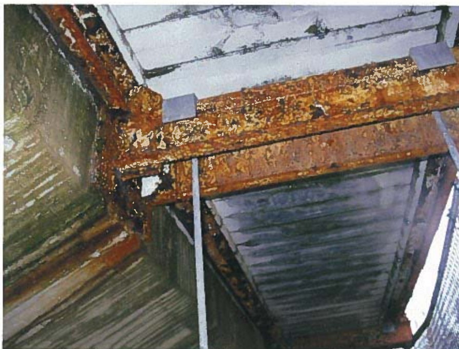
Photograph 37 – Typical condition of structural steel at sidewalk overhang at east approach. Note: Medium to severe corrosion
