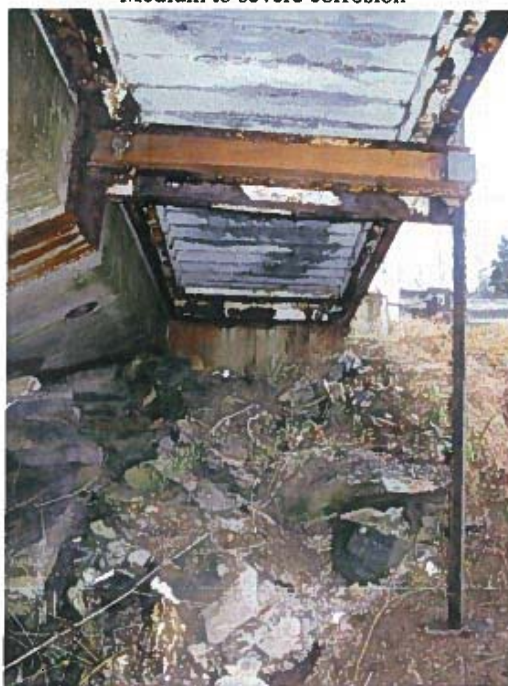
Photograph 38 – Welded reinforcement to existing transverse steel member at the sidewalk near the east abutment.
