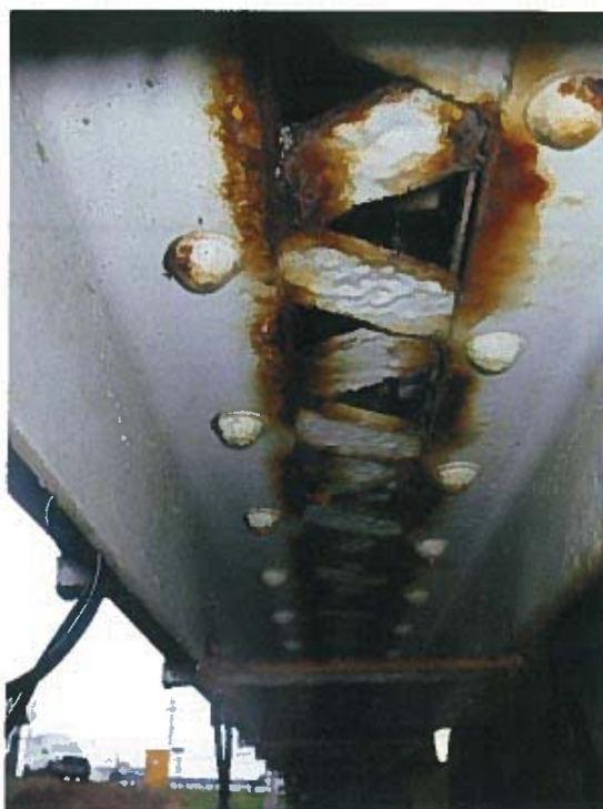
Photograph 22 – Condition of lacing bars along south truss bottom chord between panel points 3E and 5E.
