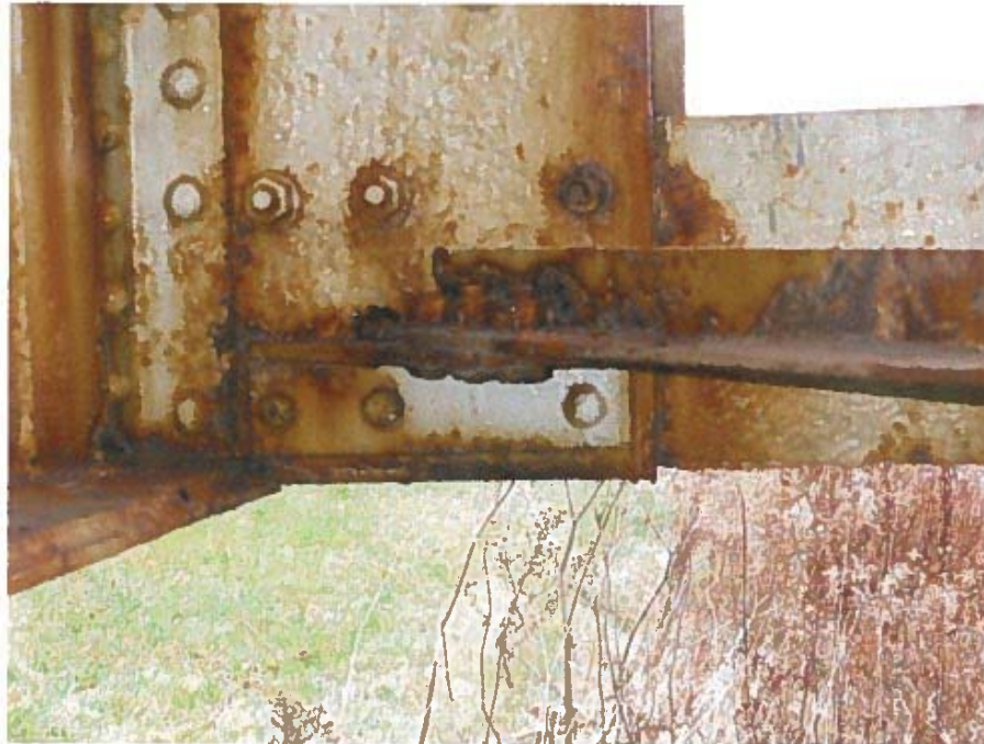
Photograph 35 – Typical condition of horizontal bracing at panel point connection. Note: Medium to severe corrosion.
