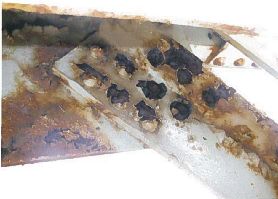
Photograph 5 – Condition of rivets at top chord (node 2W) on north truss. Note: Section loss and corrosion.
