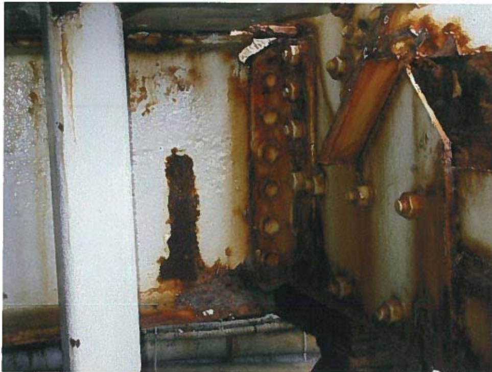
Photograph 32 – Typical condition of connection angles of the floor beam to the lower chord.
