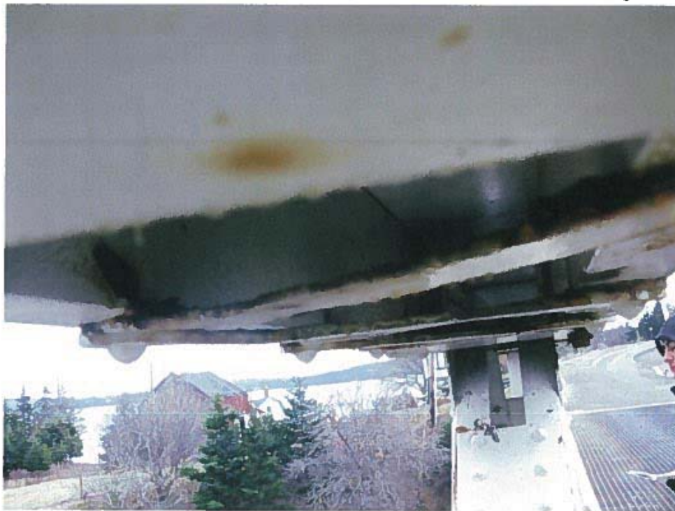
Photograph 4 – Lacing bars along top chord at north truss. Note: Section loss in lacing bars.
