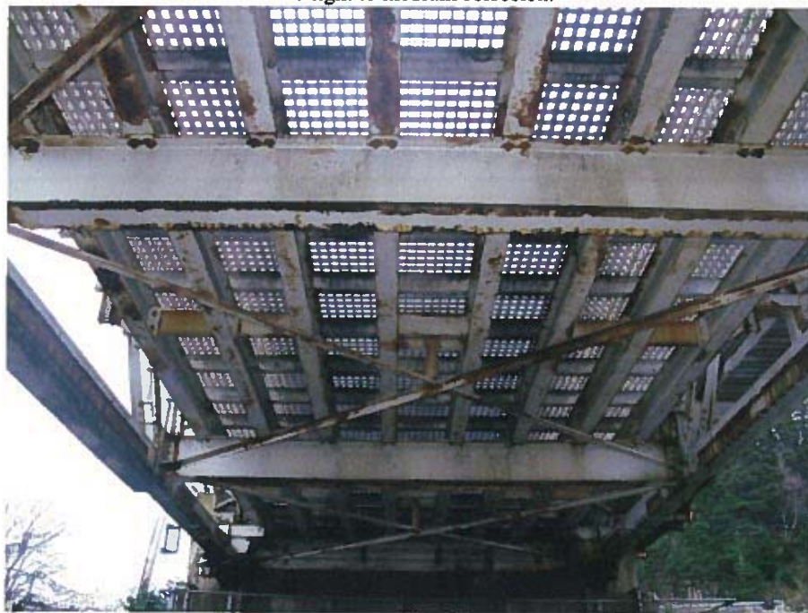
Photograph 30 – Typical condition of stringer/deck beams and grating. Note: the welded reinforcement to the bottom flange of the floor beam.
