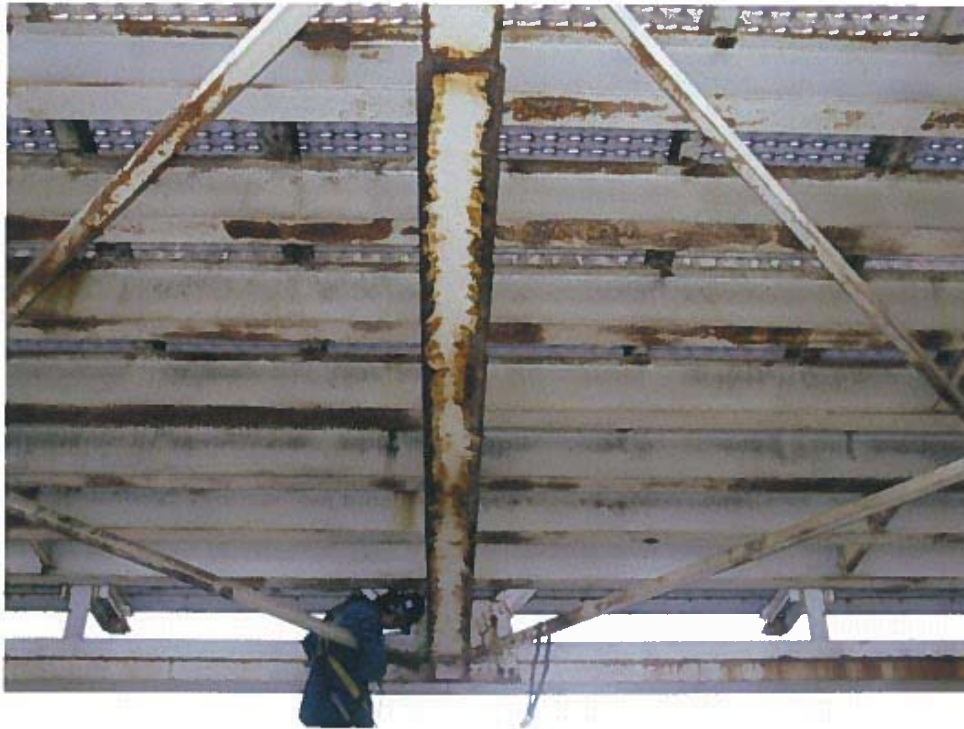
Photograph 31 – Typical condition of floor beams. Note: Welded reinforcement at the bottom flange.
