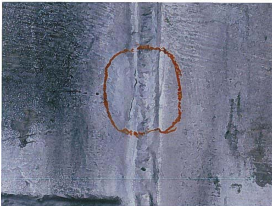
Photograph 44 – Crack in weld at welded reinforcement at panel point 5E south truss bottom chord.
