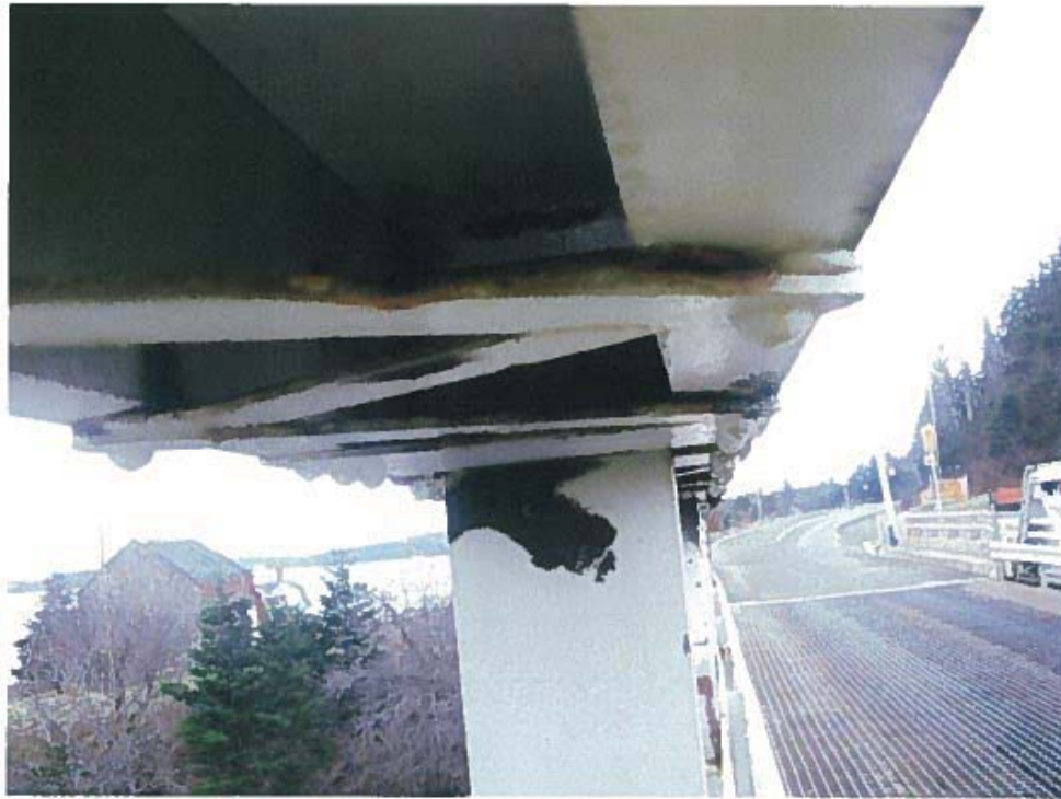
Photograph 3 – Lacing bars along top chord at north truss. Note: Section loss in lacing bars.
