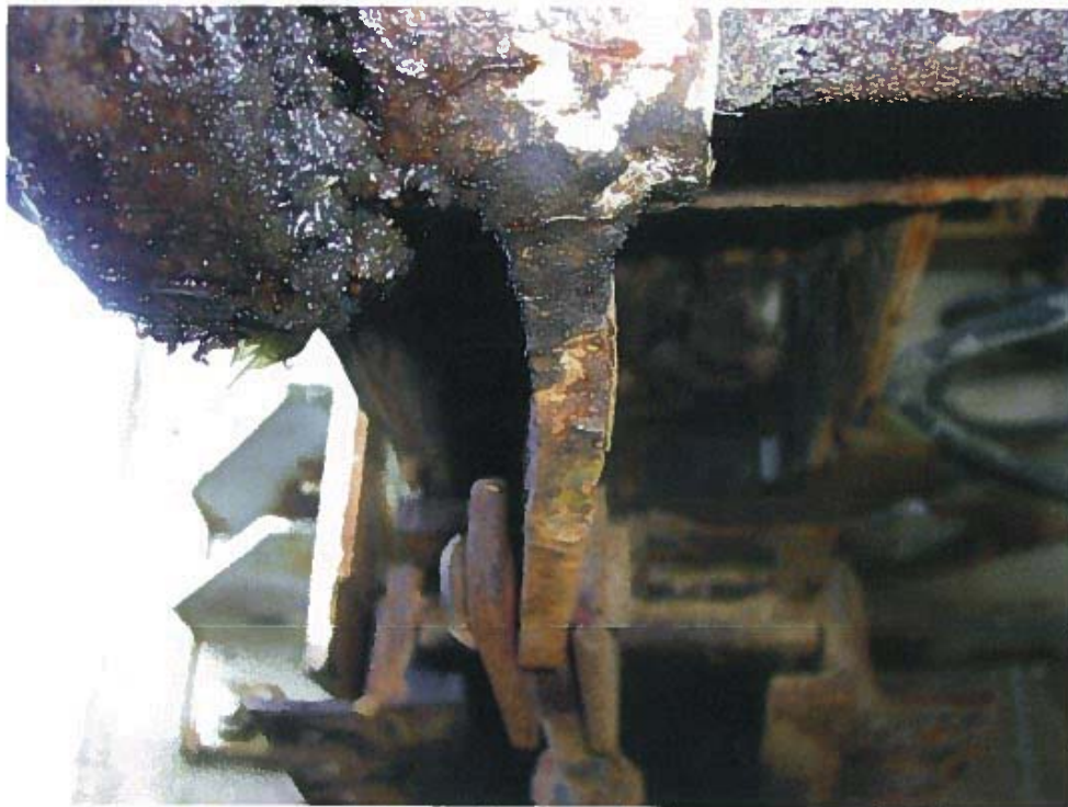
Photograph 4 – South east wedge bent crank arm
