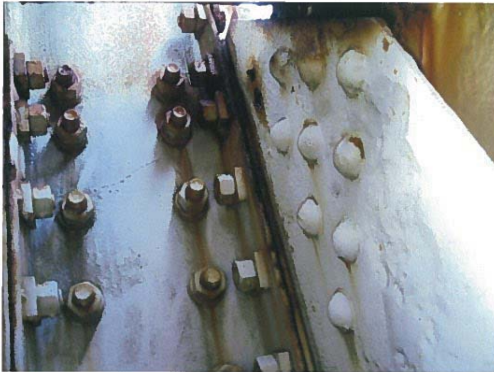
Photograph 25 – Perforation / section loss at gusset plate panel point 0 south truss bottom chord.
