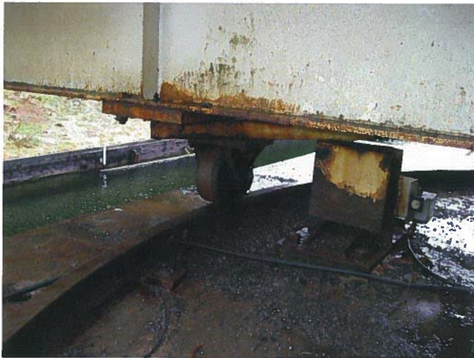
Photograph 13 – Bridge open end stop, note that rubber pad is sandwiched in between steel plates
