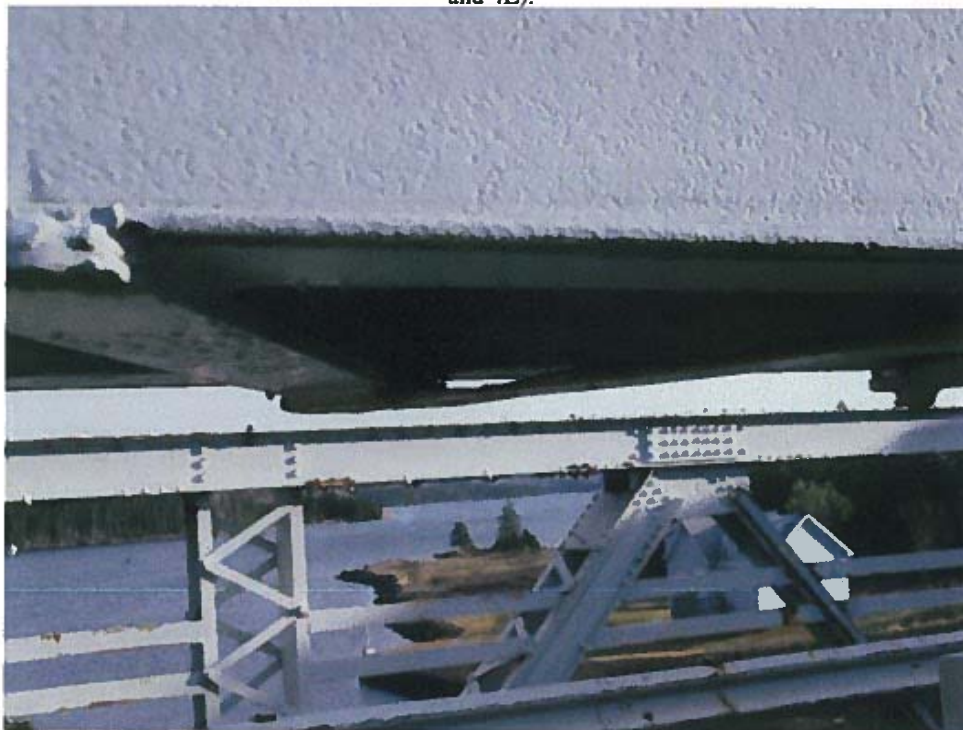
Photograph 20 – Lacing bars along top chord at south truss. Note: Section loss at lacing bars.
