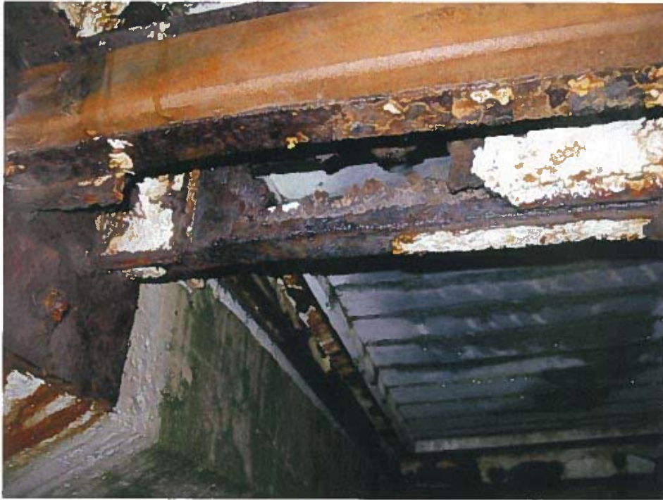
Photograph 39 – Welded reinforcement to existing transverse steel member at east app. sidewalk. Note: perforation and section loss at existing steel member
