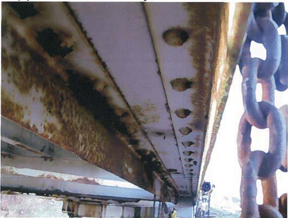
Photograph 10 - Condition of bottom chord along north truss. Note: Medium to severe corrosion.
