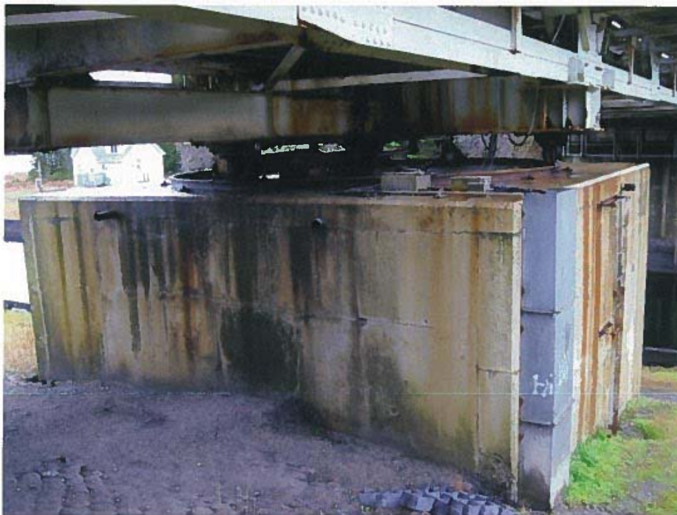
Photograph 8 – Center bearing oil drain line (pipe on the left side)
