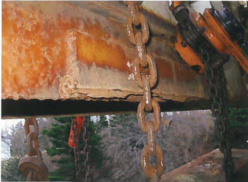
Photograph 19 – Welded reinforcements along north truss bottom chord (between panel points 3E and 4E).
