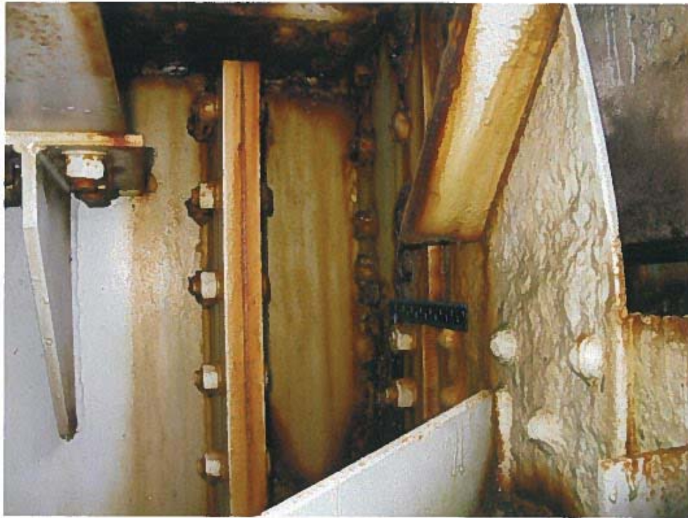
Photograph 17 – Section loss and perforation at gusset plate (panel point 0) at north truss.
