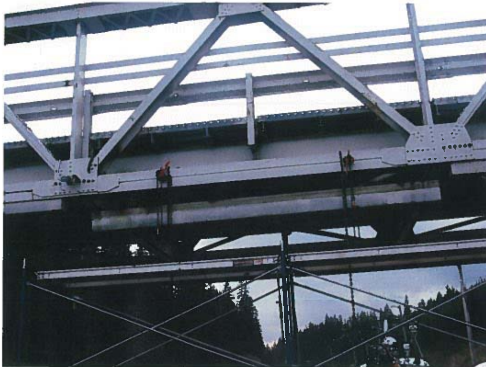
Photograph 18 – Welded reinforcement along north truss bottom chord and at panel point locations.
