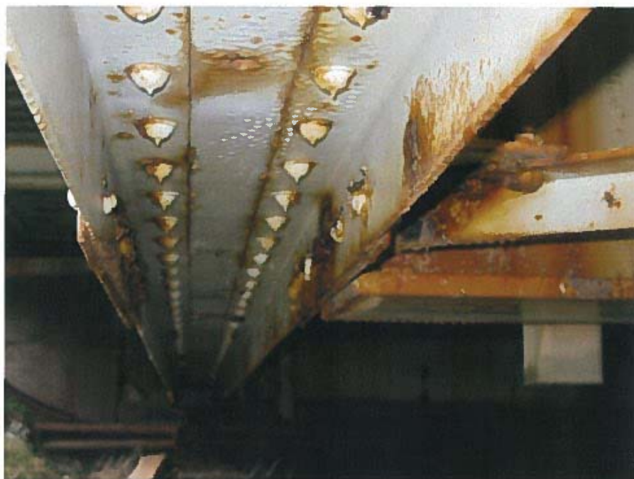
Photograph 21 – Condition of bottom chord along south truss. Note: Medium to severe corrosion.
