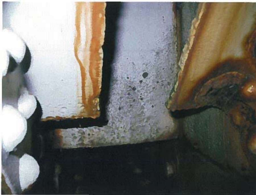
Photograph 14 – Section loss and perforation of the vertical member at panel point location along north truss bottom chord.
