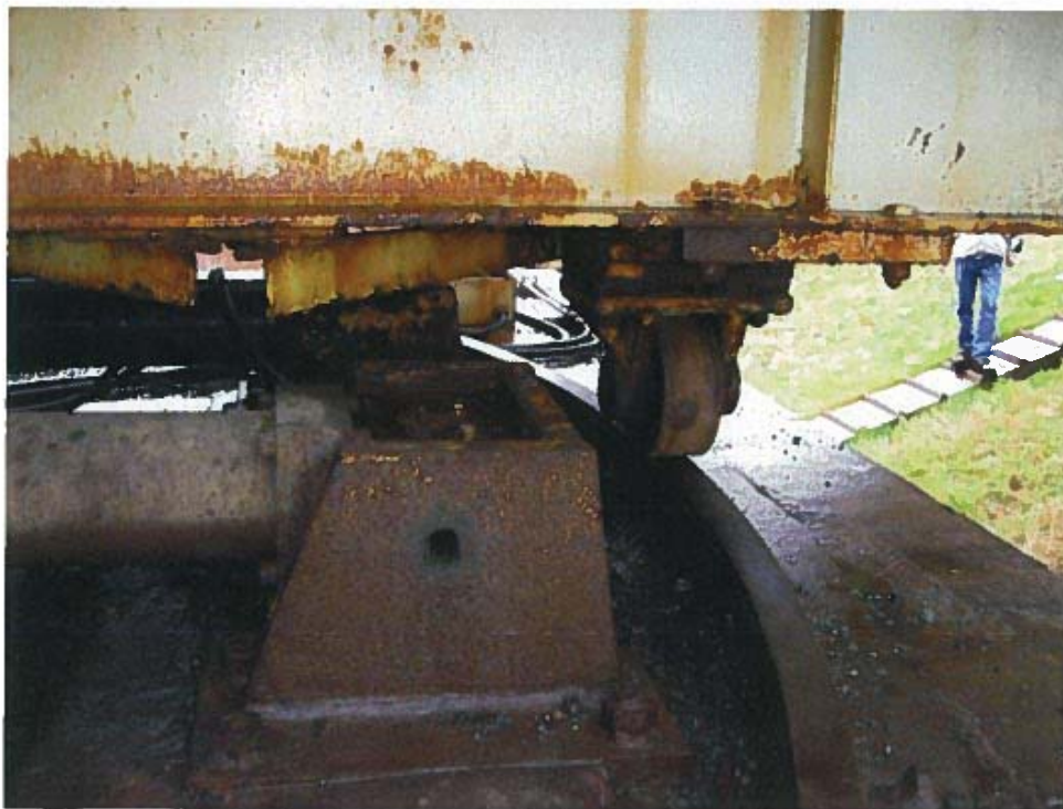
Photograph 12 – East bogey wheel, note number of shims
