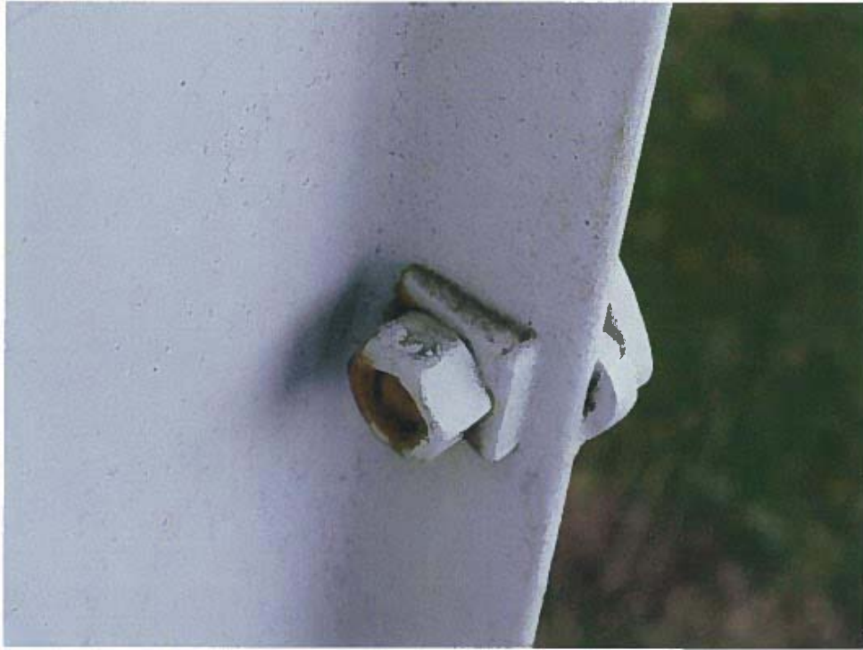
Photograph 7 – Insufficient bolt thread (typical).
