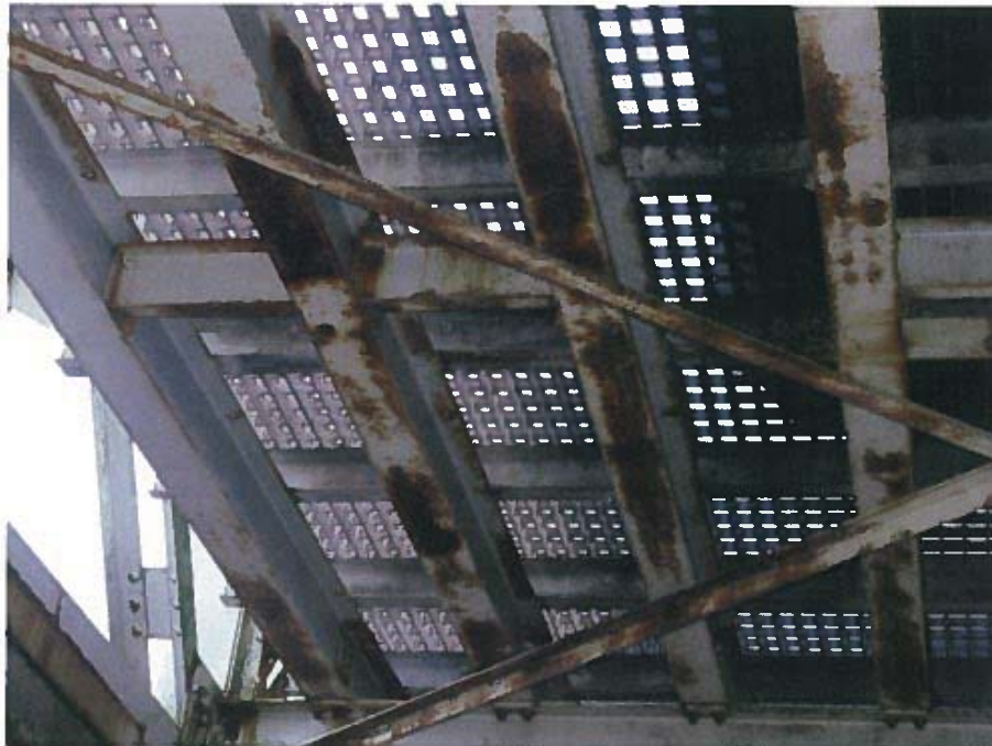
Photograph 29 – Typical condition of stringer/decking beams and grating. Note: coating break down and light to medium corrosion.
