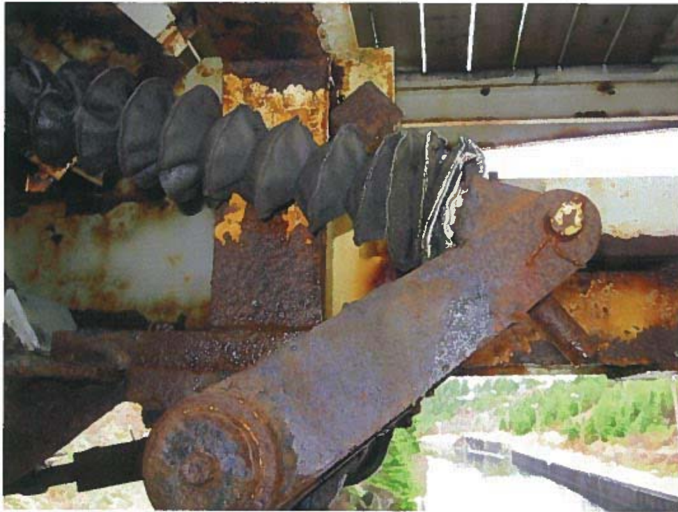
Photograph 3 – Wedge crank arm
