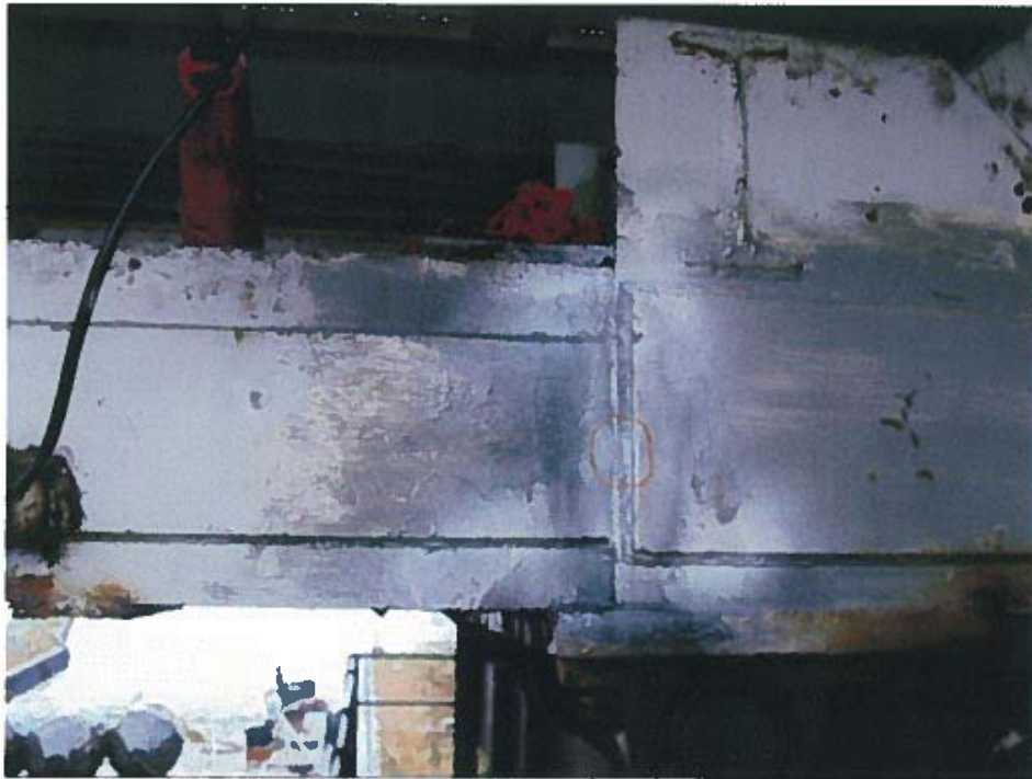
Photograph 43 – Crack in weld at welded reinforcement at panel point 5E south truss bottom chord.
