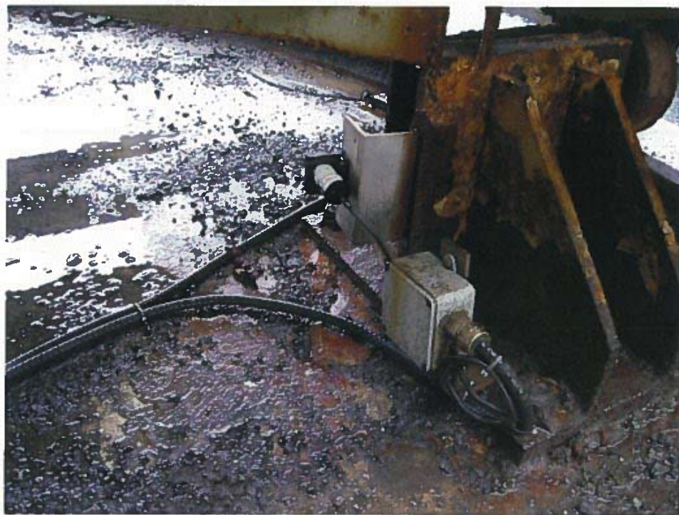
Photograph 22 – Bridge open proximity sensor
