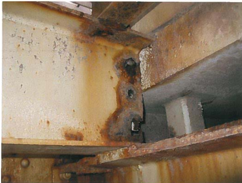
Photograph 28 – Perforation and section loss at stringer S8 between panel points 2W and 3W.
