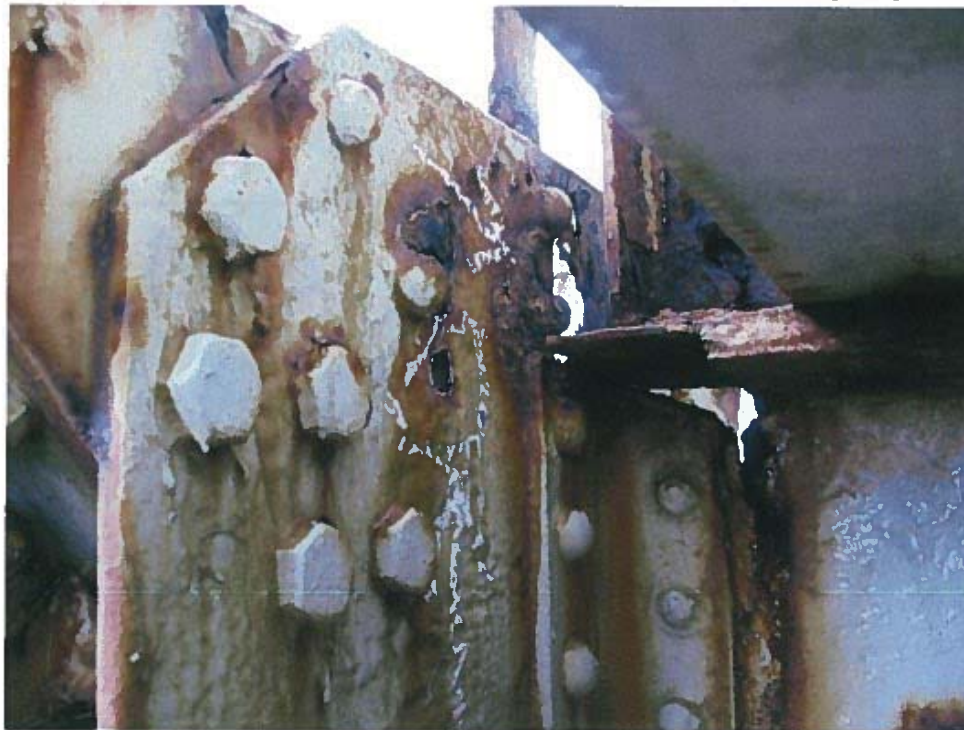
Photograph 16 - Section loss and perforation at gusset plate location at north truss panel point 2W
