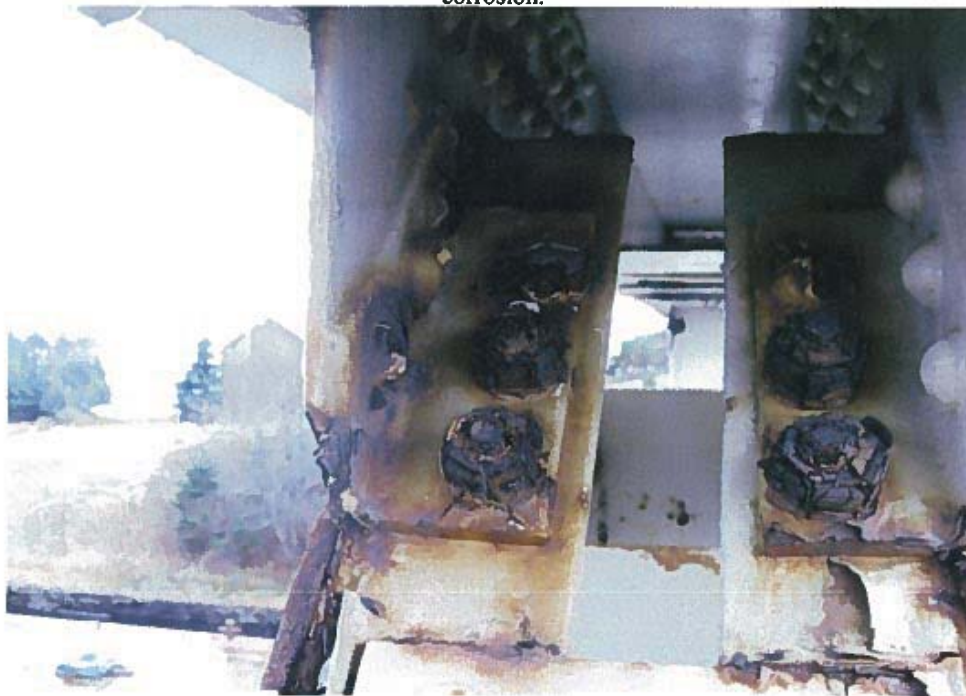
Photograph 5 – Condition of rivets at top chord (node 2W) on north truss. Note: Section loss and corrosion.
