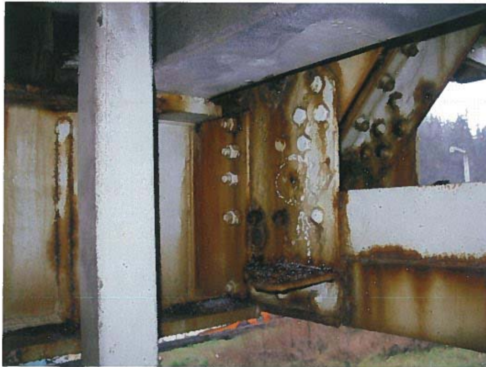
Photograph 24 – Perforation / section loss at gusset plate panel point 2W south truss bottom chord.
