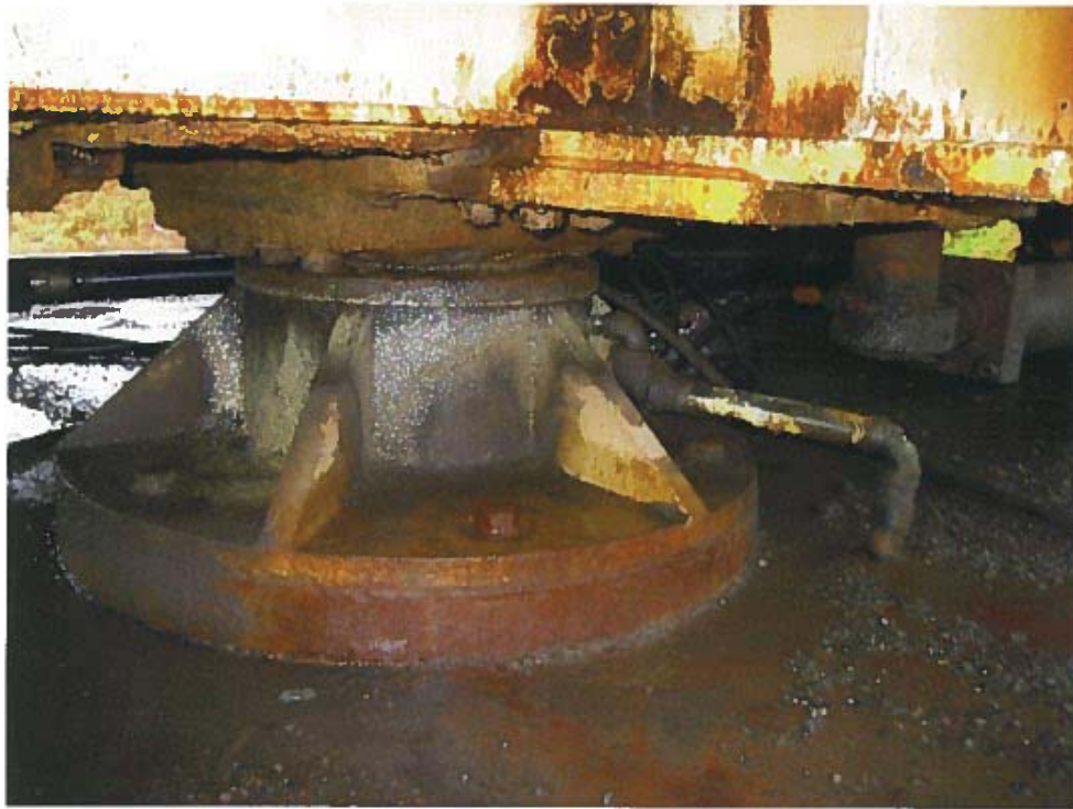
Photograph 7 – Center bearing oil drain line
