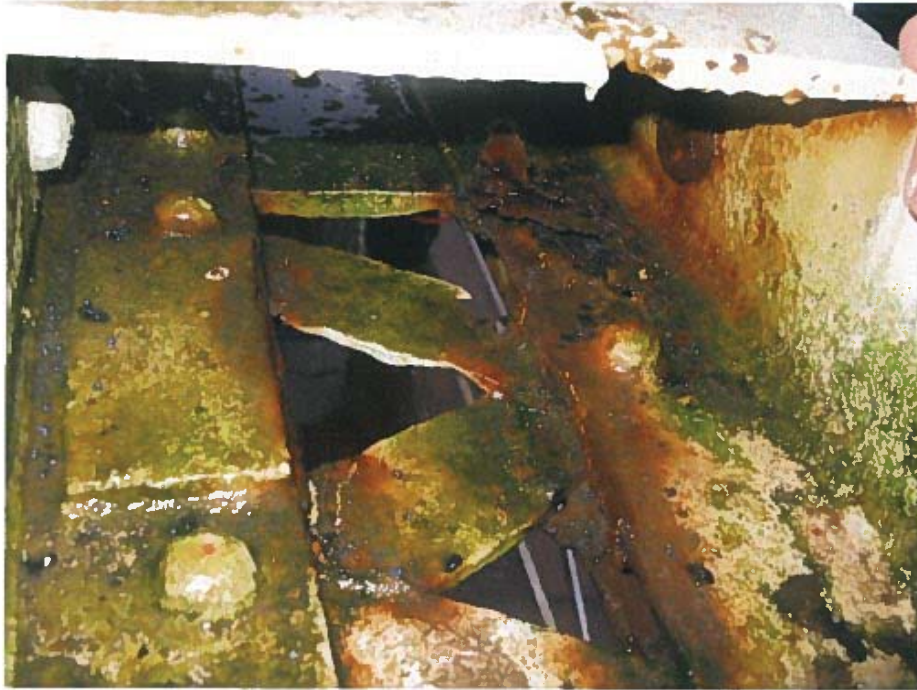
Photograph 13 – Perforation / section loss and corrosion at lacing bars at north truss bottom chord.
