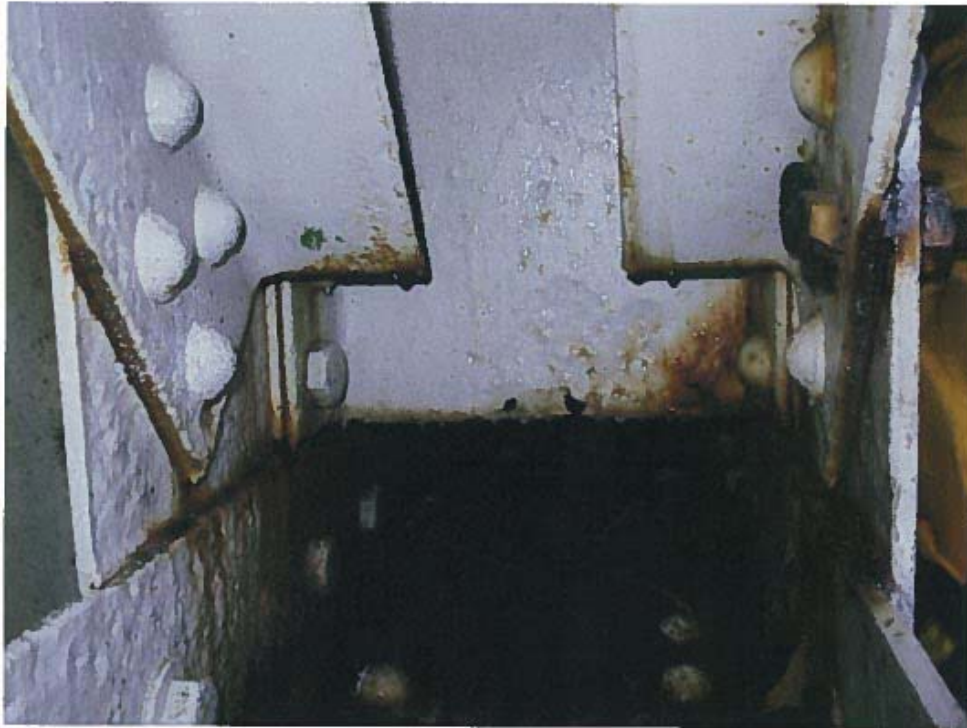
Photograph 23 – Perforation and section loss at vertical member at panel point 4E on south truss.
