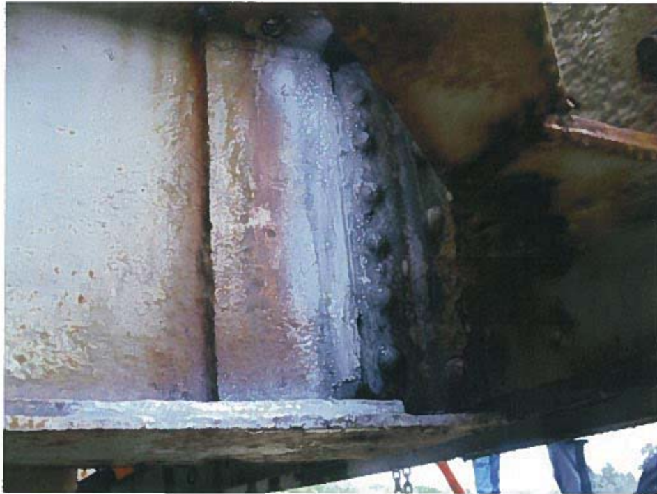
Photograph 47 – Magnetic particle testing of welded reinforcement at the web of the floor beam to the connection angle at panel point 2W.
