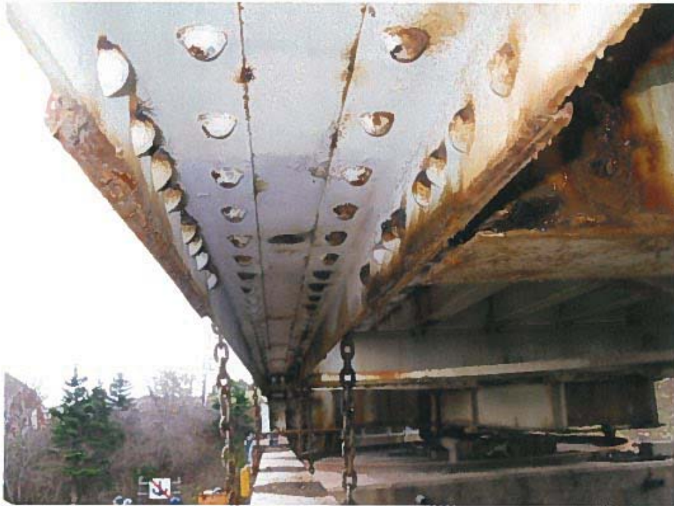
Photograph 9 – Condition of bottom chord along north truss. Note: Medium to severe corrosion.
