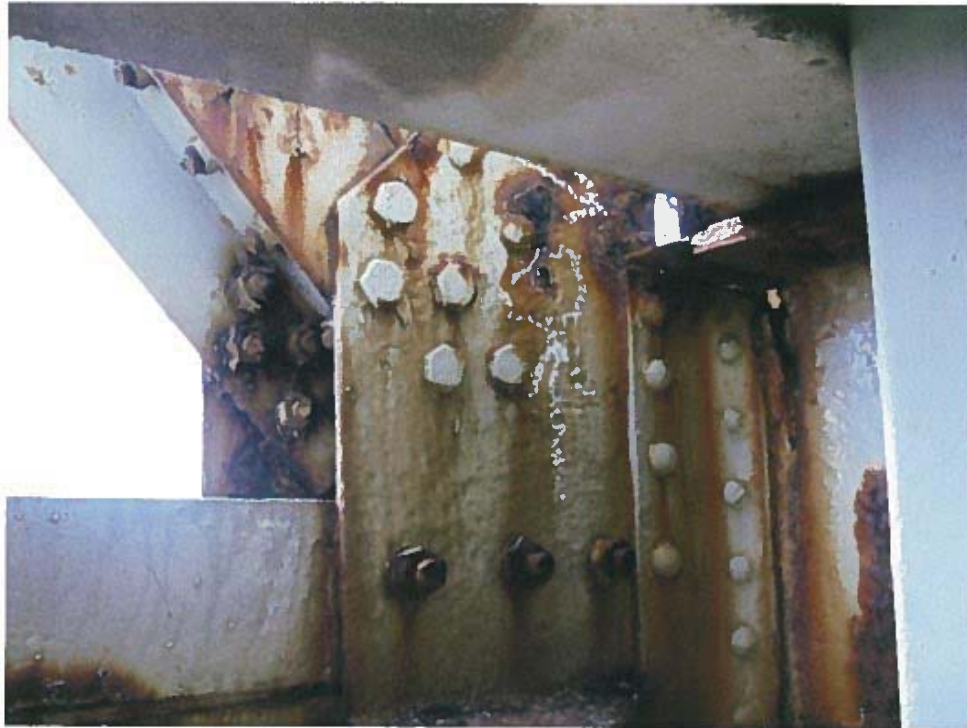
Photograph 15 – Section loss and perforation at gusset plate location at north truss panel point 2W.
