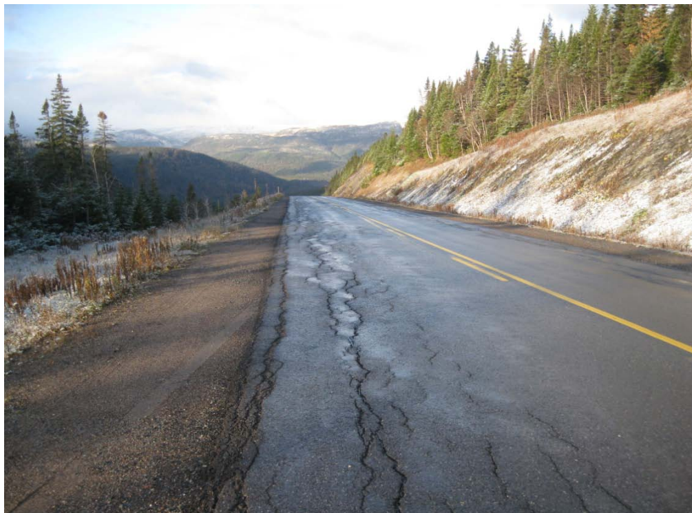
Photo D12: Severe Edge Cracking, Highway 431, Gros Morne National Park
