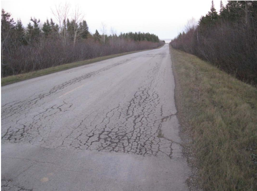
Photo D23: Severe Wheel Track Alligator Cracking – Forillon National Park
