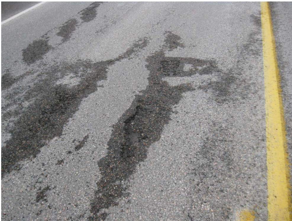
Photo D8: Severe ravelling, TCH, Terra Nova National Park
