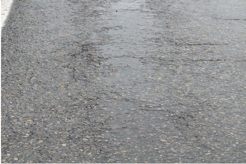
Photo D27: Start of severe ravel leading to alligator cracking (2007 Photo)
