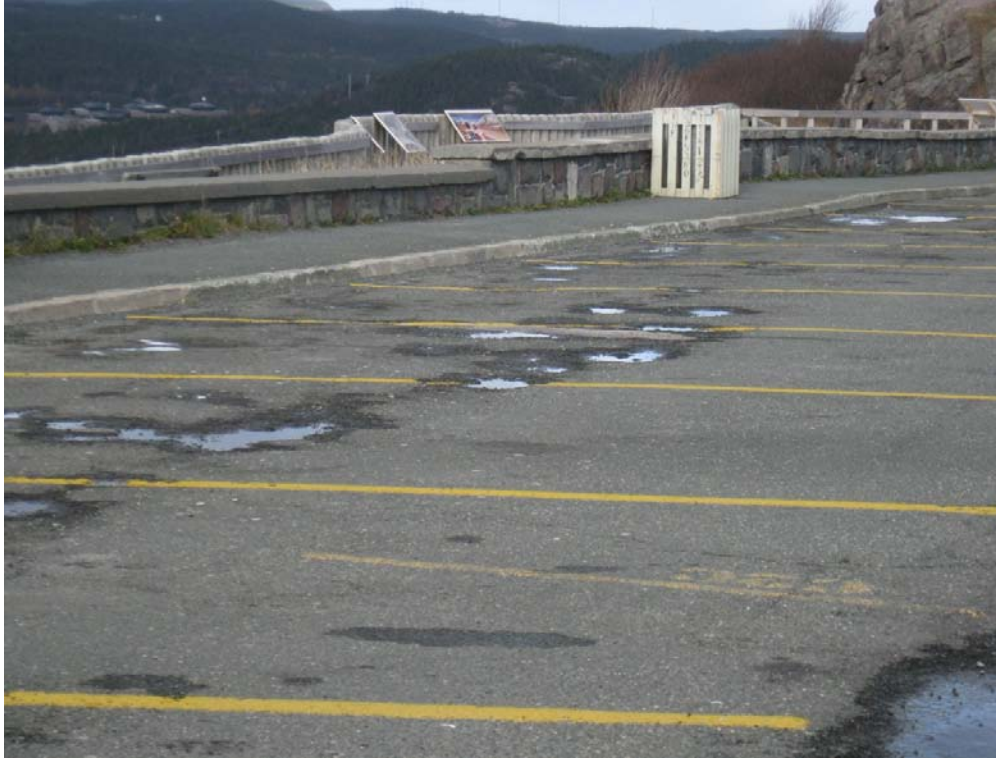
Photo D3: Distortion, Potholes – Signal Hill, Newfoundland
