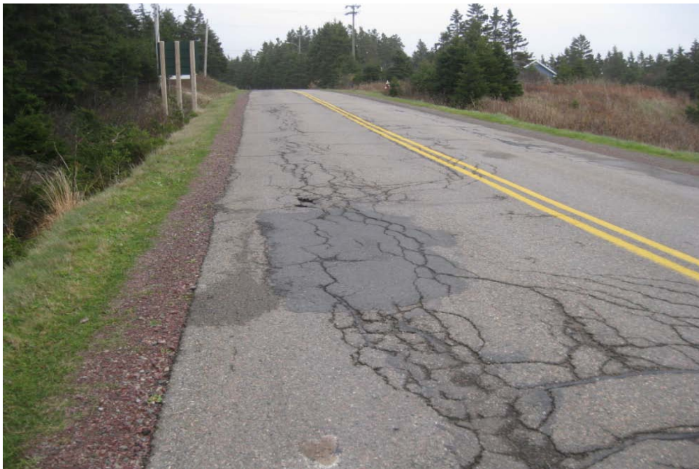
Photo D14: Very Severe Alligator Wheel Track Cracks – Fort Louisbourg
