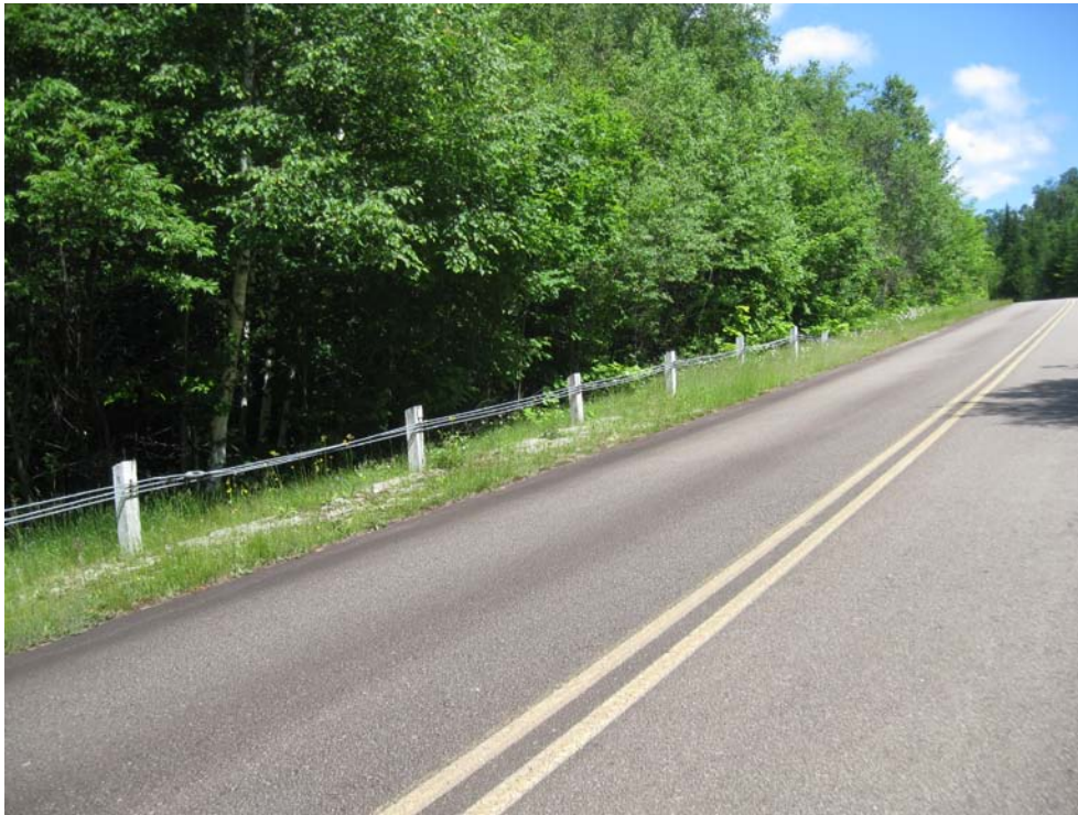
Photo D 34: 3-Strand Guard Rail – loose cables and hence ineffective guardrail La Mauricie National Park
