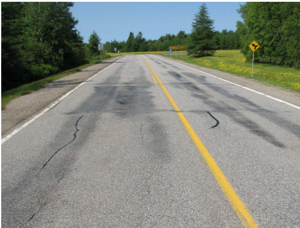
Photo D24: Severe & extensive Bleeding, Kouchibouguac
