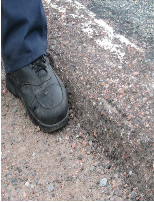
Photo D31: Sharp Drop of Pavement Edge – Cabot Trail, Cape Breton National Park
