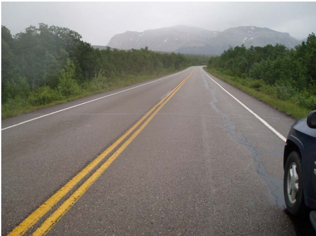
Photo 3: Pavement in Fair Condition PCI 64
