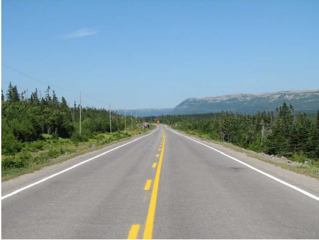
Photo 2: Pavement in Good Condition PCI 71
