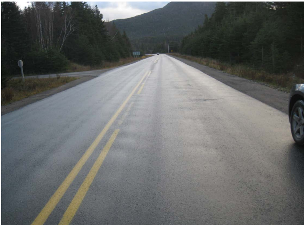
Photo D10: Moderate Ravelling foreground, Severe Ravelling mid-photo –Gros Morne National Park
