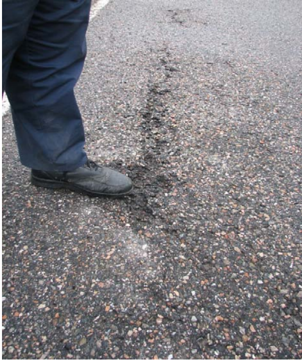
Photo D29: Severe Ravelling Highway 430 Newfoundland (2007 Photo)
