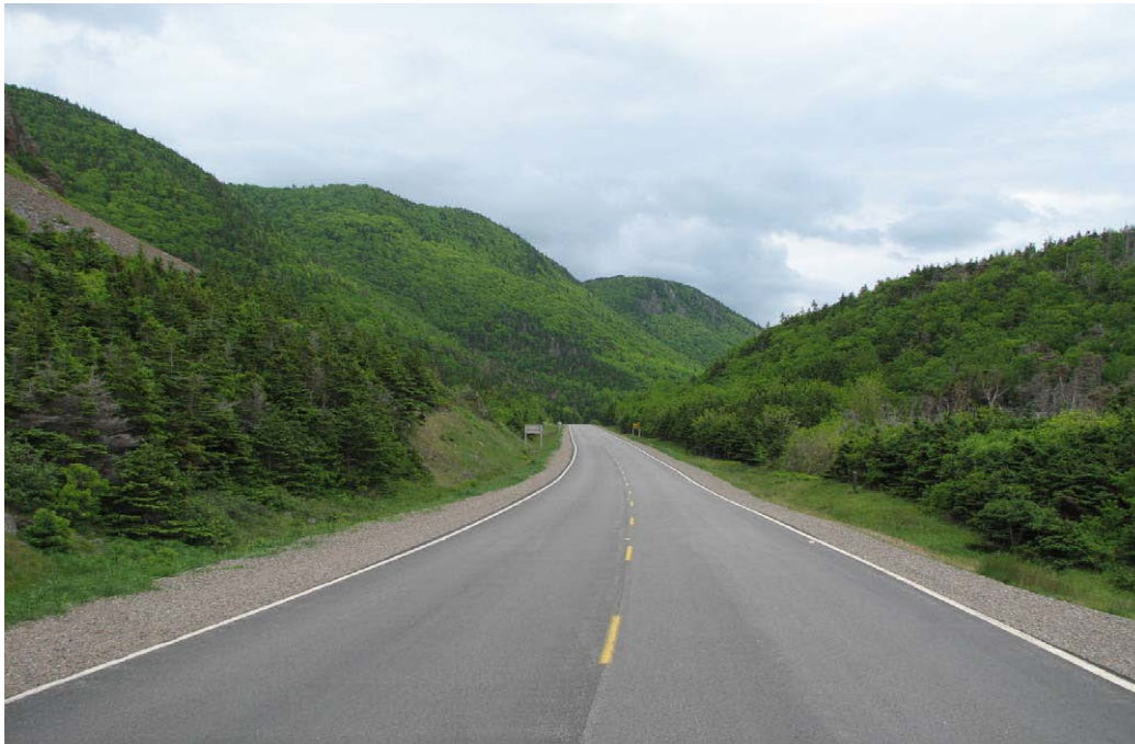
Photo 1: Pavement in Very Good Condition PCI 75
