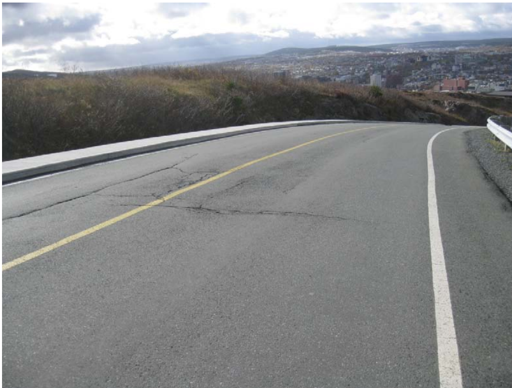
Photo D4: Rutting, Wheel Track Alligator Cracking, Transverse Alligator Crack – Signal Hill Newfoundland
