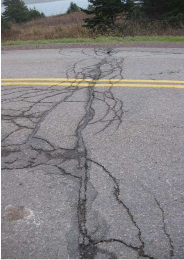
Photo D13: Very Severe Transverse Crack and alligator cracking, Fort Louisbourg
