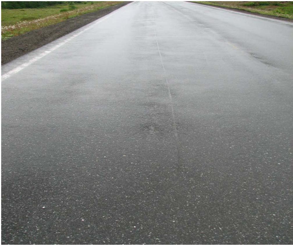
Photo D28: Start of Severe Ravelling Highway 430 Newfoundland (2007 Photo)
