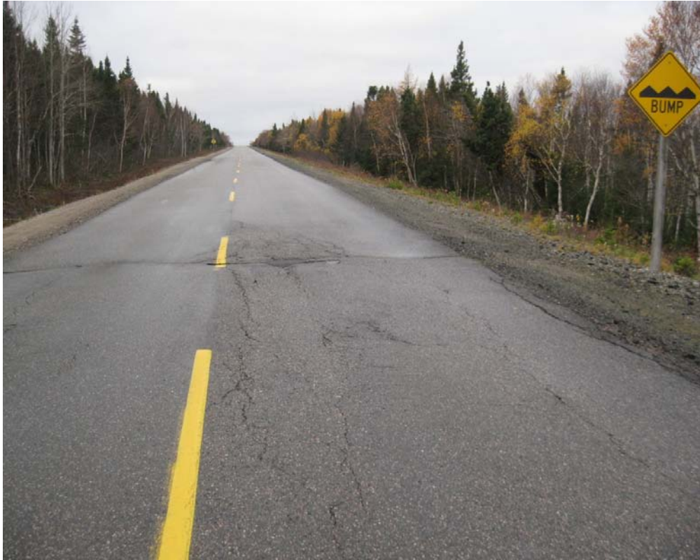
Photo D5: Distortions, Alligator Transverse and Wheel Track Cracking – Eastport Road, Terra Nova NP
