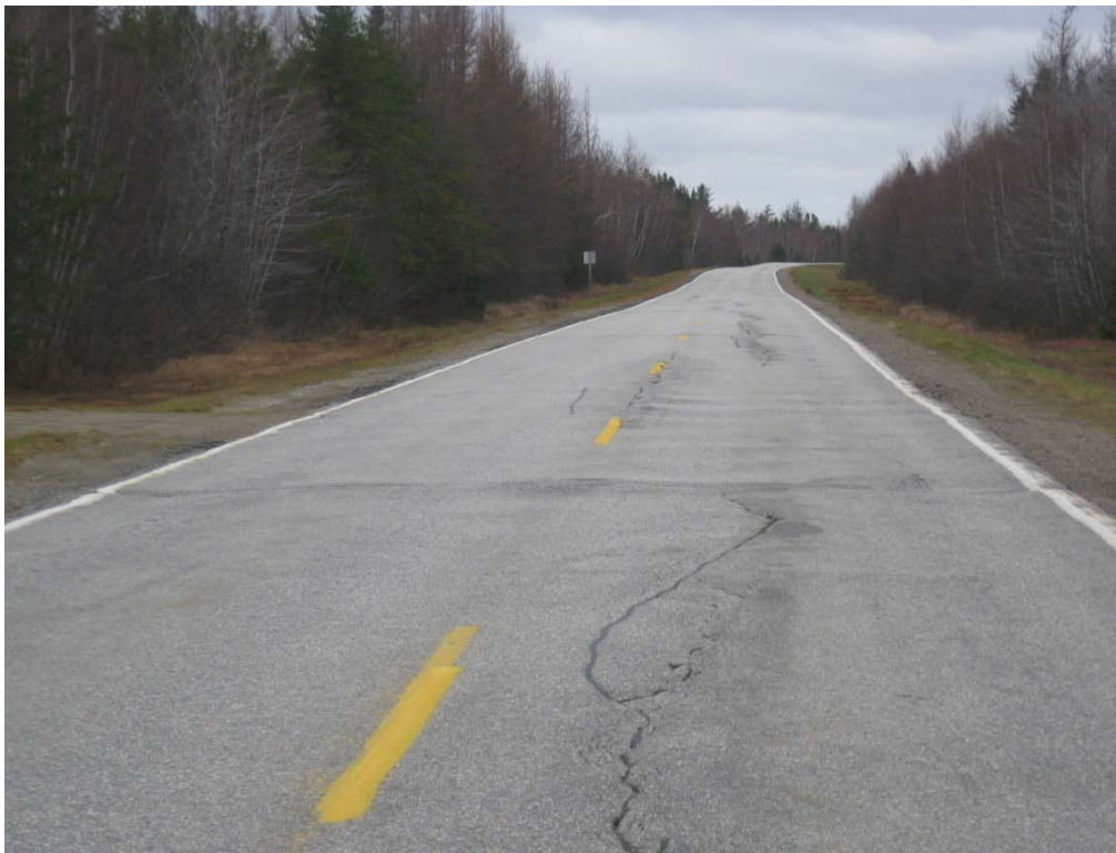
Photo D22: Severe Transverse and Meander Cracking – Kouchibouguac National Park
