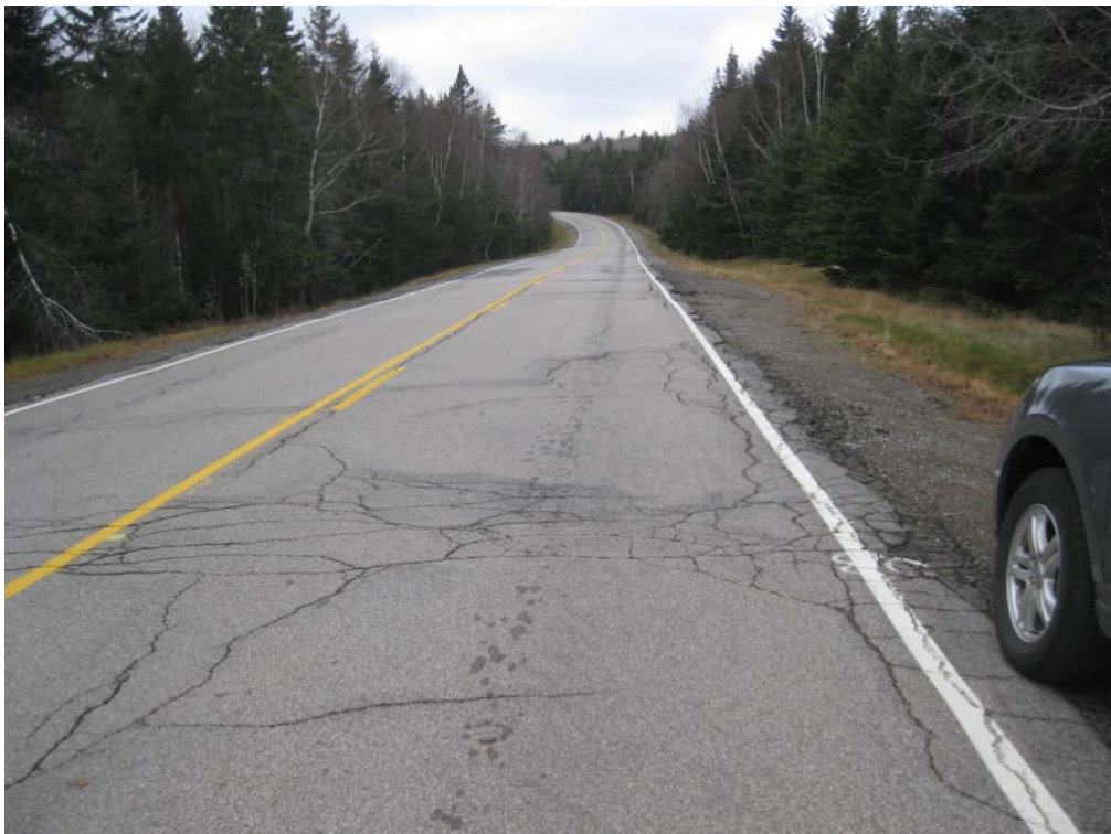
Photo D20: Severe Edge Cracking, Severe Transverse Alligator Cracking – Fundy National Park
