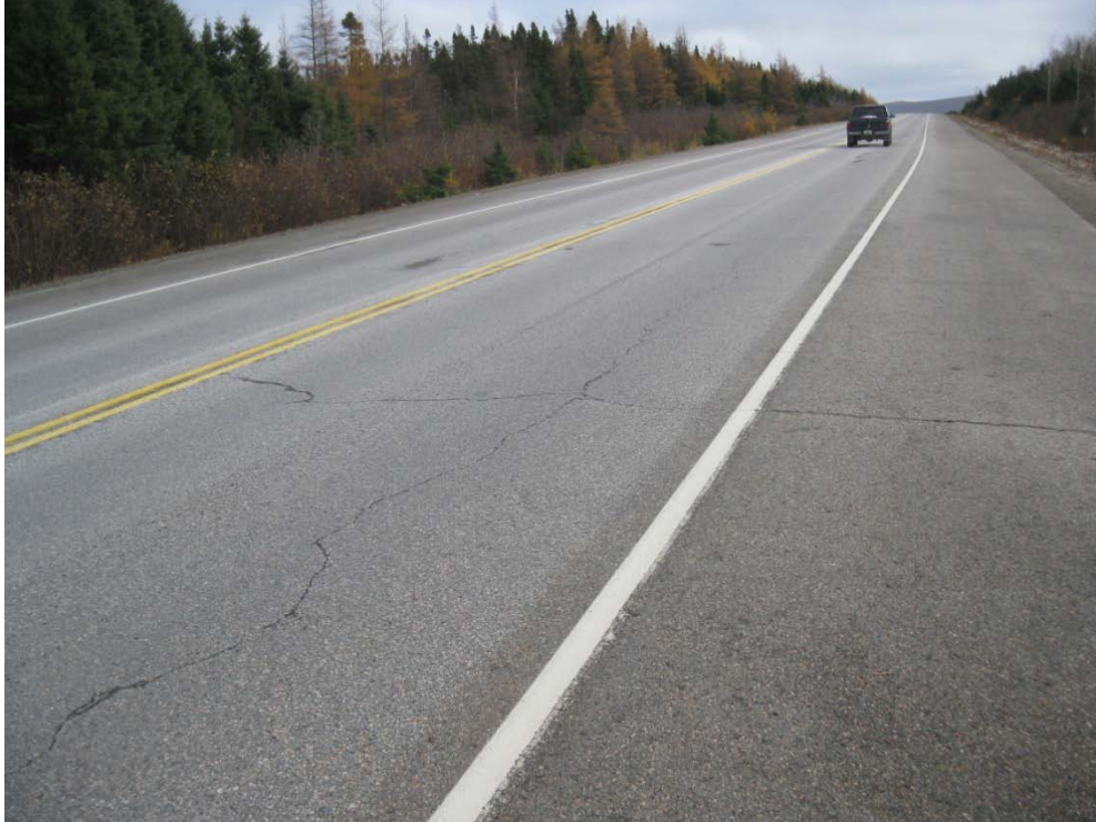
Photo D7: Block, Transverse, and Longitudinal Cracking. Note severe ravelling in left lane, TCH, Terra Nova NP
