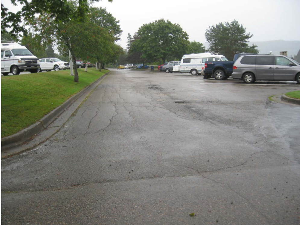
Photo D1: Meander, Transverse, Longitudinal and Very Severe Wheel Track Alligator Cracking –A.G. Bell Museum.
