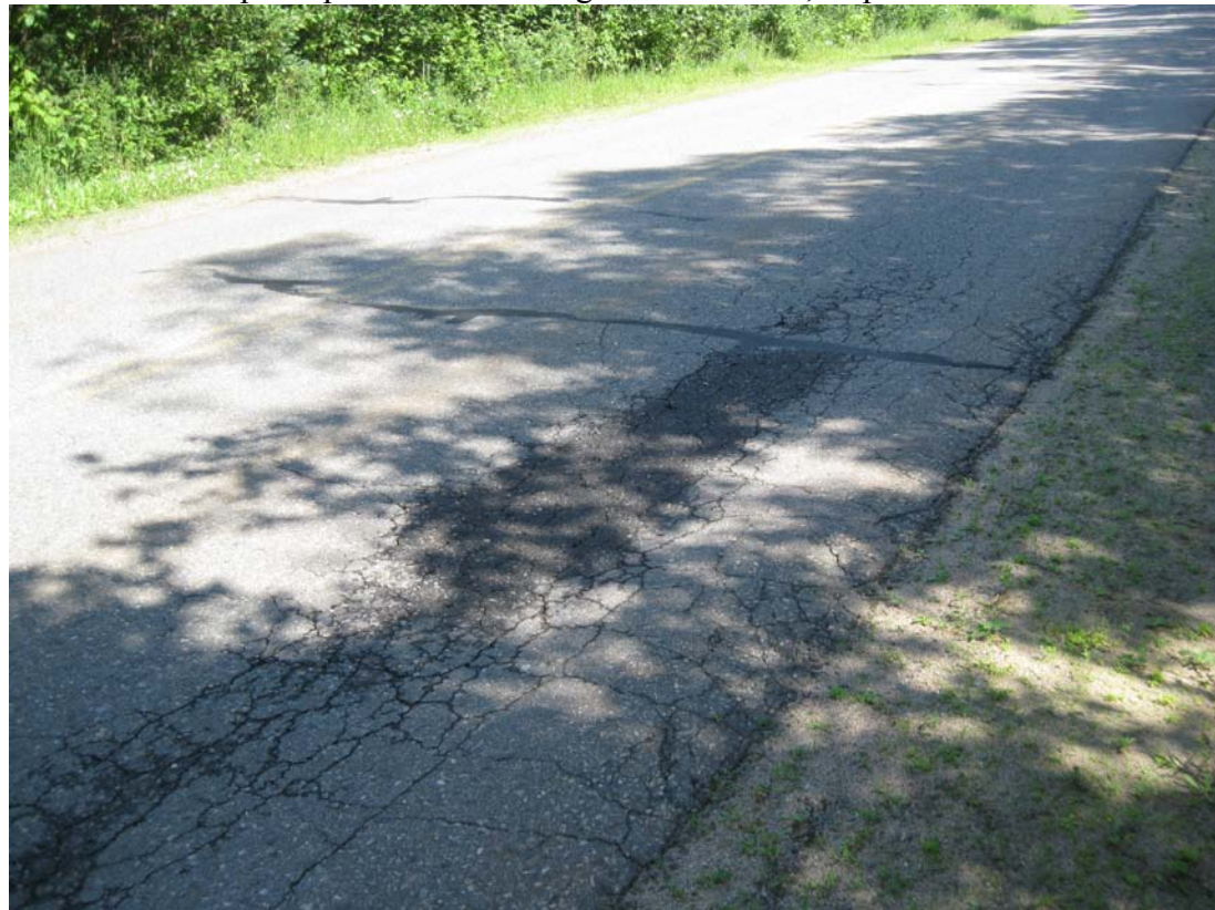
Photo D32: Very Severe Rutting and Alligator Wheel Track Cracking Km 2, La Mauricie National Park
