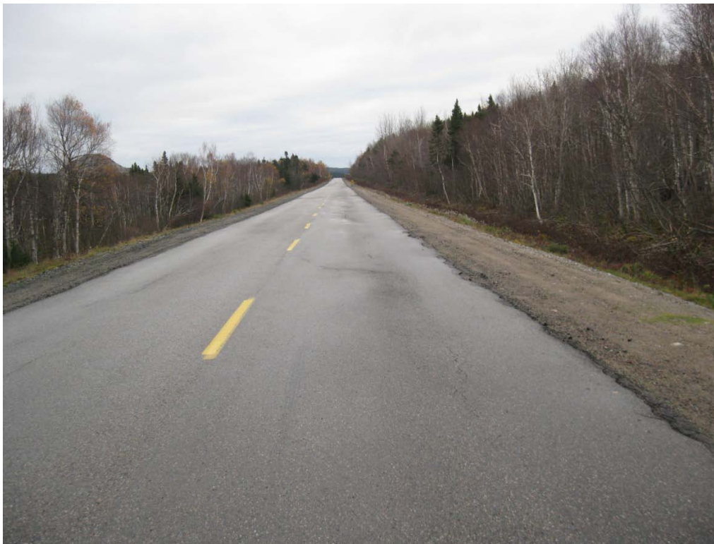
Photo D6: Distortions, Rutting, Edge Cracking - Eastport Road, Terra Nova NP
