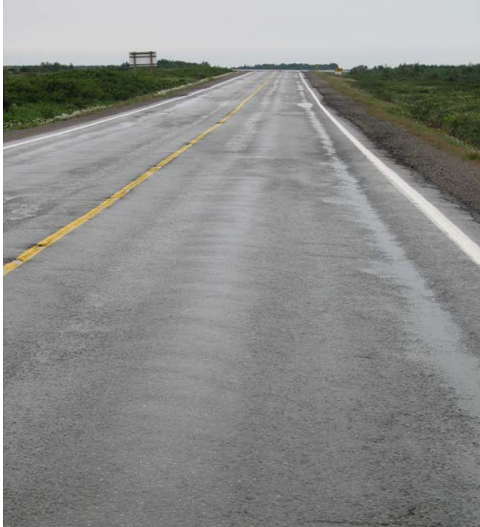
Photo 4: Pavement in Poor Condition PCI 58
