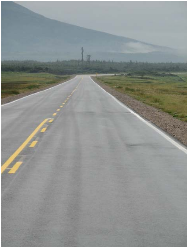
Photo D26: Progression of Ravelling Highway 430 Newfoundland (2007 Photo)
