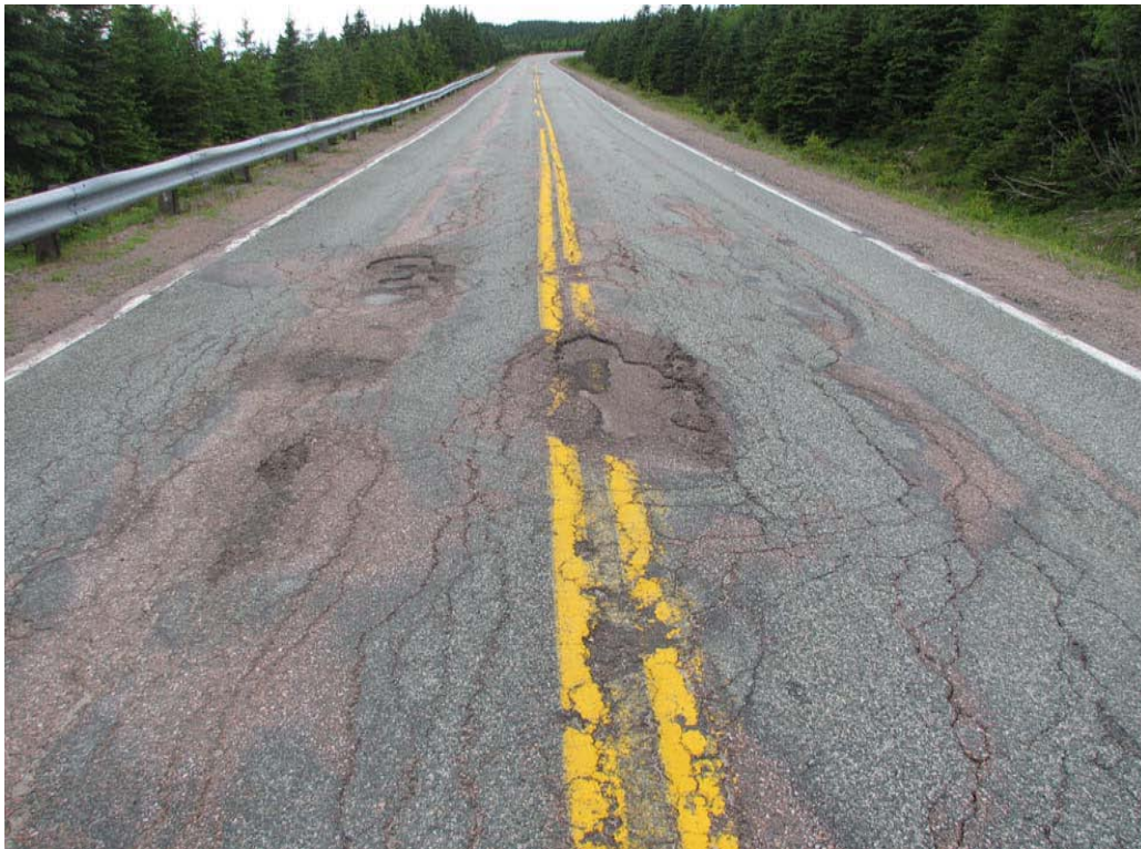
Photo 5: Pavement in Very Poor Condition PCI 43
