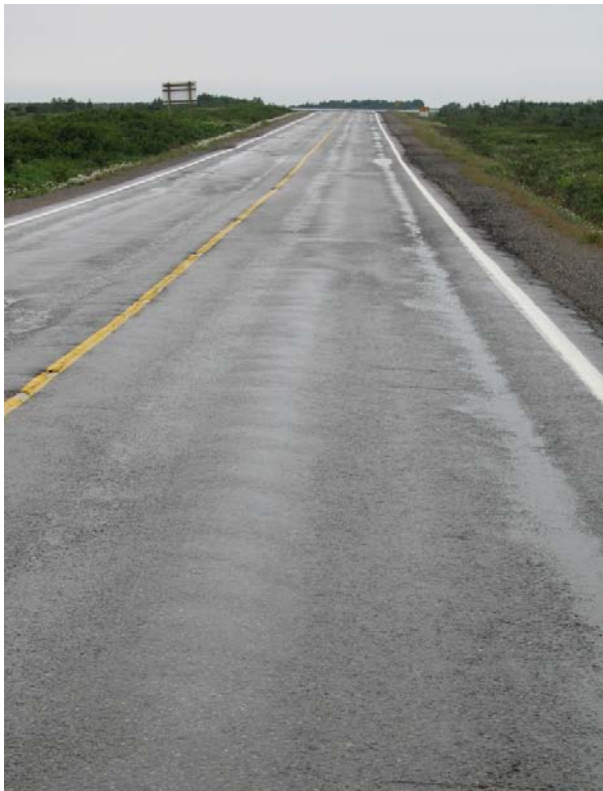
Photo D30: Severe ravelling leading to ruts and alligator cracking Highway 430 Gros Morne National Park (2007 Photo)
