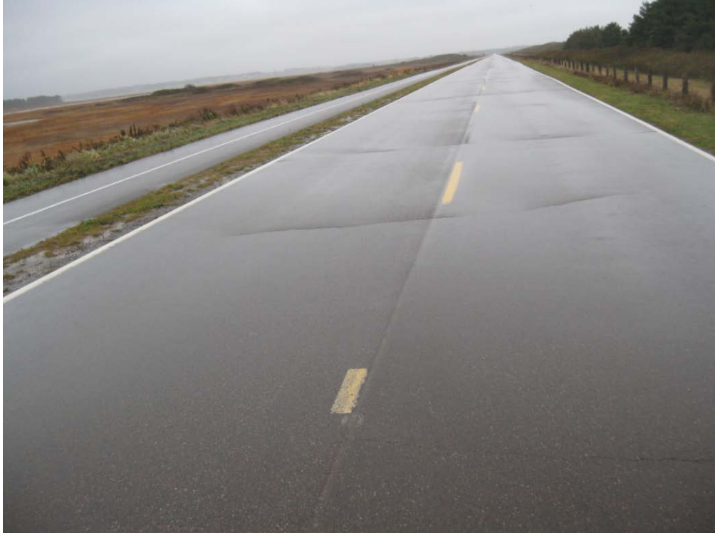
Photo D17: Reflective Transverse Crack on an a Recent Overlay Gulf Shore Highway, PEI National Park
