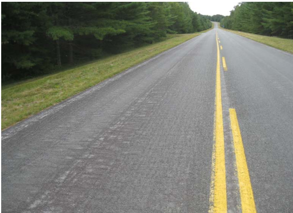
Photo D2: Moderate Ravelling of Micro-surfacing – Kejimikujik
