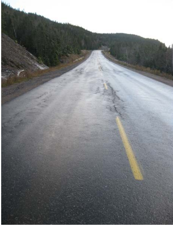
Photo D11: Severe Centreline Crack, Highway 431, Gros Morne National Park
