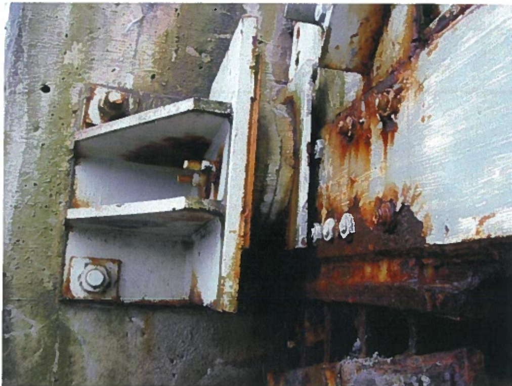
Photograph 14 – Bridge closed end stop located on west fixed abutment
