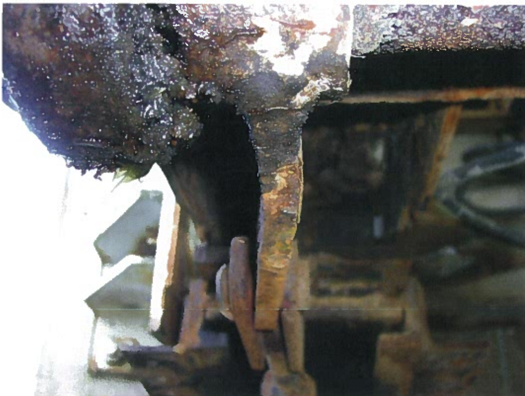
Photograph 4 – South east wedge bent crank arm
