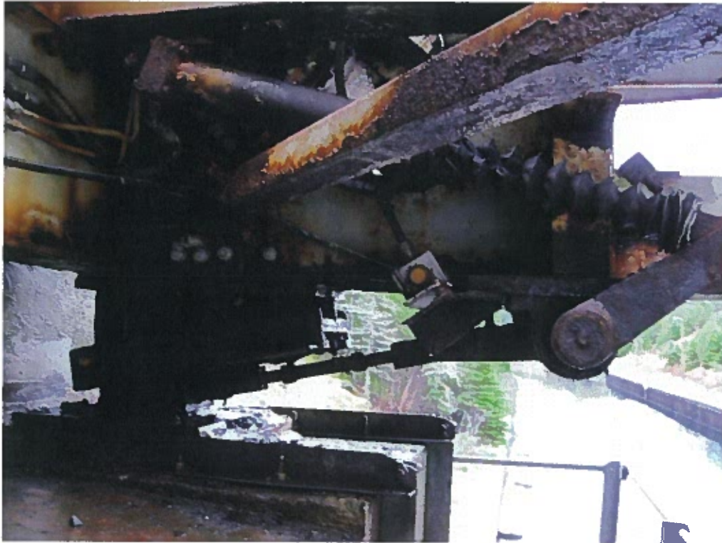
Photograph 1 – Wedge assembly at the south-east end of the movable span.
