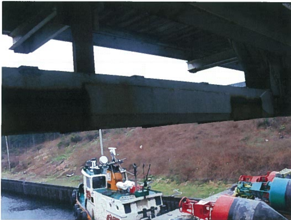
Photograph 26 – Welded reinforcement along south truss (between panel points 4E and 5E).
