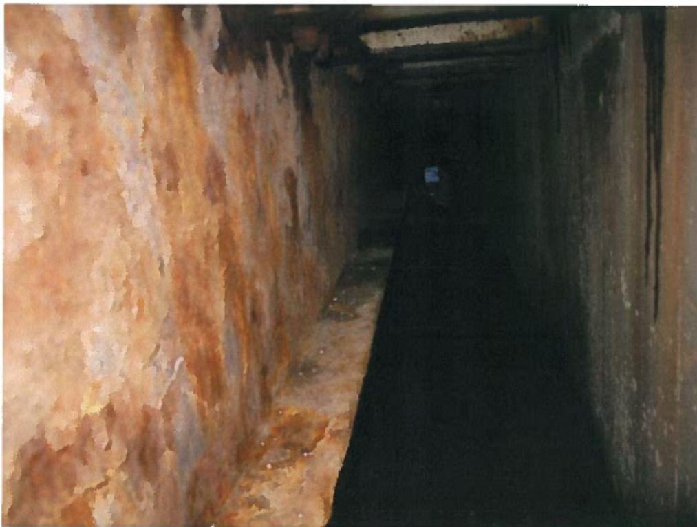
Photograph 33 – Inside face of the end floor beam at east abutment.
