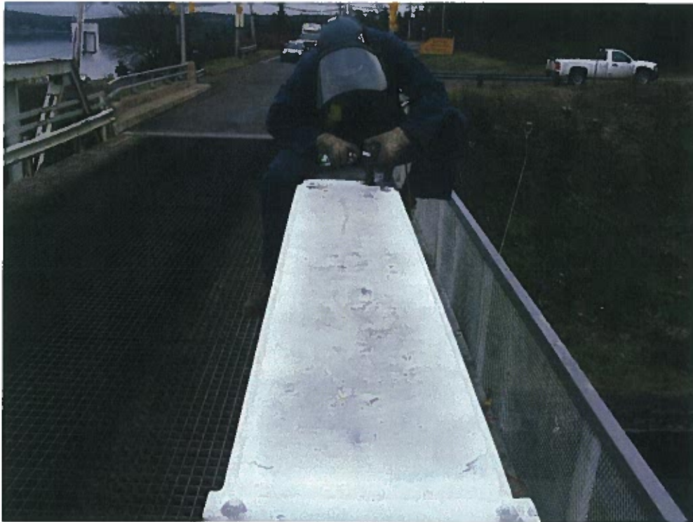
Photograph 41 – Magnetic particle testing of welded reinforcement at south truss top chord between panel points 1E and 3E
