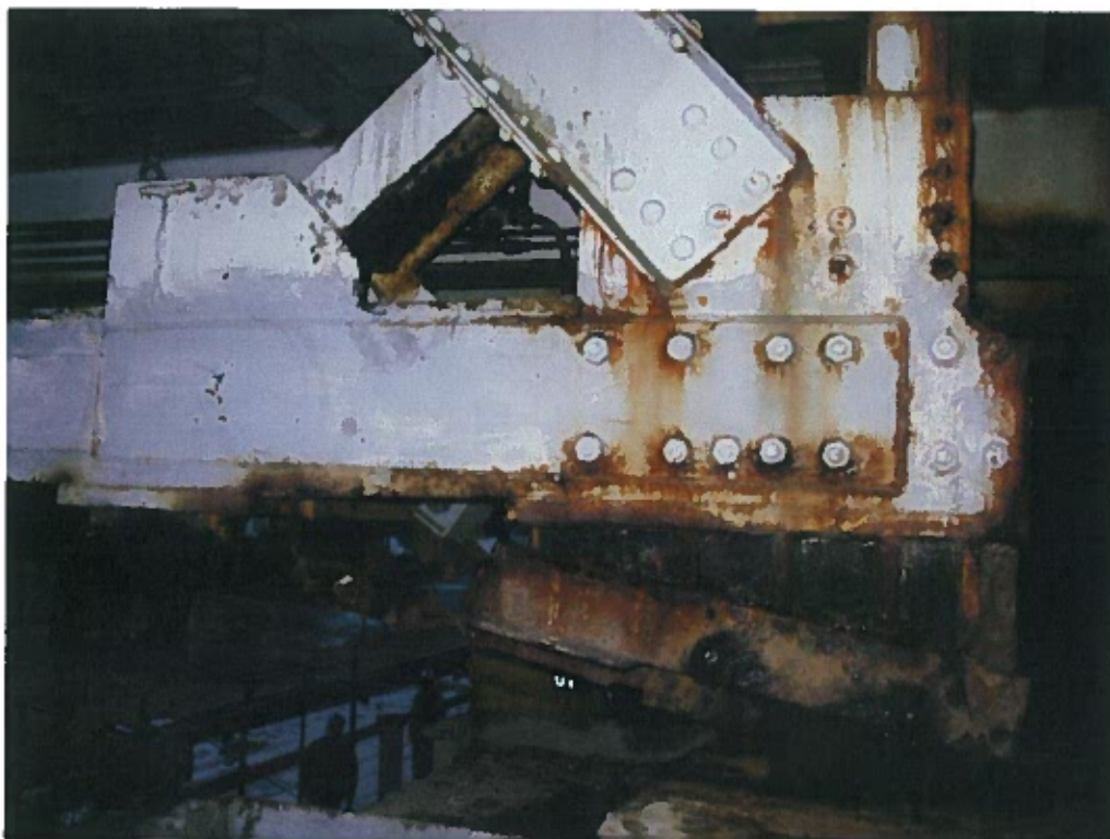
Photograph 27 – Welded reinforcement along south truss at the nose.
