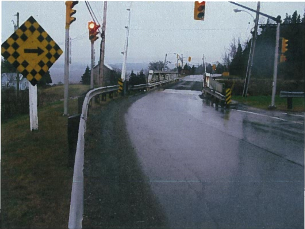
Photograph 2 – West approach looking east.
