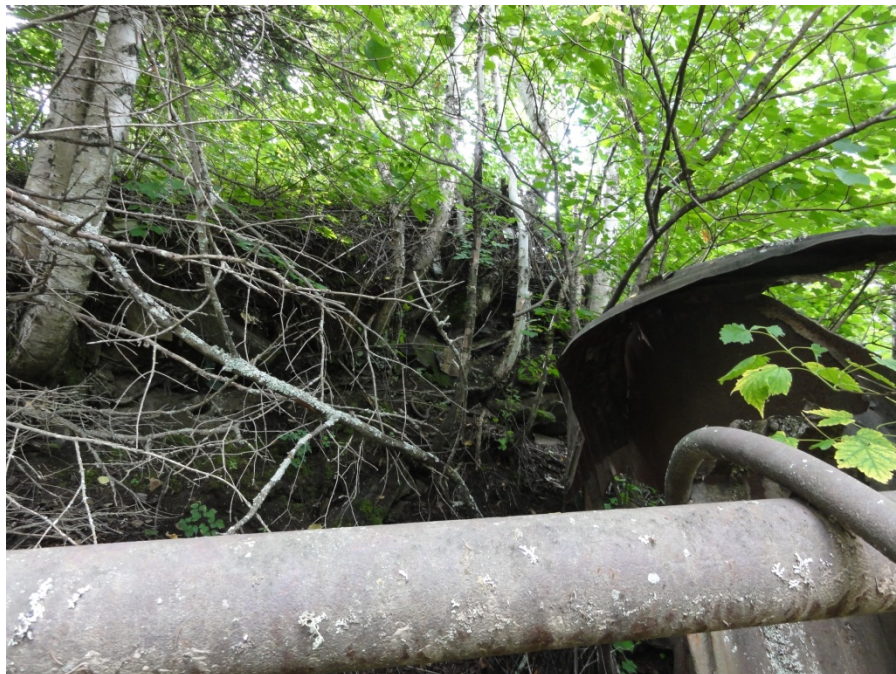
Photograph 4: Portion of the metal culvert visible with trees growing around the waste located along the slope.
