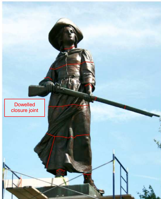
Location of the main (dowelled or bolted) assembly joints
