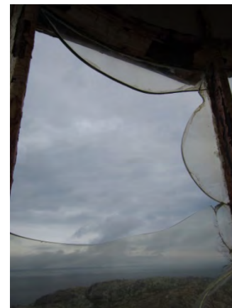
Photo 15: View of broken window pane at top of the light tower.
