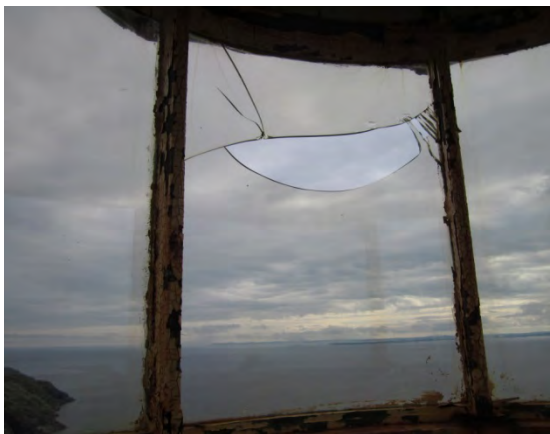
Photo 13: View of broken window pane at top of the light tower.
