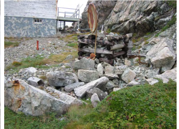
Photo 15: View of septic vent, cribwork foundation and satellite dish.
