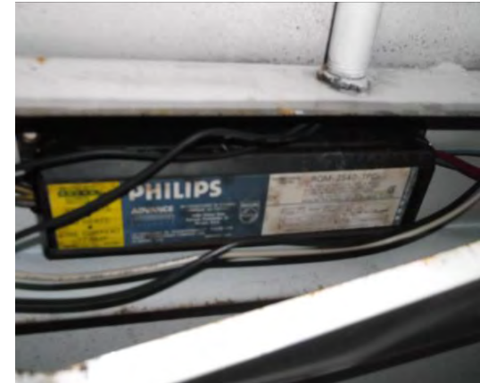
Photo 27: View of Phillips light ballast in equipment building room 1.
