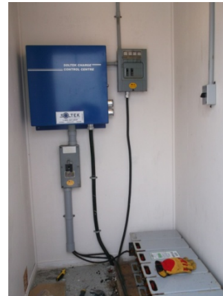
Photo 6: View of solar batteries in solar shed 1.
