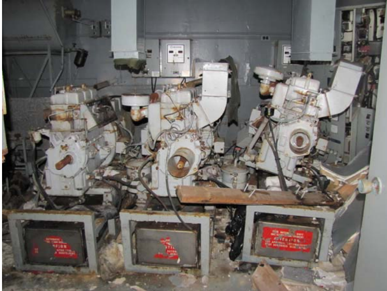
Photo 13: Generators with oil tanks
