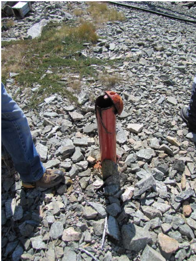
Photo 14: Septic system vent pipe to be cut at grade and capped
