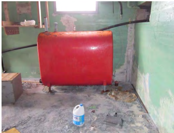
Photo 17: View of 909 L furnace oil AST in basement of dwelling.
