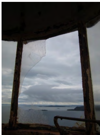
Photo 14: View of broken window pane at top of the light tower.
