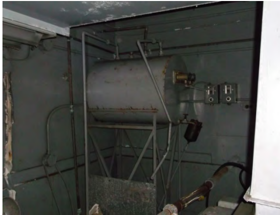
Photo 8: View of AST (approx. 500 L) in room 1 of equipment building.
