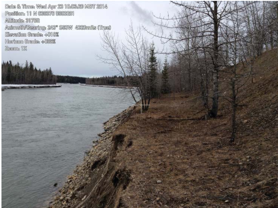
Photo 1: Upstream view from midpoint of works. This is a suitable bench and upper slope for supplementary planting, where vegetation does not currently exist. The eroded lower bank may be staked with live stakes or willow wattles only.
