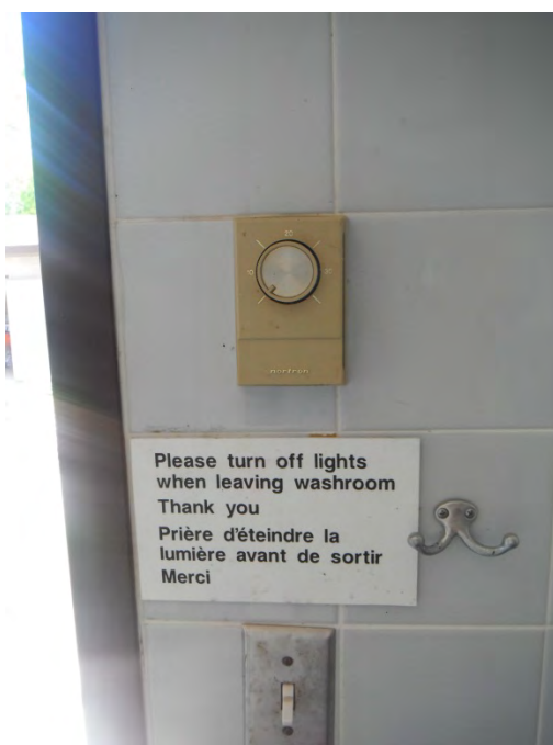
Photo 12 Bi-metallic sensing strip thermostat, no mercury
