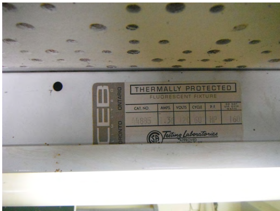
Photo 11 Light fixture manufacturer sticker, found throughout office building, no PCBs
