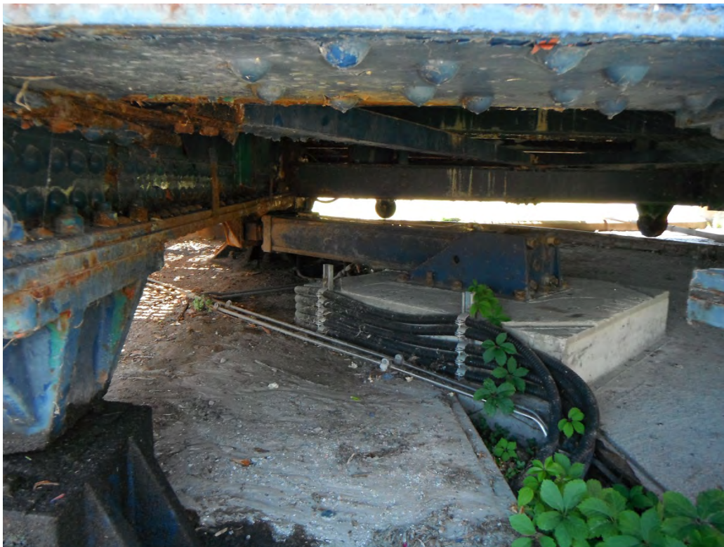
Photo 8 Swing bridge mechanism (underneath), facing west
