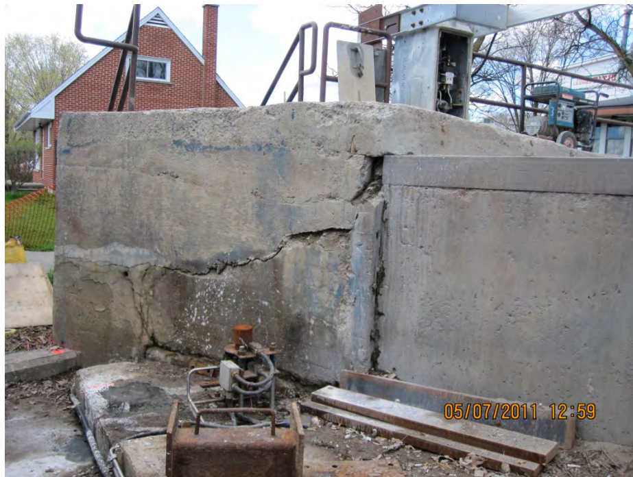
No.22: The west portion of the swing bridge abutment wall (the portion for the sidewalk and stairs). Note the concrete wall was poured in different years and the cracks between different pours.
