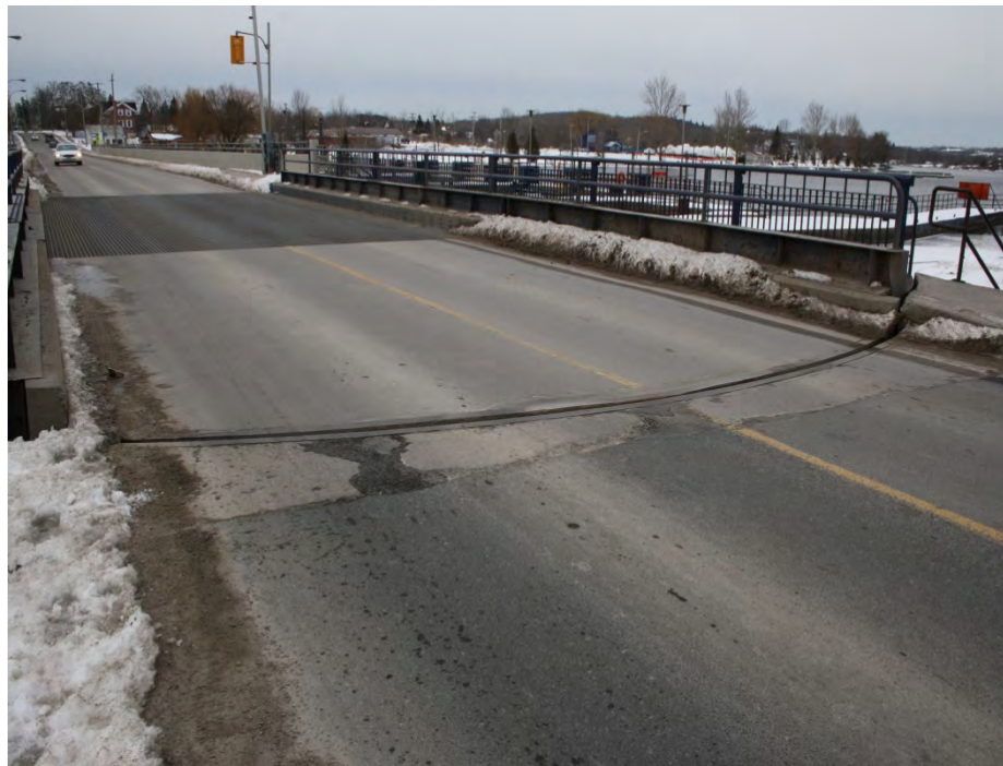
No.8: The swing bridge deck, looking south; a combination steel grate and concrete deck.
