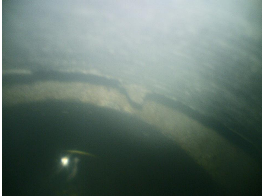
Photograph 7: approximately 2 inches void between the pier concrete and bedrock
