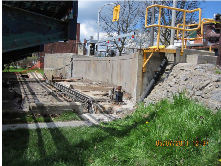
No.7: Overview of the North Abutment Wall; looking west after the swing bridge was swung away.
