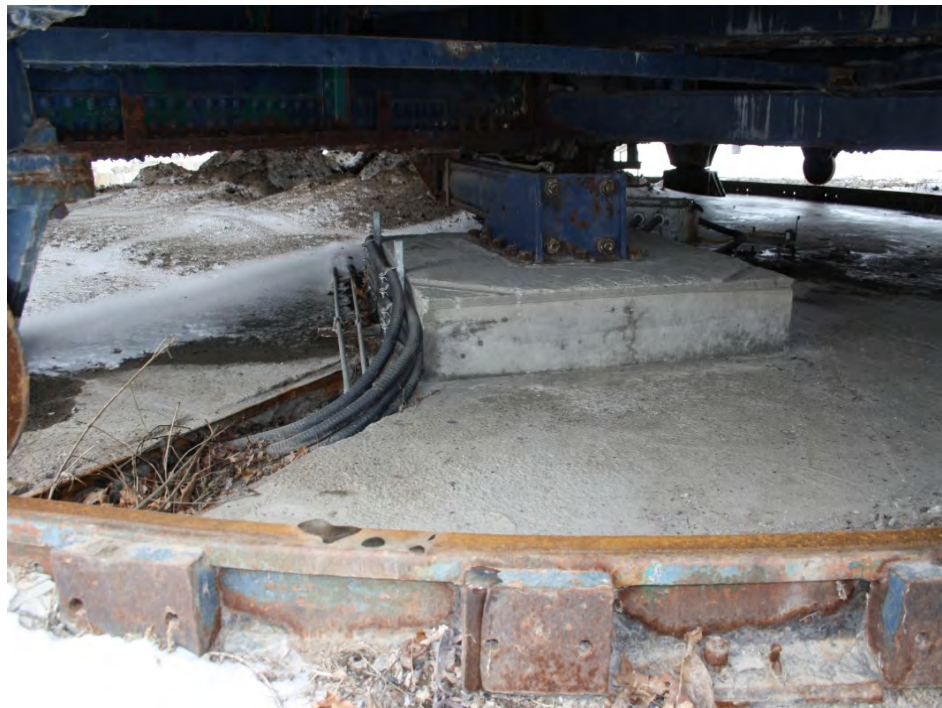
No.18: The central concrete pivot pier; note that the concrete at the surface of the pier appeared to be recently resurfaced; note the hydraulic system and the hydraulic jack used to swing the bridge.
