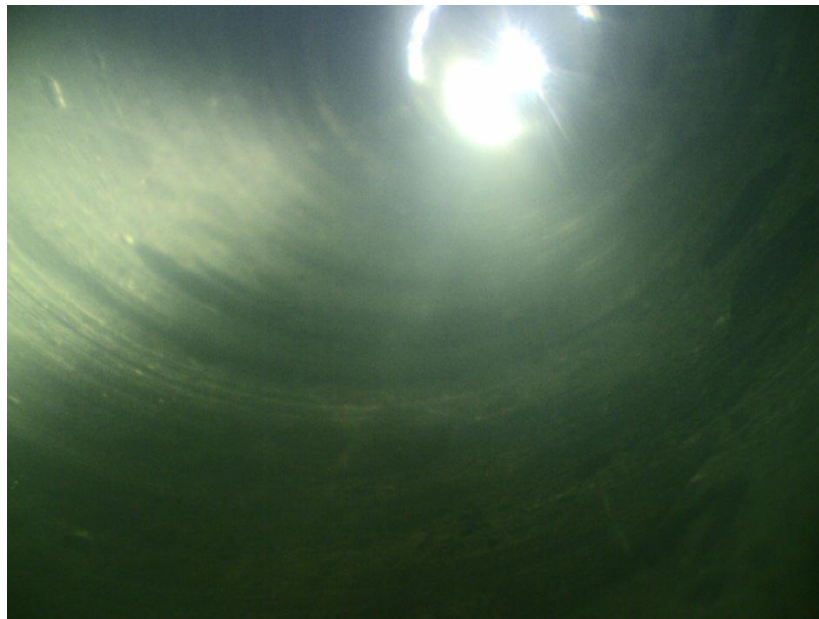
Photograph 2: no cracking or fracture of the pier concrete noted inside the corehole
