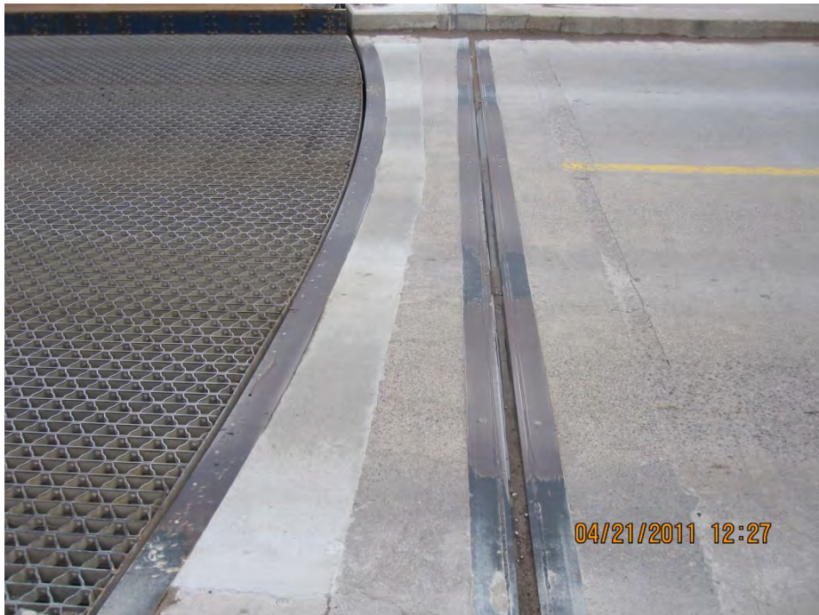
No.10: The south abutment wall and south nosing, looking west. Note the recent repair (lighter colour concrete) south of the steel plate on the abutment wall.
