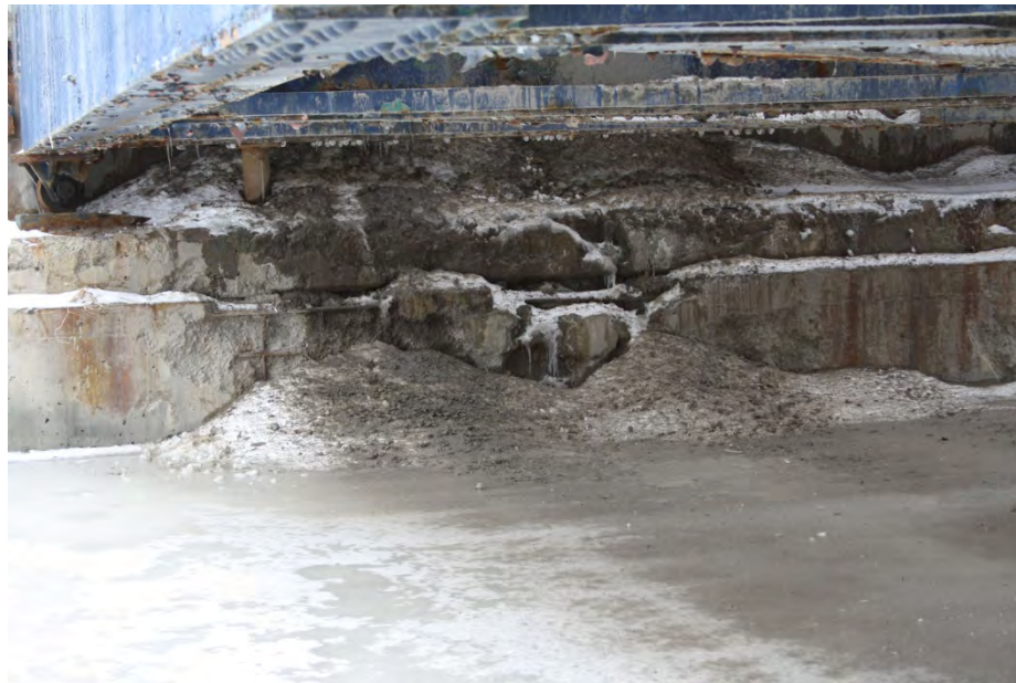
No.11: The south abutment underneath the bridge deck, looking south; note the deterioration of the concrete, exposed steel rebar; note the snow, salt and sands or soils falling from the steel grate deck.
