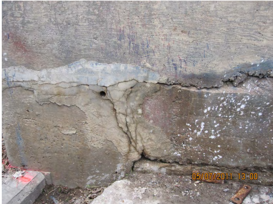
No.23: A close look of the west portion of the swing bridge abutment wall (the portion for the sidewalk and stairs). Note the concrete wall was poured in different years and the cracks between different pours; note the drainage hole on the wall.
