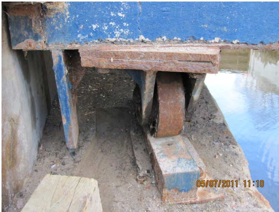
No.14: The south abutment, looking west; note the steel wheel sitting on top of the steel plate to support the bridge during the operational seasons.
