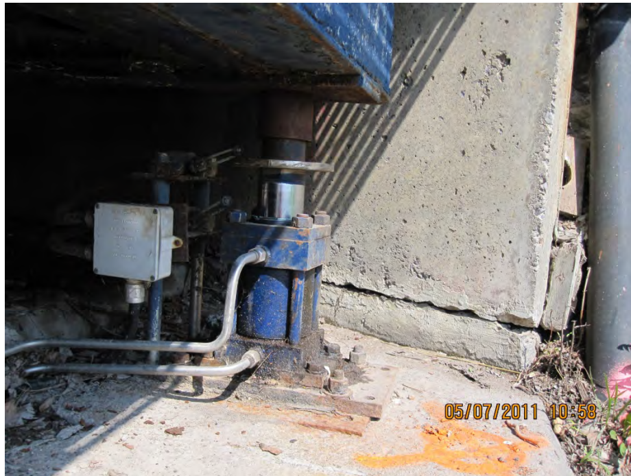
No.17: The north abutment east side of the bridge, looking northwest; note the support hydraulic jack used to support the bridge during the operational
