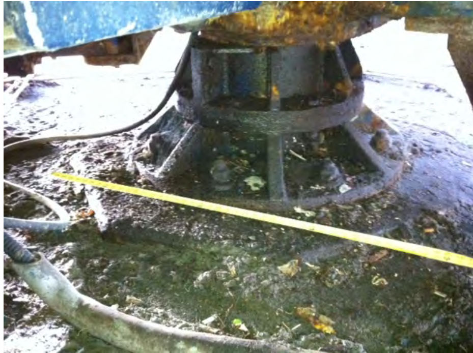
No.21: Central pintle with a round steel plate (Approx. Dia. 0.8m) bolted on concrete platform slightly elevated above the pier concrete.
