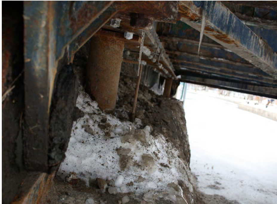
No.13: The south abutment underneath the bridge deck, looking west; note the snow, salt and sands or soils falling from the steel grate deck; note two steel posts used to support the bridge during the non-operational seasons.
