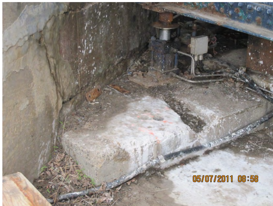
No. 16: The north abutment west side of the bridge, looking northeast; note the support hydraulic jack used to support the bridge during the operational seasons.
