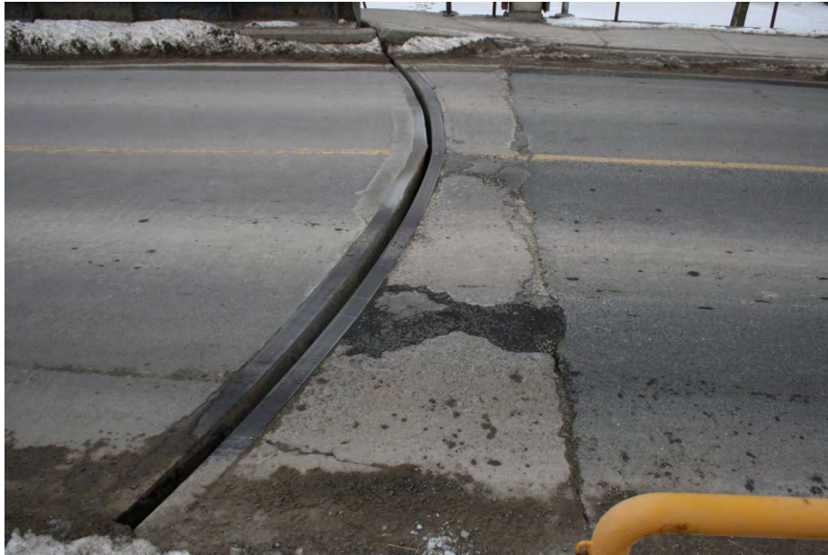
No.9: The north abutment wall and north nosing, looking west. Note the recent repair south of the steel nosing plate on the bridge deck; note the deterioration on top of the abutment wall and asphalt patch repair.
