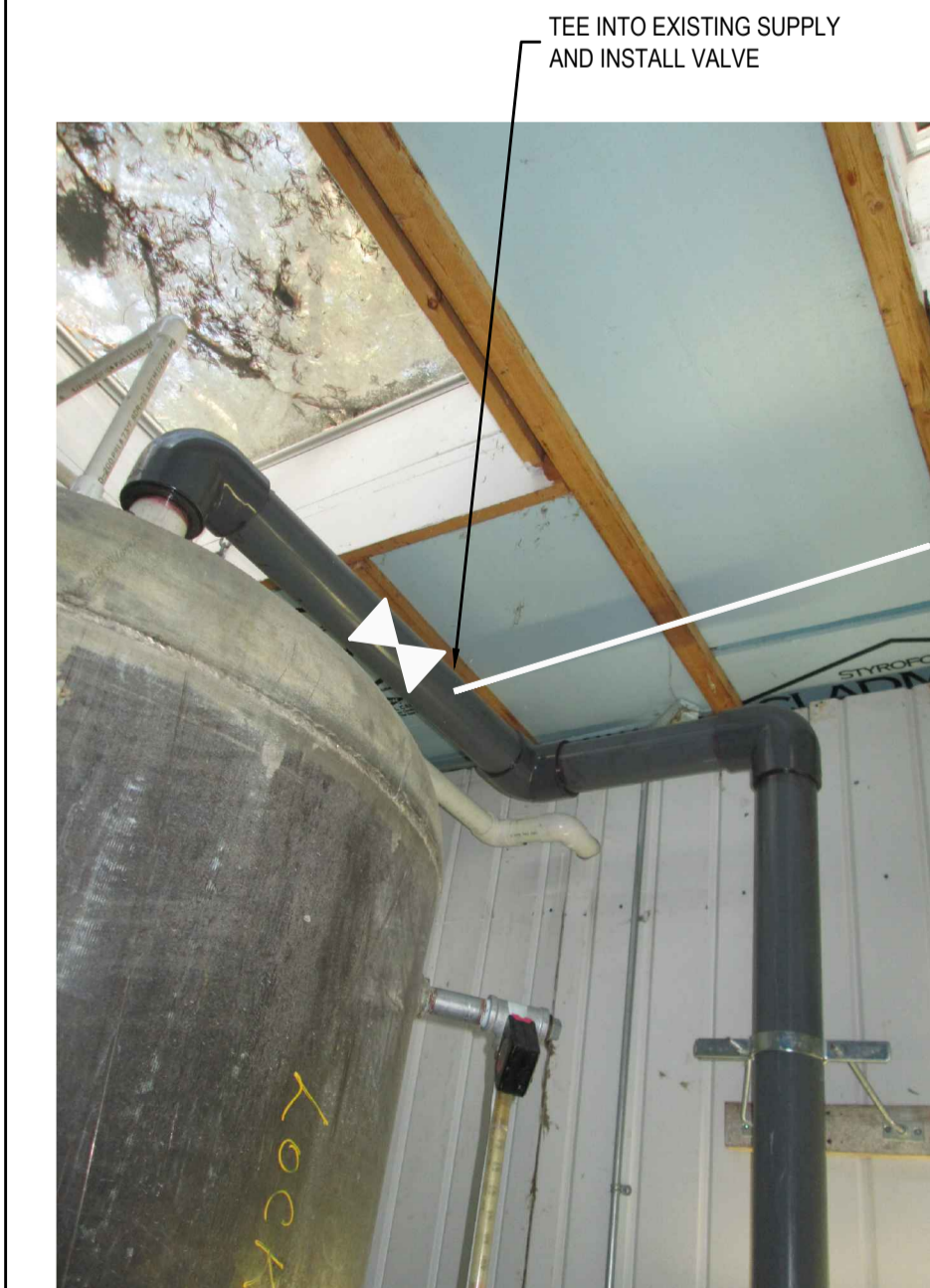
P3 VALVING AND PIPING UPPER DOMESTIC PUMP HOUSE ROOM 2 (PROVISIONAL)
