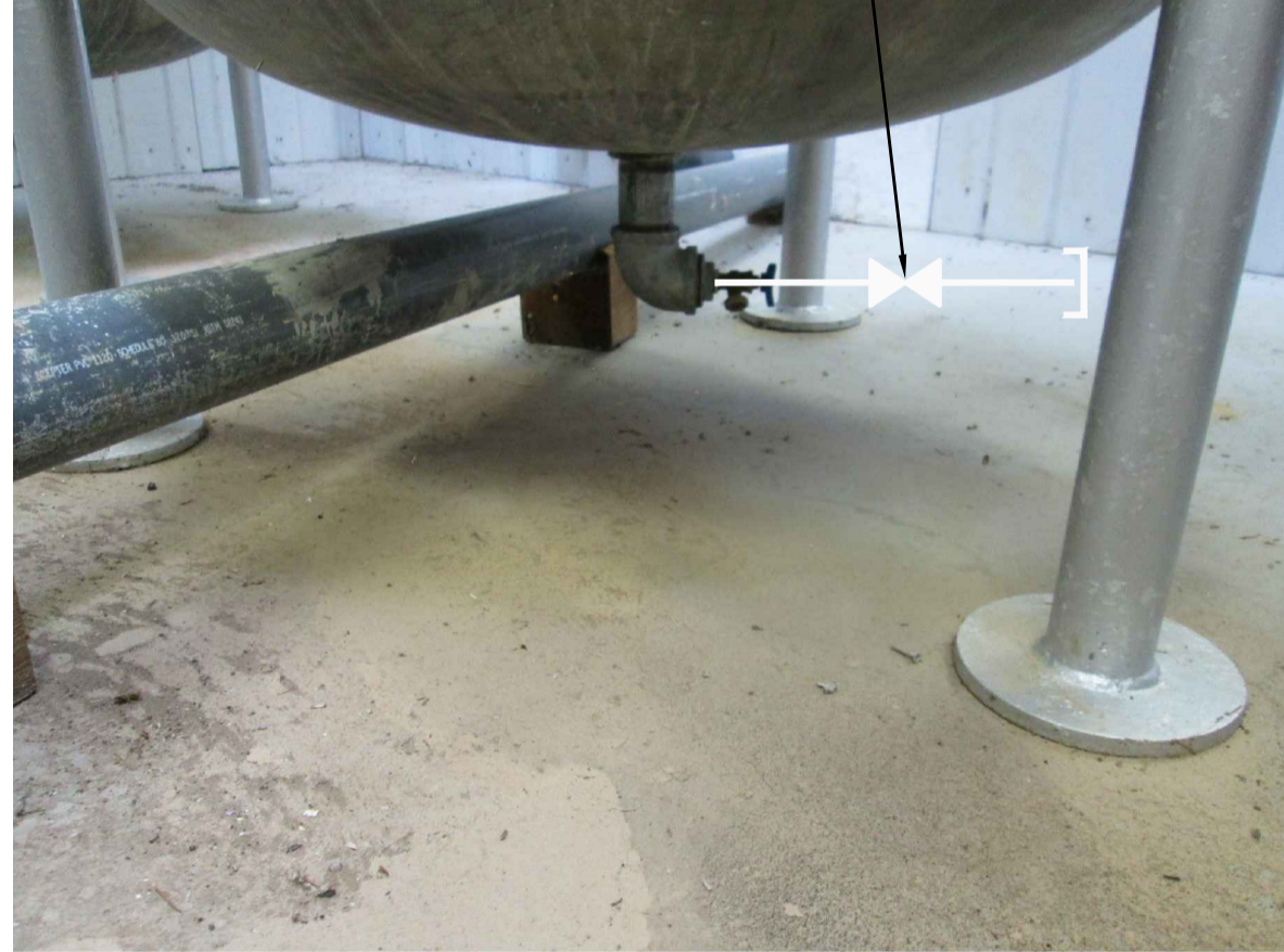
P5 UNDER DRAIN UPPER DOMESTIC PUMP HOUSE ROOM 2 (PROVISIONAL)
