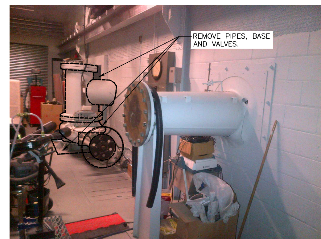
5 INTERIOR PIPING REMOVAL DETAIL ME01 SCALE N.T.S.
