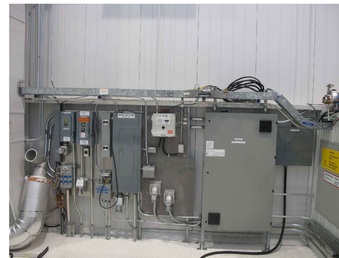
OVERALL VIEW, REMOVE WIRE TRAY
