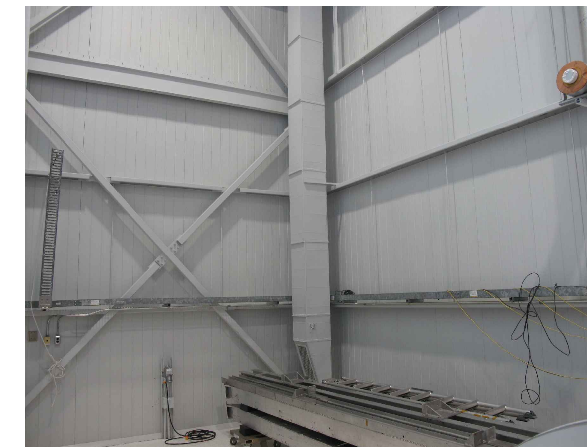
REMOVE EXISTING WIRE TRAY C/W ALL SUPPORTS & ACCESSORIES.
