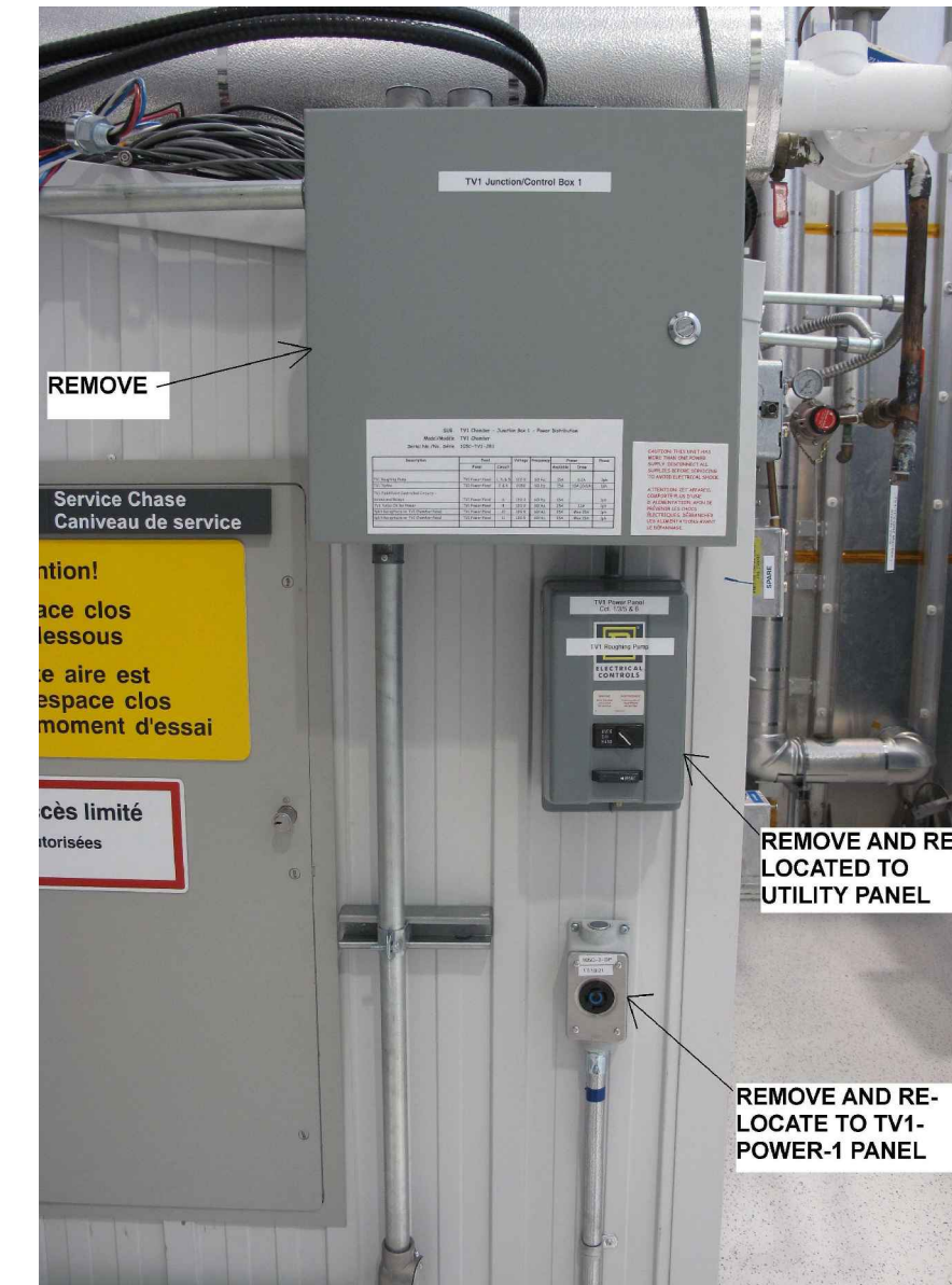
ITEMS TO BE REMOVED FROM SIDE OF SERVICE CHASE
