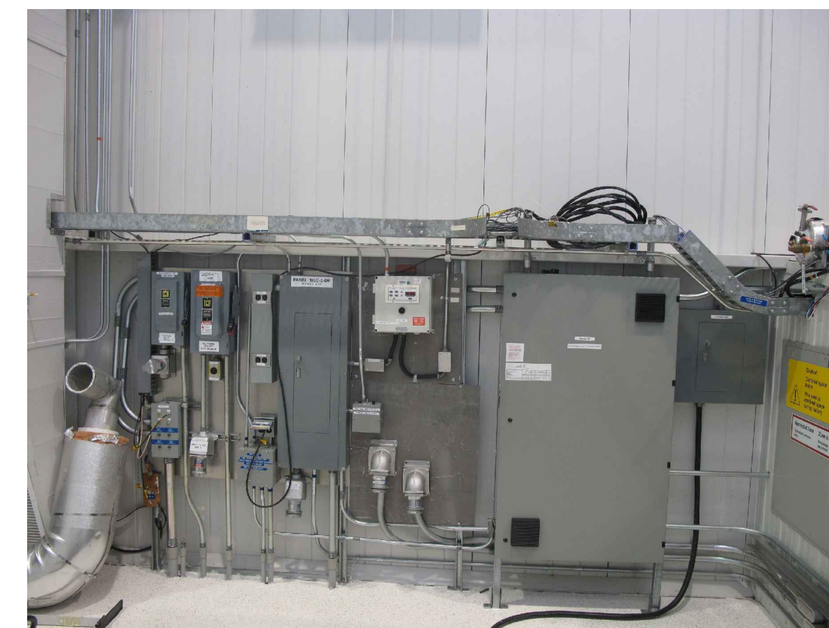
OVERALL VIEW, REMOVE WIRE TRAY
