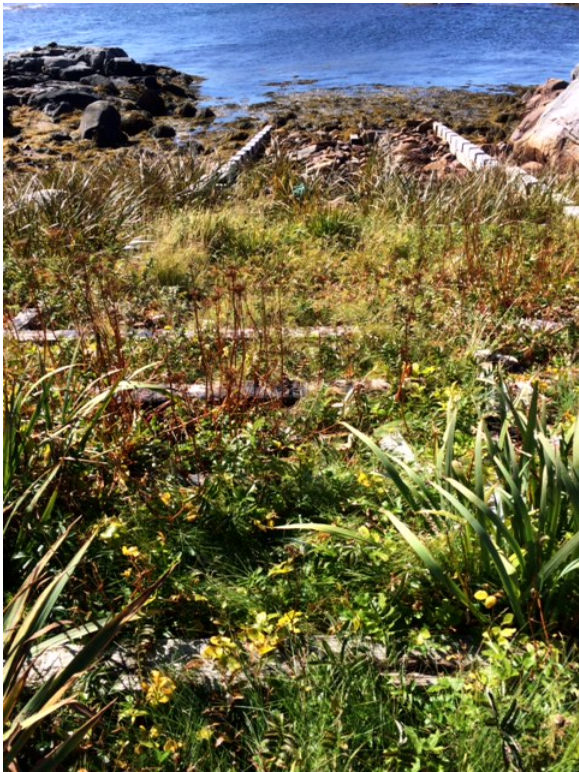
Creosote timber used in slipway
