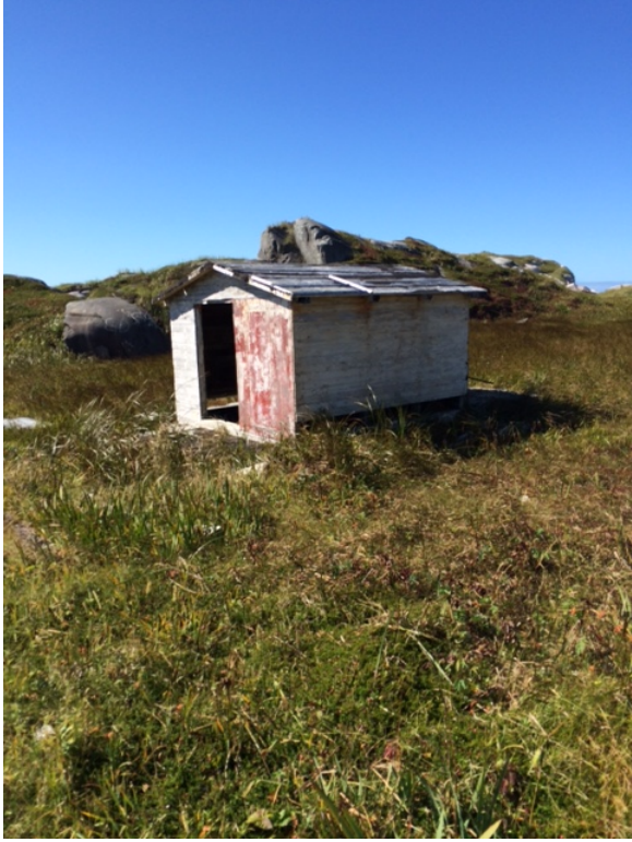
Shed at Slipway Site
