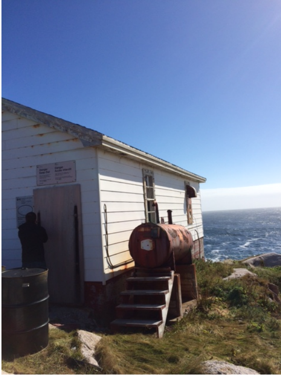
Showing equipment building
