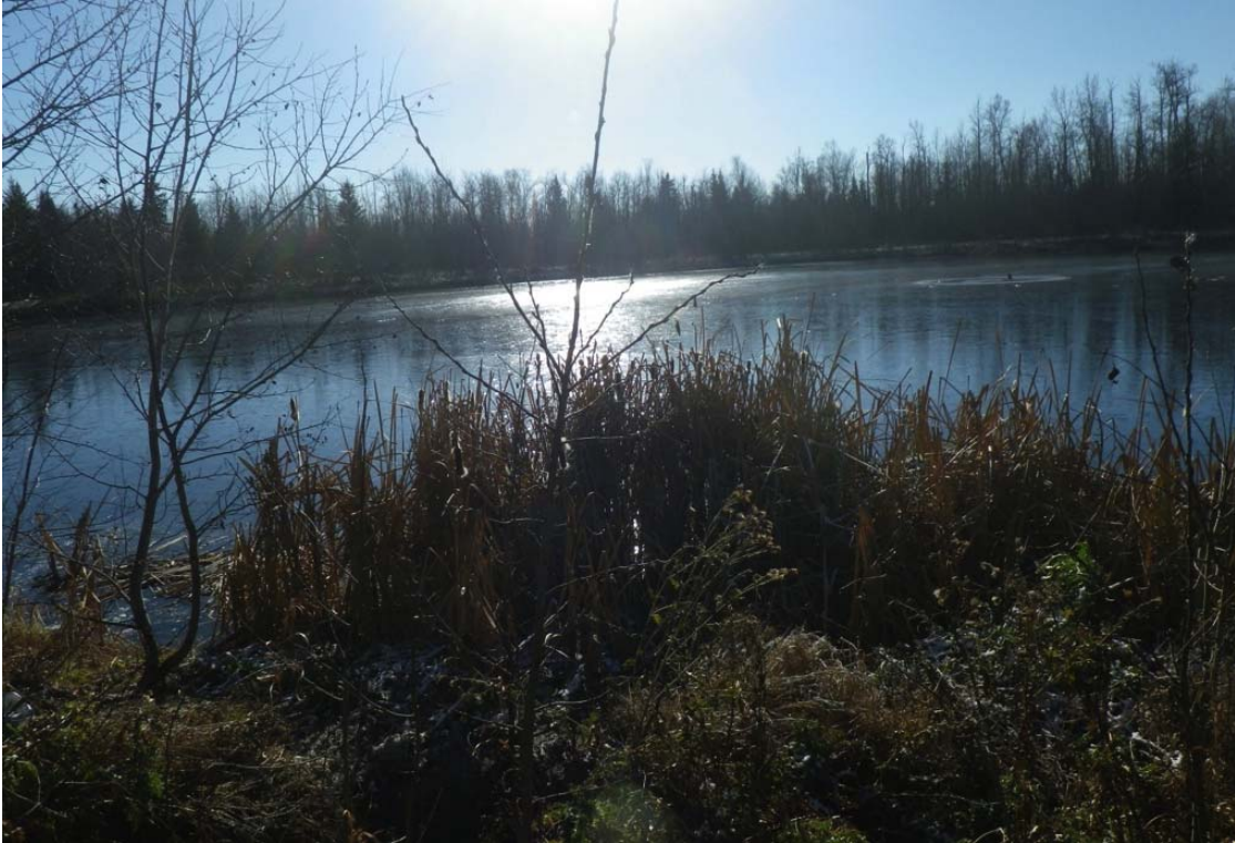
Photograph 1: Wide-angle view of Astotin Lake Recreation Area Sewage Lagoon, facing south, with inlet pipe visible at the far right of the photo.
