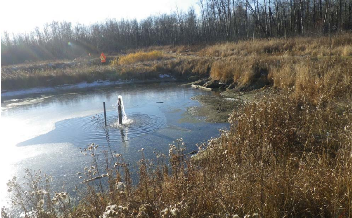
Photograph 9: Administration Area Sewage Lagoon inlet pipe, with effluent flowing into settling cell. Photo taken facing west.
