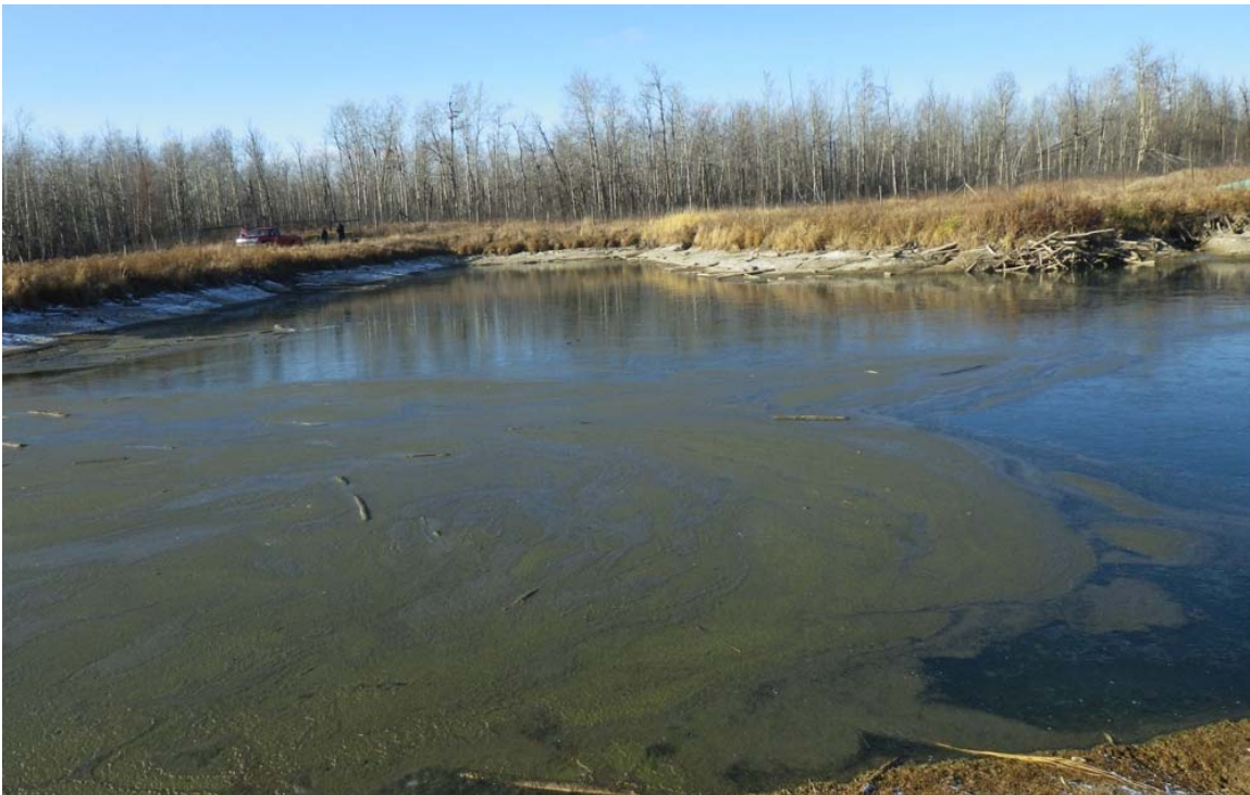
Photograph 8: Wide-angle view of the Administration Area Sewage Lagoon storage cell, facing north from south berm. The small settling cell is located behind the berm to the right.
