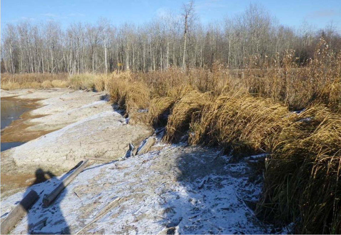
Photograph 11: South berm of Administration Area Sewage Lagoon storage cell, showing areas of slumping. Photo taken facing east.
