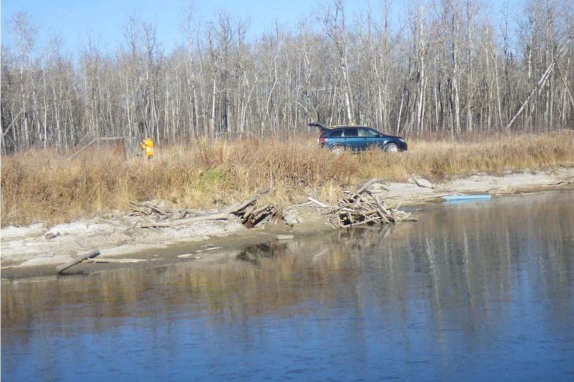
Photograph 13: Storage cell of the Administration Area Sewage Lagoon, facing east. Beaver structures are visible in the berm between the storage cell and the settling cell. The blue pipe discharges water from the settling cell into the storage cell.
