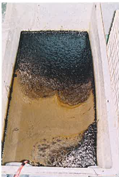
Figure 4 Surface of mixing tank showing the accumulated coalesced bitumen.
