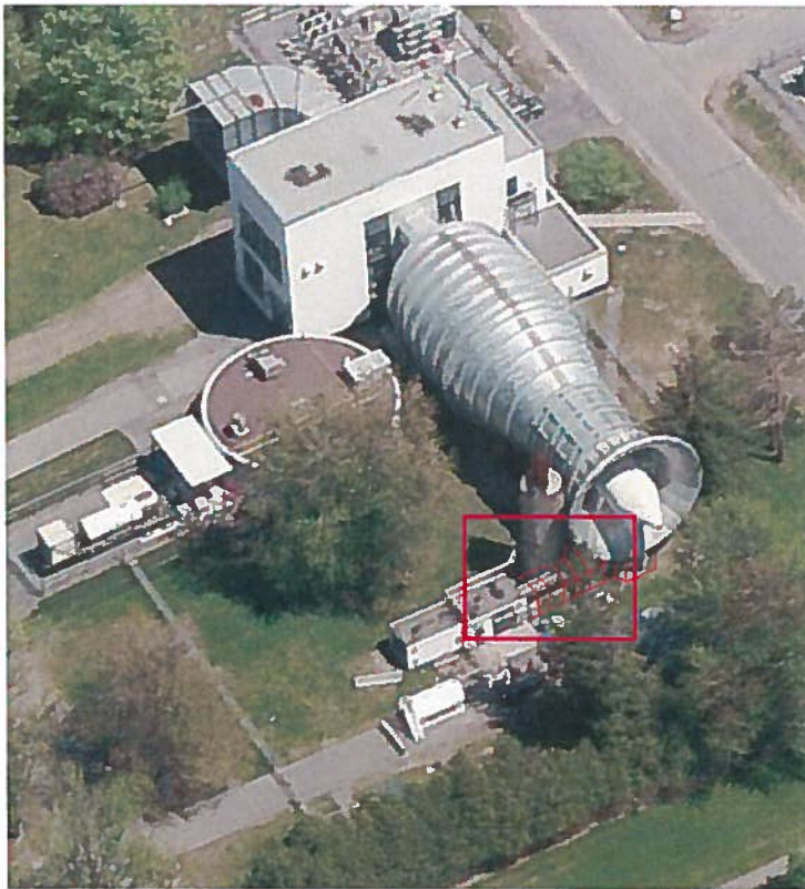
Figure 1 - NRC Propulsion Wind Tunnel – acoustic enclosure illustrated in red.
