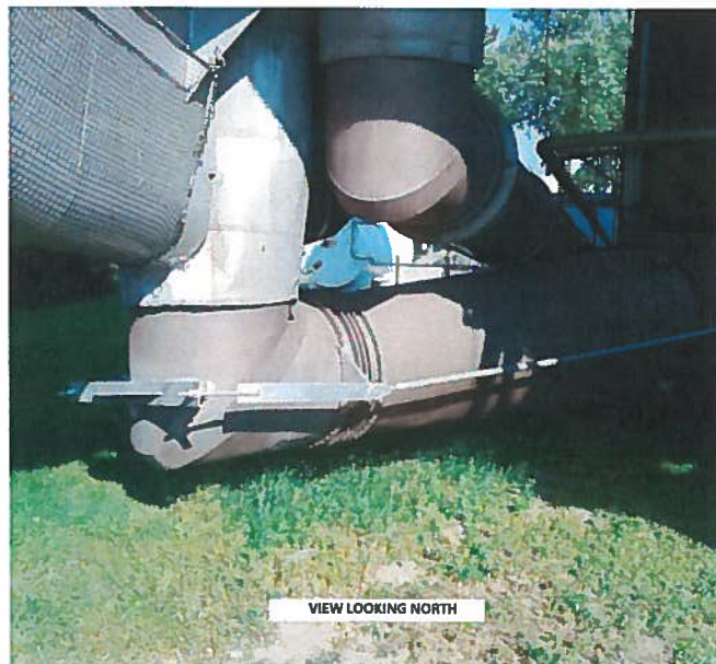
Figure 8. Exhaust Pipework – Looking North.
