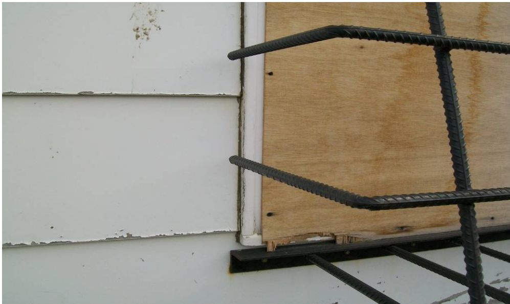
Photograph 8: View of white paint along the exterior window sill along the west side of the building. Paint sample collected contained 800 ppm of lead.
