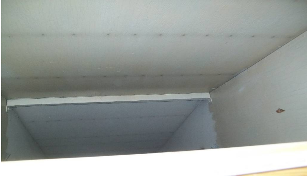
Photograph 7: View of older upper ceiling area of east wing of building. Paint samples collected from yellow paint of older ceiling contained between 7,800 – 64,000 ppm of lead.
