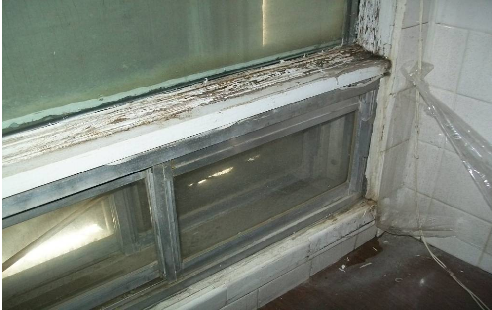
Photograph 3: View of asbestos-containing caulking along window sill of older window in west wing of building. Sample of caulking contained 4% Chrysotile asbestos.
