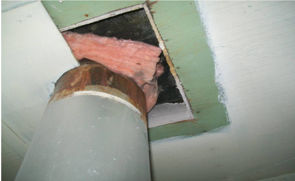
Photograph 5: View of asbestos-containing cement Transite panel along upper ceiling of in east wing of building. Sample of Transite contained 35% Chrysotile asbestos.
