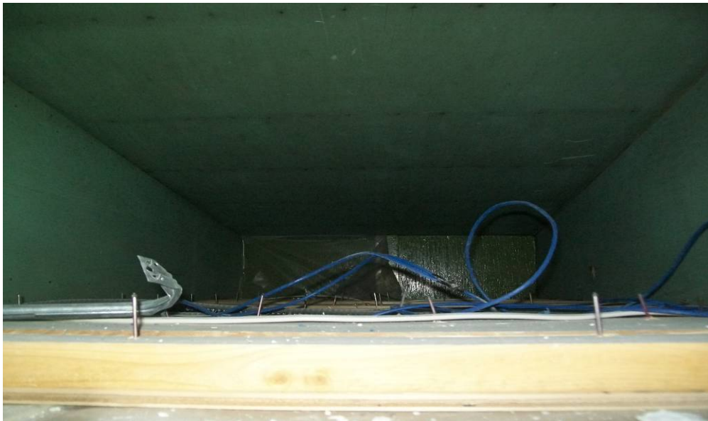
Photograph 6: View of older upper ceiling area of east wing of building. Paint samples collected from green paint of older ceiling contained 110,000 parts per million (ppm) of lead.
