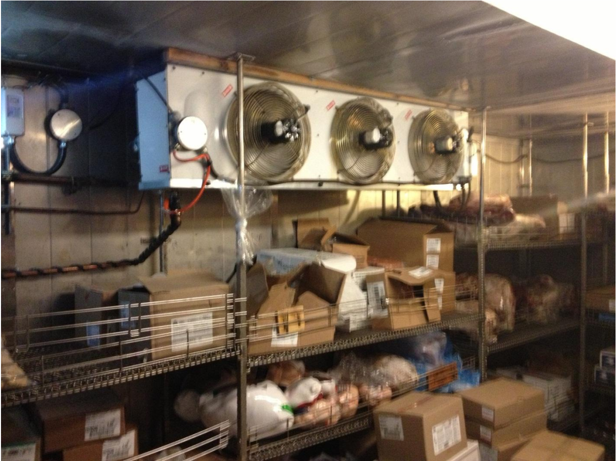
Freezer Room Evaporator Coil (To Remain)
