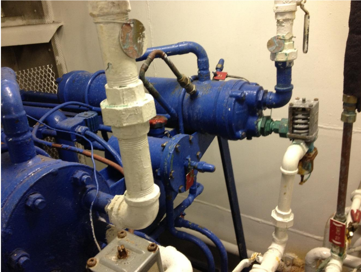
Refrigeration Package (Aft Condenser to be replaced as seen in picture)
