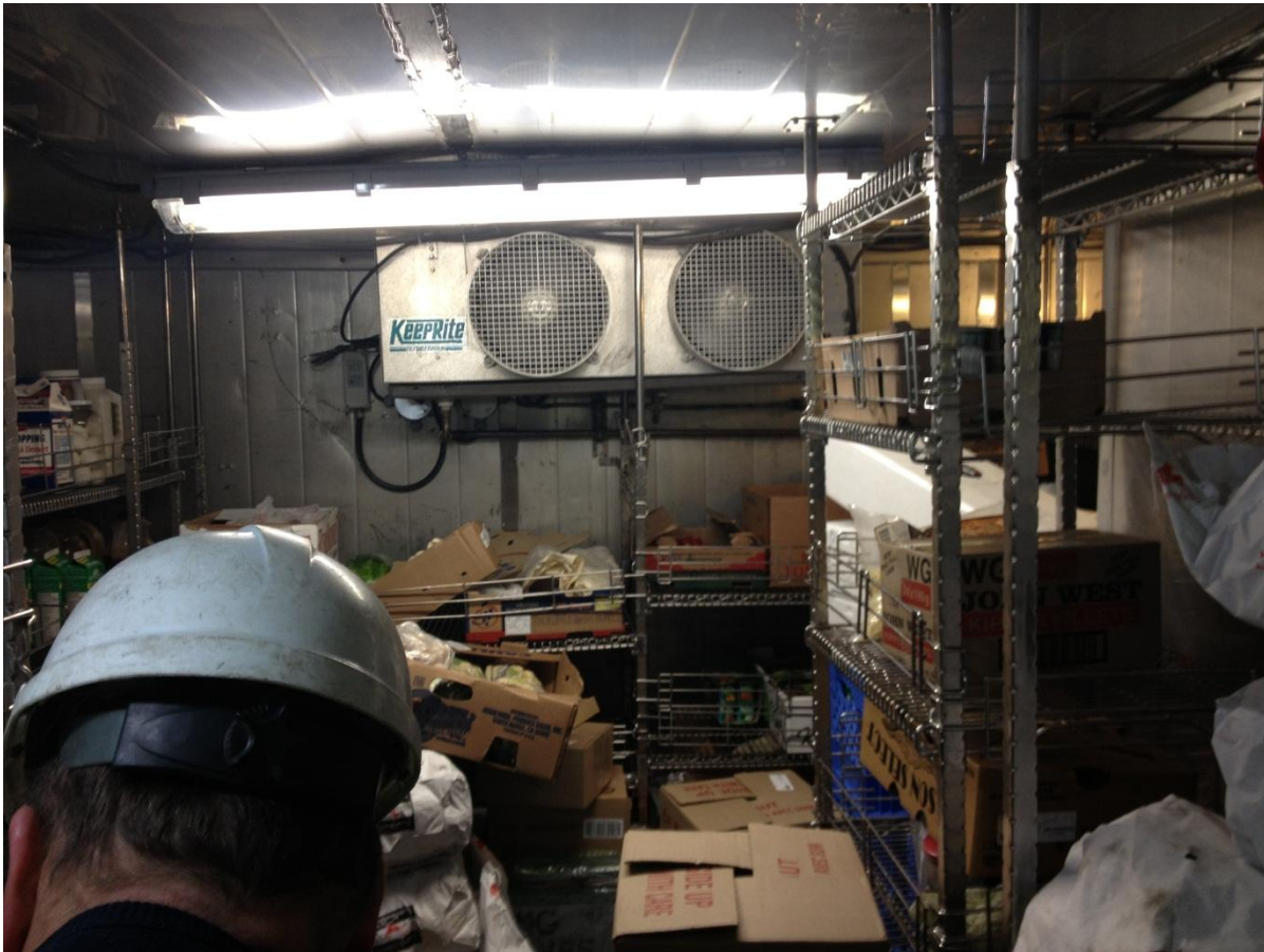
Cooler Room Evaporator Coil (To Remain)
