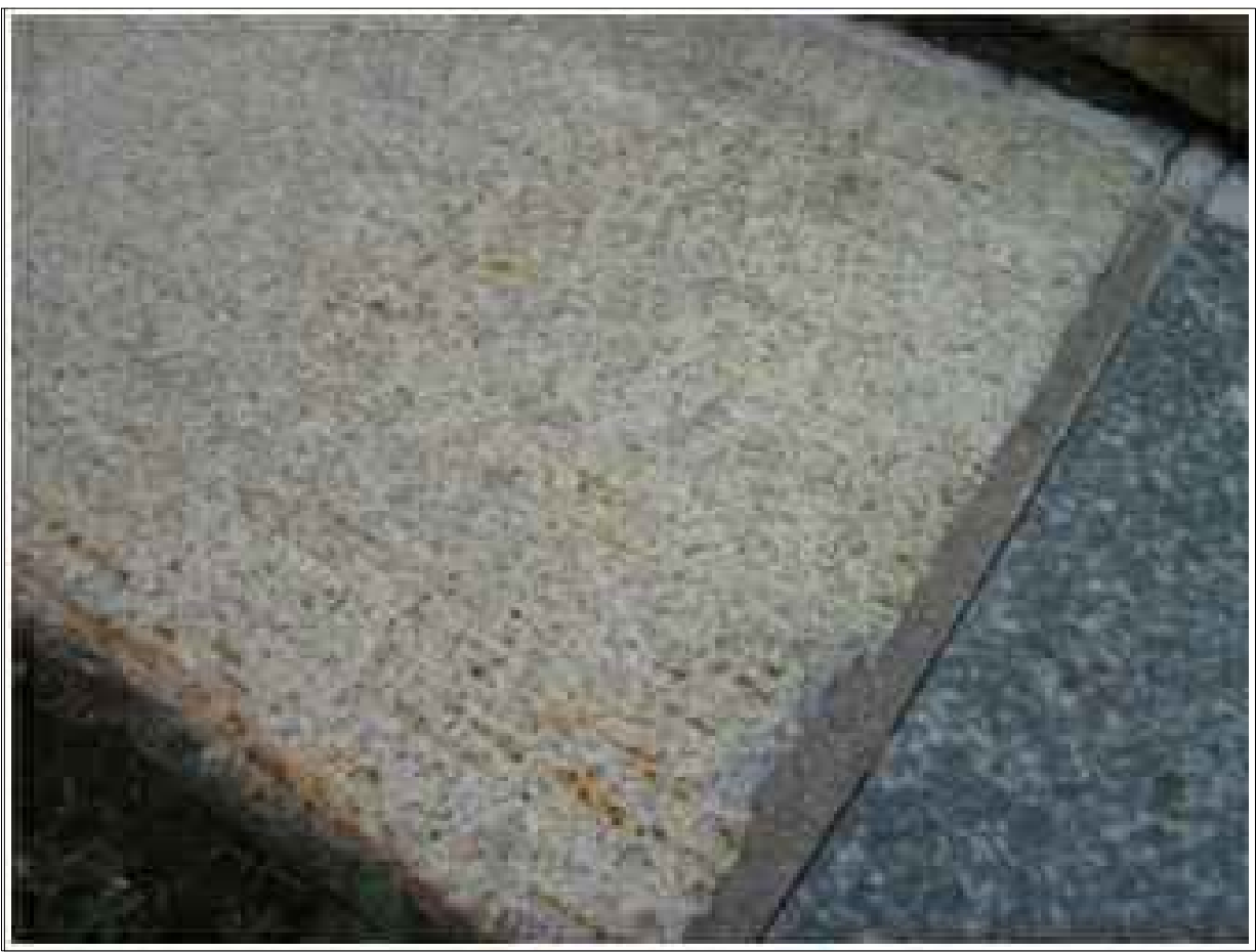
PIERRE NON-ASSORTI - FAILLITE DE JOINT MISMATCHED STONE - FAILED JOINT
