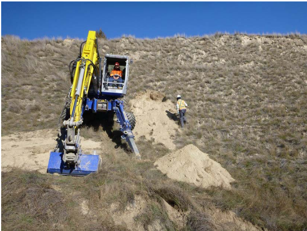
Photo 10: TP3 –Disturbed soil/fill noted to 1 m with native soil below. Minor debris to 1 m.
