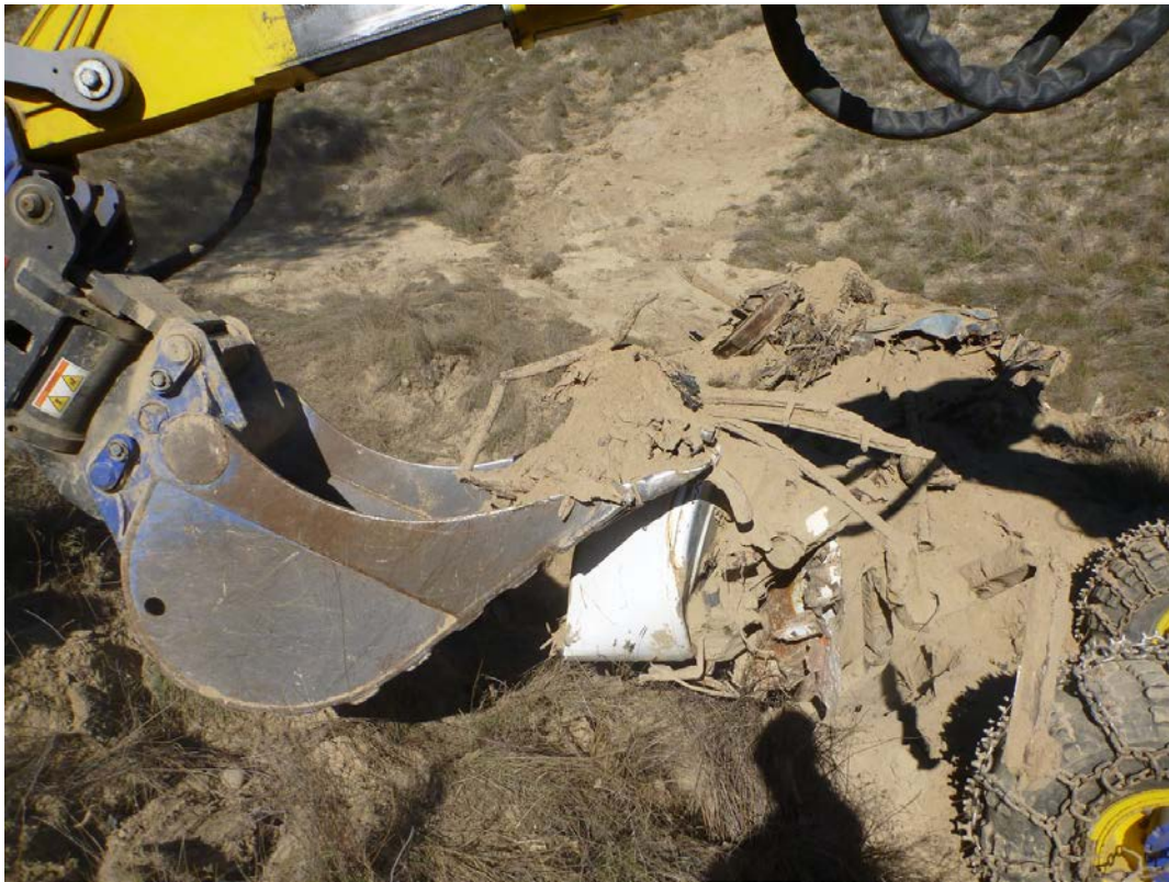
Photo 15: TP7 - Metal debris observed throughout excavation.
