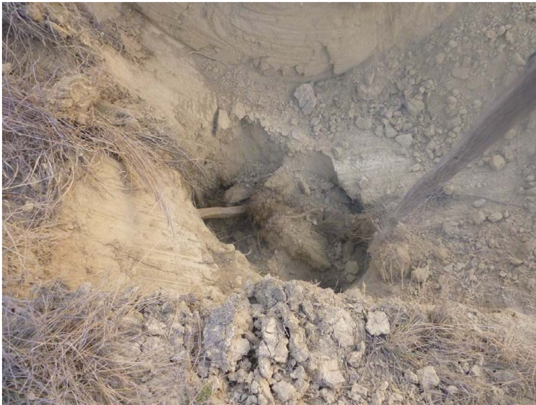
Photo 24: Excavation in area of cavity and water flow – found deep cavity in trail.
