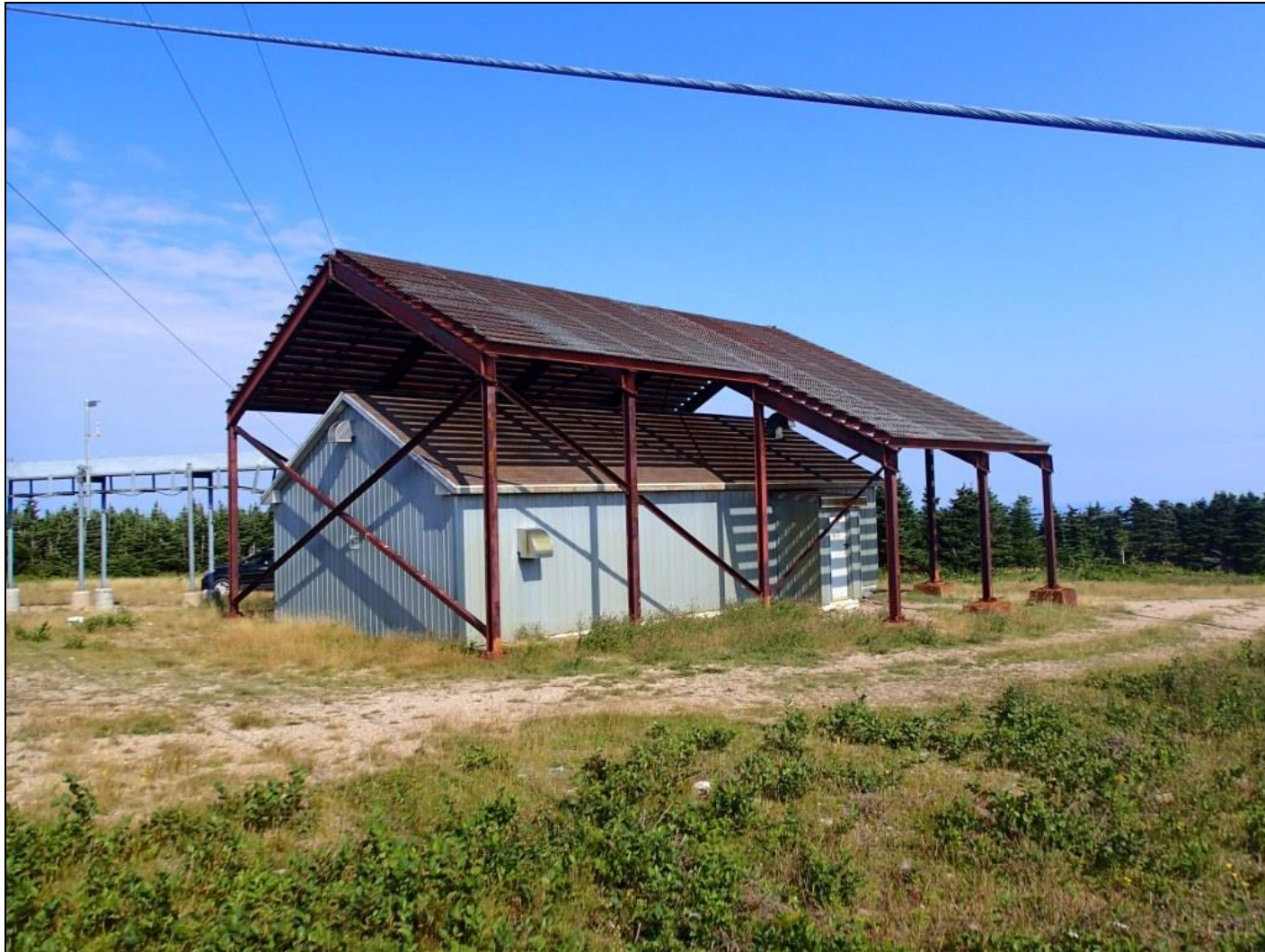
CCG equipment building, ice shelter and waveguide bridge. View from vicinity of eastern guy anchor.
