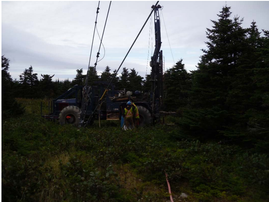
Photo 1: Shows the drill-rig setup at borehole BH-BGC14-01.
