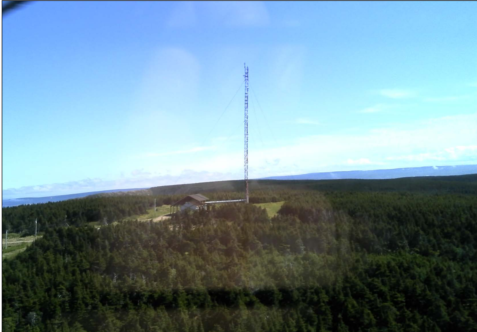
Canadian Coast Guard (CCG) site at Cape North. The equipment building, steel ice shelter over building, waveguide bridge and VHF tower are visible.
