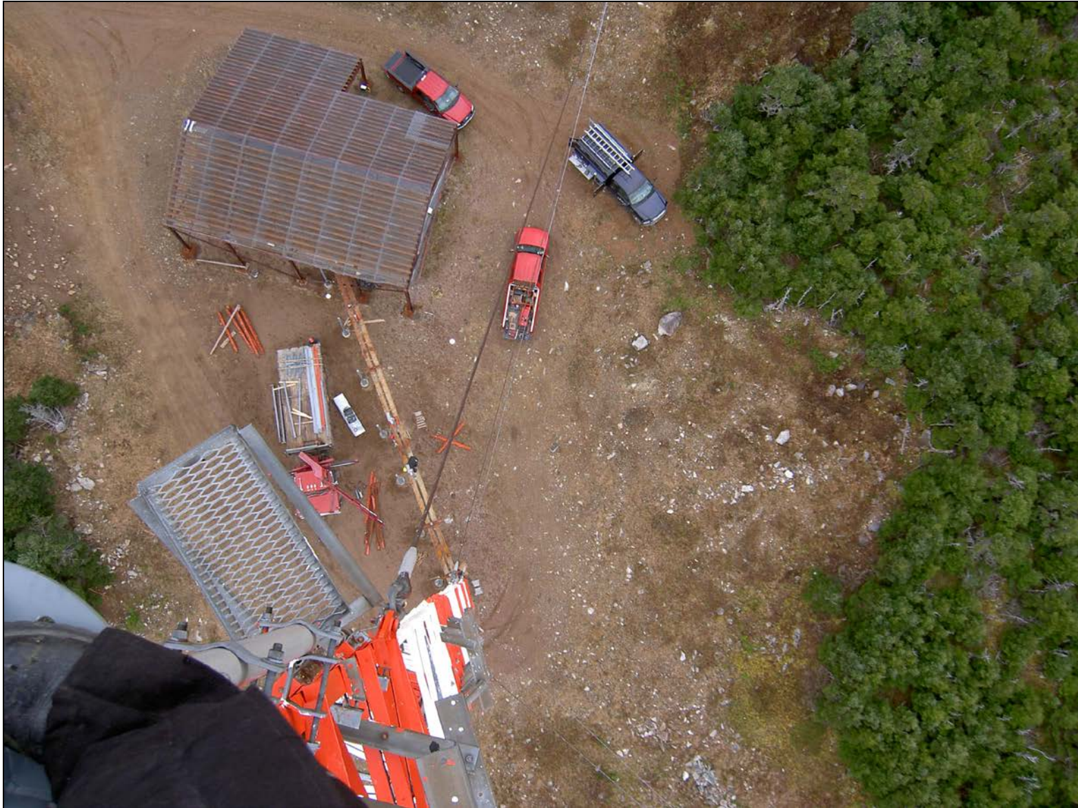
CCG Cape North tower site, viewed from top of existing VHF tower. Older waveguide bridge and ice shelter visible on ground.
