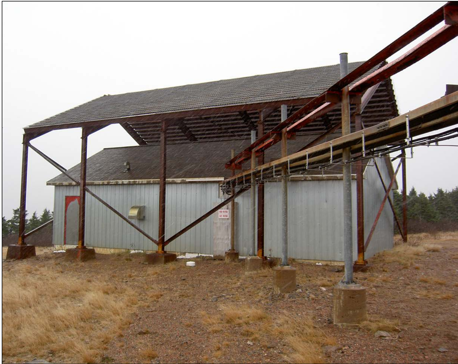
Older waveguide bridge (replaced) and western side of CCG equipment building.
