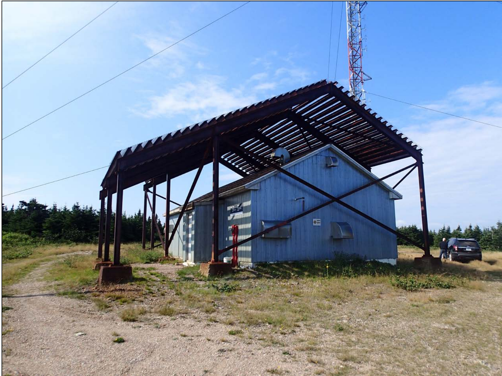
CCG equipment building and steel ice shelter in foreground. VHF tower visible behind building.
