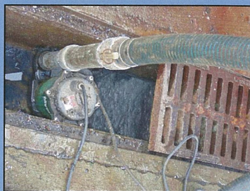
Example of a pump set up used to collect wash water on the NLW.
