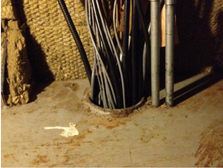
Photo 50.4 Existing cable way between the electronics room and the Bridge crawl space.
