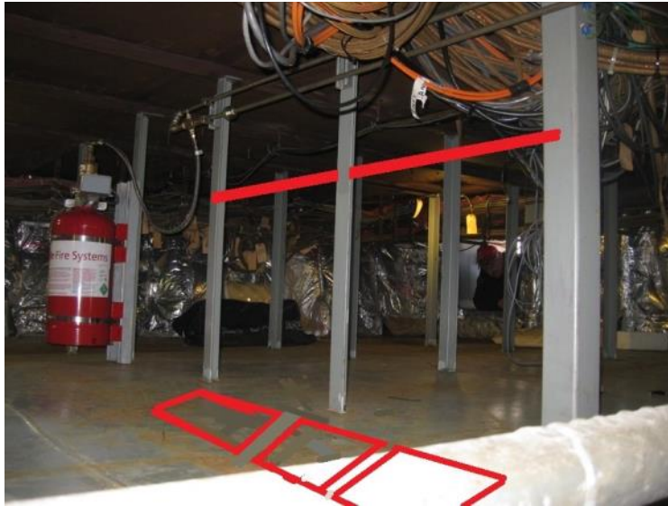
Photo 50-2 Suggested location of transformer bases and horizontal support bracket in the crawl space under the bridge deck. View is looking to starboard, aft to forward.
