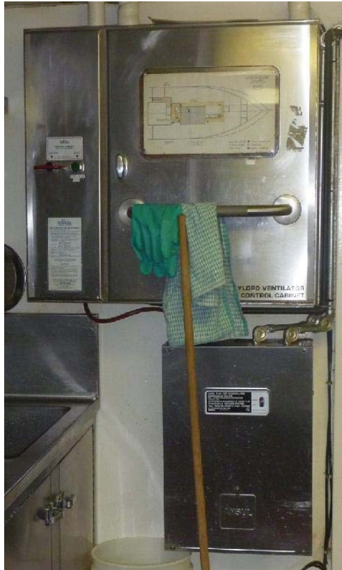
34.3.2.2.12 Exhaust hood control cabinet and fire suppression system
