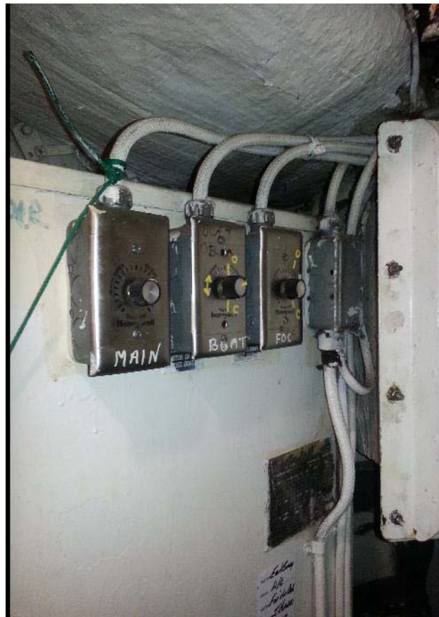
Image 36.1 – Damper Control Switches
