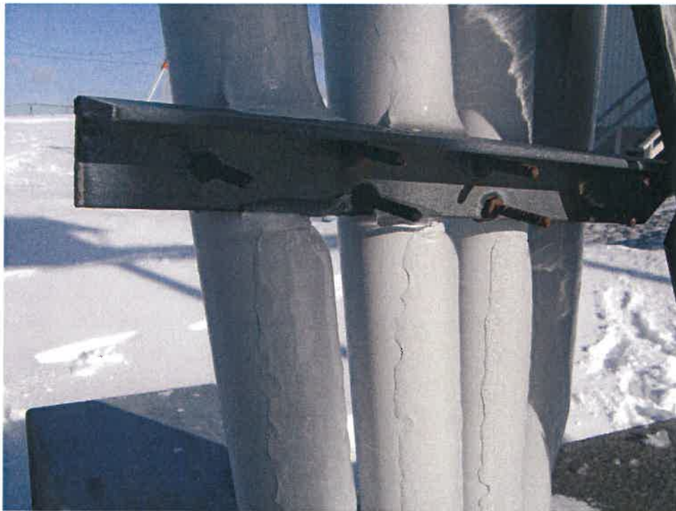
Photo #27: Corroded Hardware
