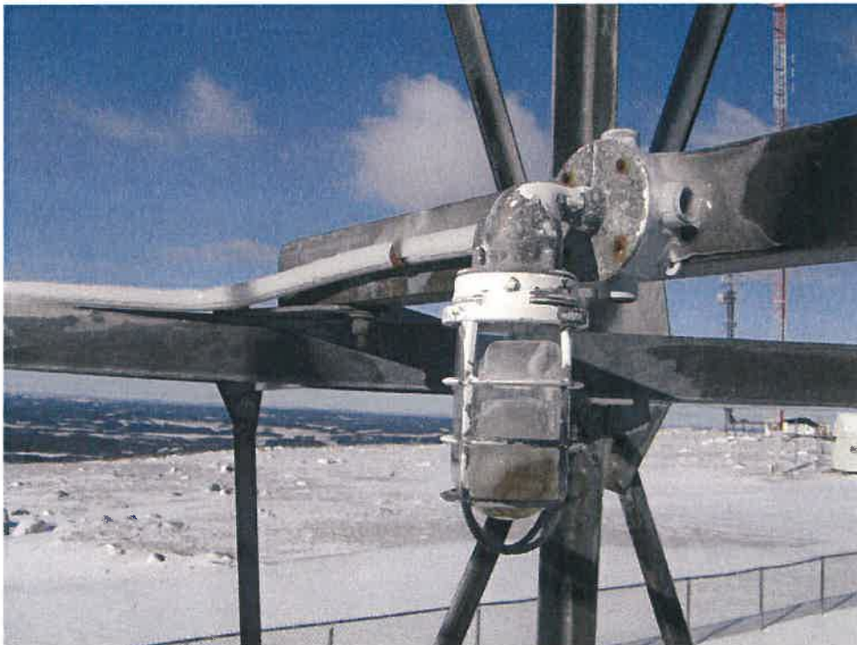
Photo #13: Access Lighting on Tower
