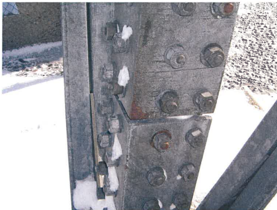
Photo #22: Surface Corrosion on Bolts Typical Throughout
