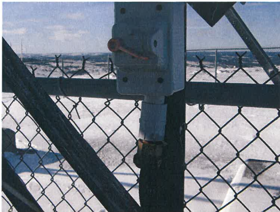
Photo #20: Corroded Electrical Connection
