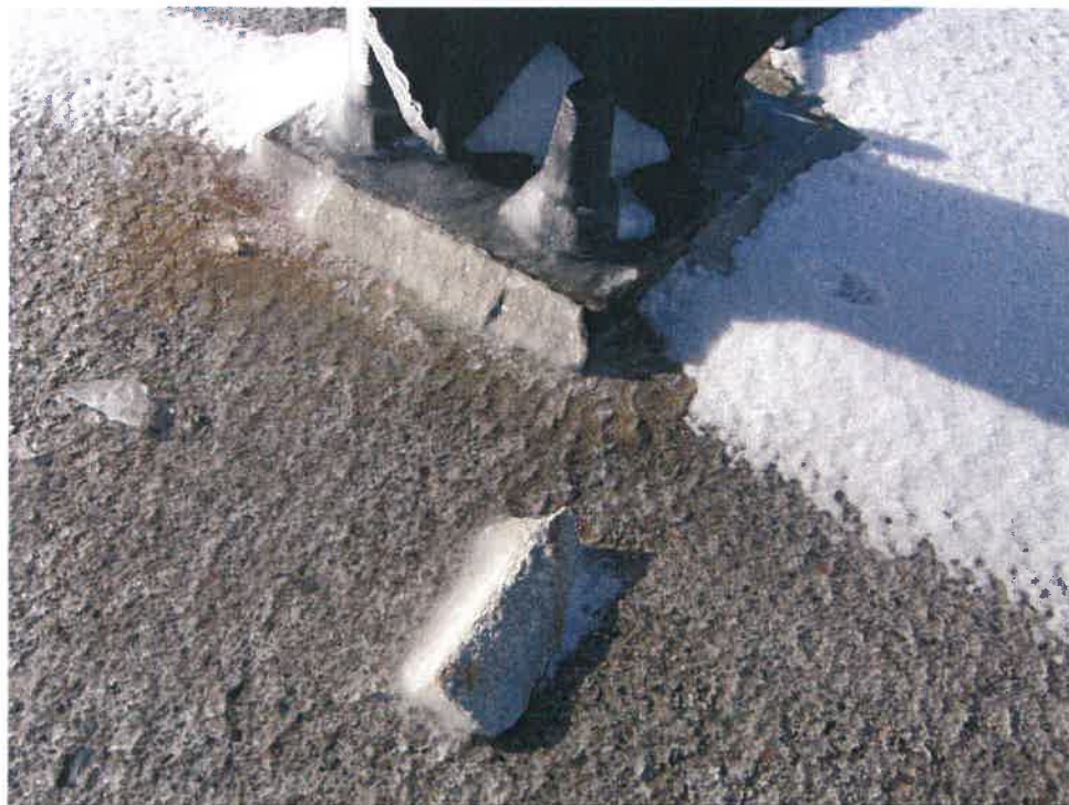
Photo #17: Damaged Grout
