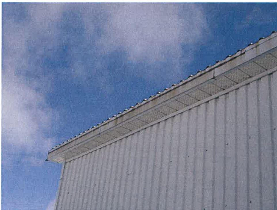
Photo #23: Surface Corrosion on Eave of Building
