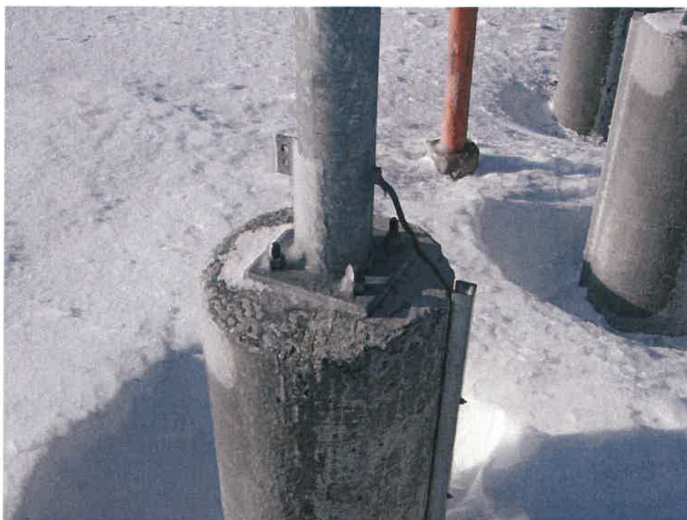
Photo #7: Waveguide Post Grounding Typical
