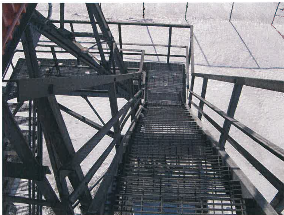
Photo #5: Integral Stairs and Platforms
