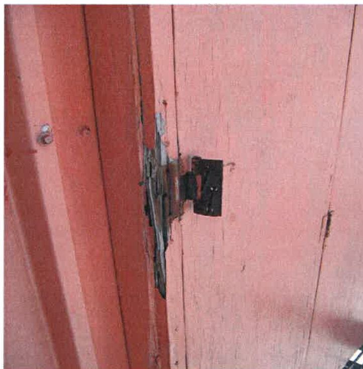
Photo #21: Damaged Door Frame
