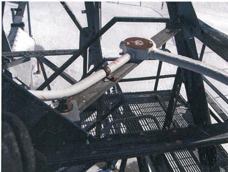
Photo #29: Corroded Electrical Box
