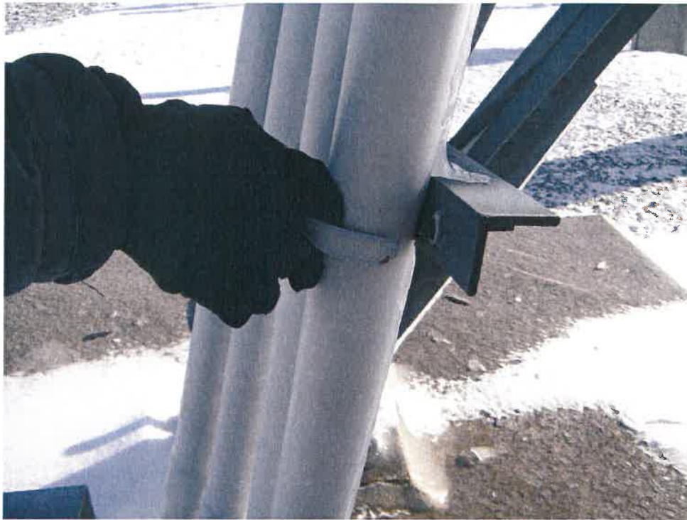
Photo #28: Broken Bracket
