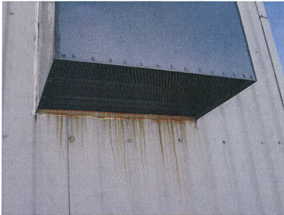
Photo #24: Surface Corrosion from Building Vent
