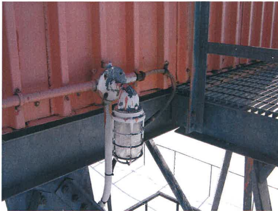
Photo #30: Corroded Electrical Connectors
