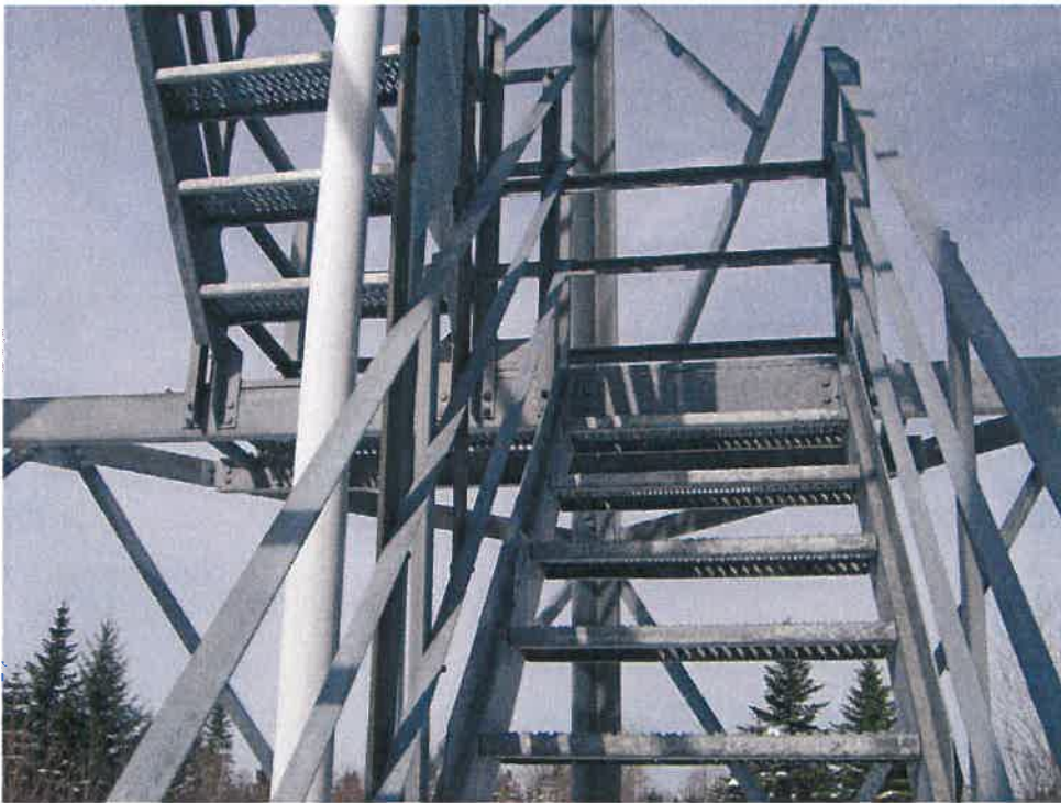
Photo #5: Integral Stairs and Platforms
