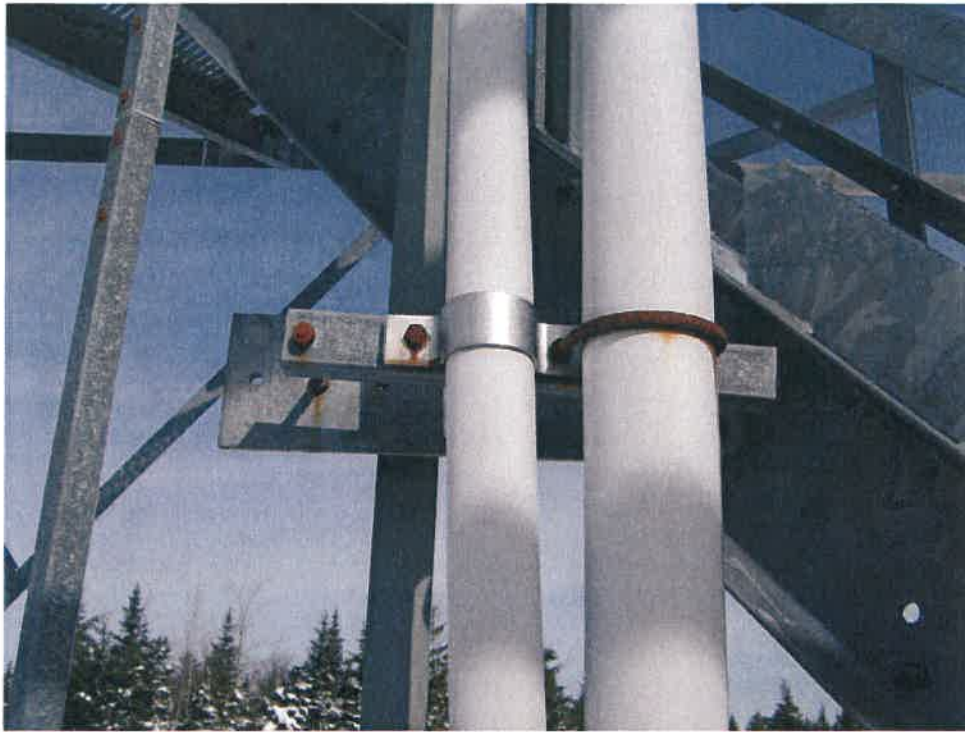
Photo #20: Corroded Electrical Supports
