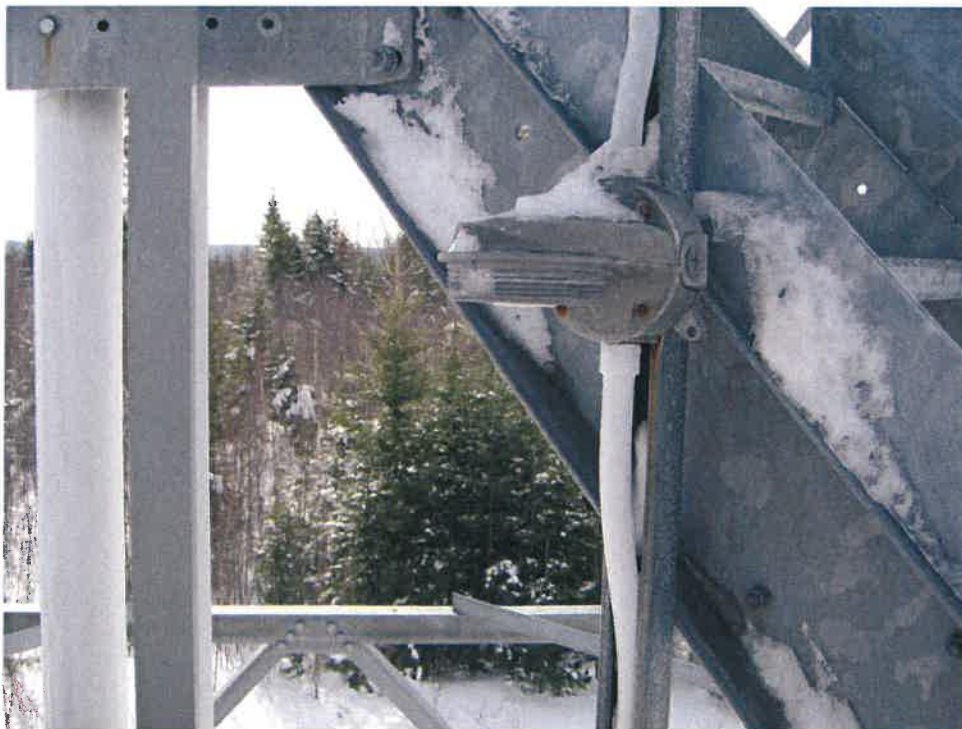
Photo #11: Damaged Access Lighting Level Two
