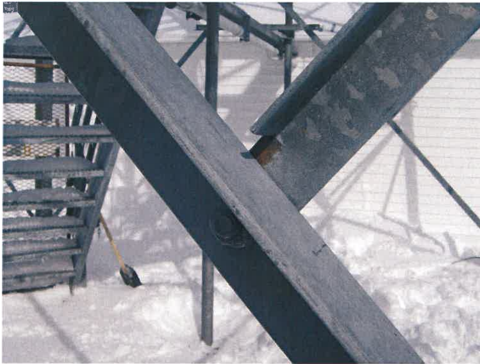
Photo #14: Surface Corrosion Typical Lower Level
