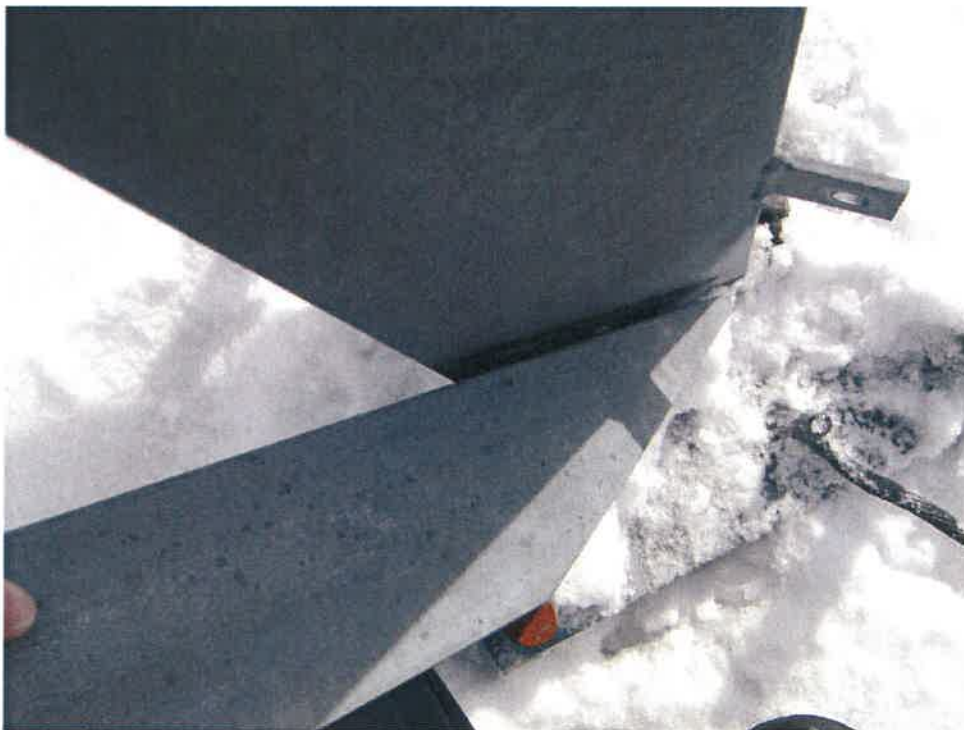
Photo #23: Loose Diagonal Bolts
