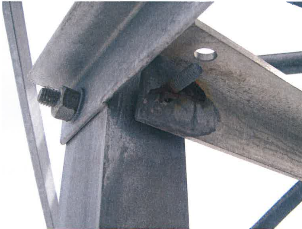
Photo #24: Corroded Cotter Pins
