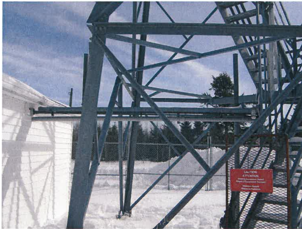
Photo #6: Waveguide Bridge
