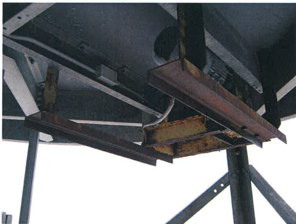
Photo #19: Surface Corrosion on Winch Support
