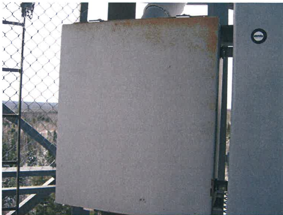
Photo #18: Surface Corrosion on Control Box
