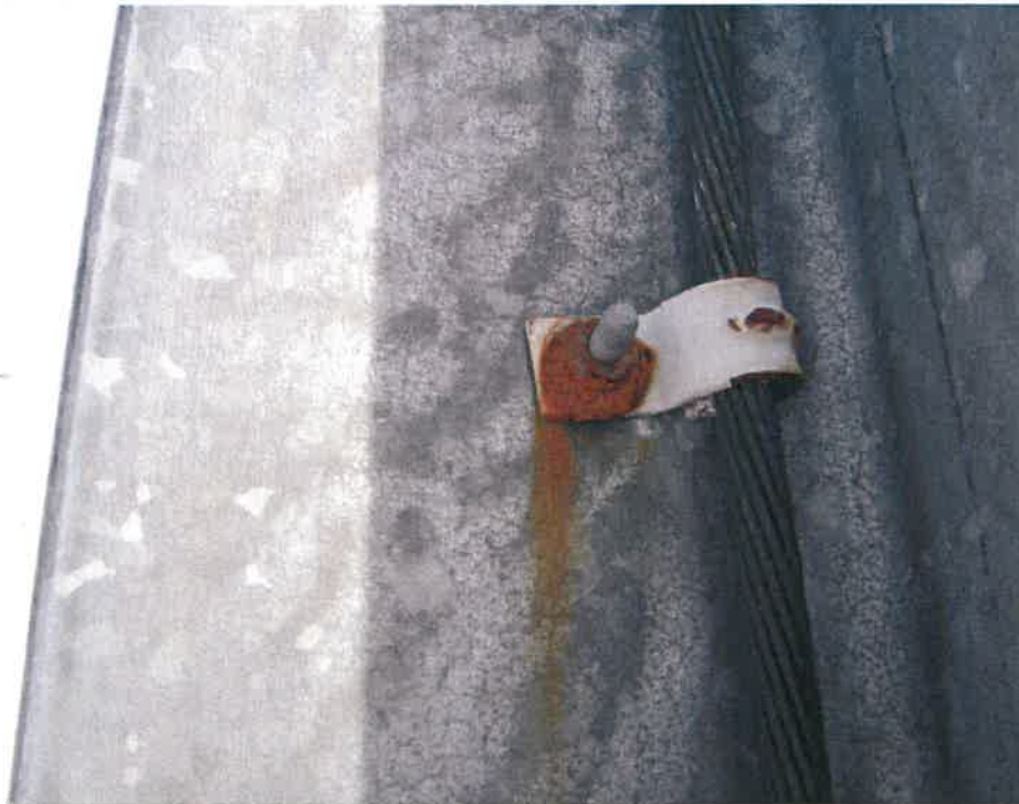
Photo #17: Surface Corrosion on Ground Lead Clips
