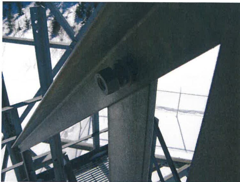
Photo #16: Loose Bolt "Tighten by Tiller"
