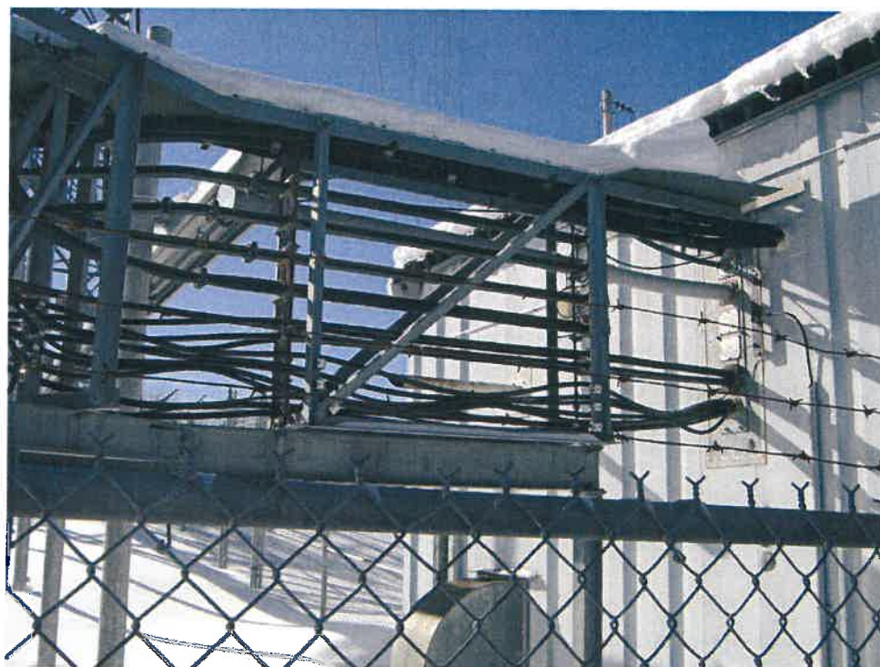
Photo #7: Waveguide Bridge 2
