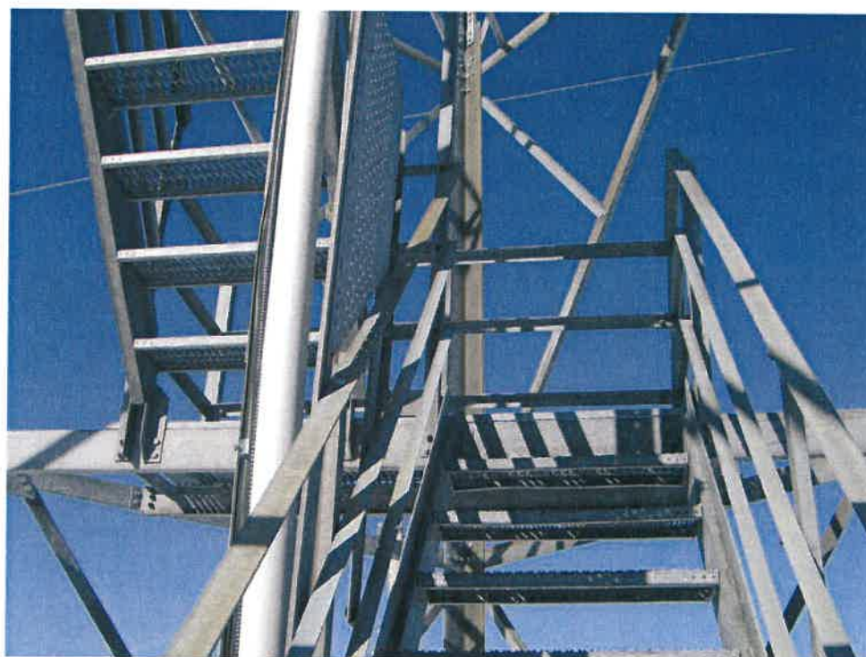
Photo #5: Integral Stairs and Platforms
