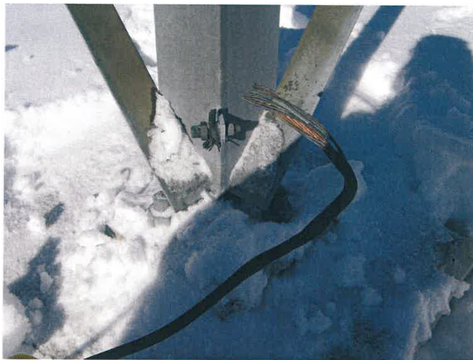
Photo #14: Broken Leg Grounding
