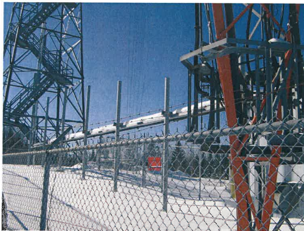
Photo #6: Waveguide Bridge
