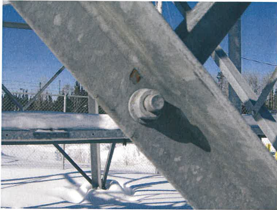
Photo #18: Damaged Diagonal Face 1-2 @ 6 Feet
