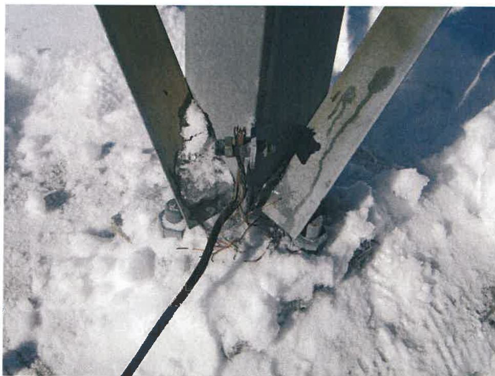
Photo #15: Repaired Leg Grounding
