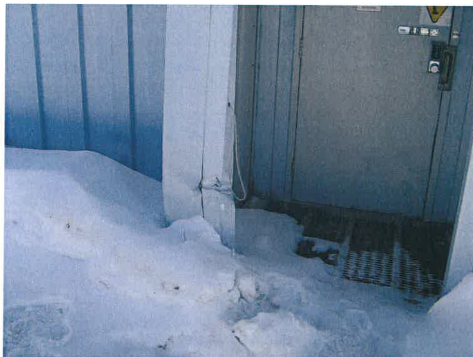
Photo #13: Damaged Wind Break
