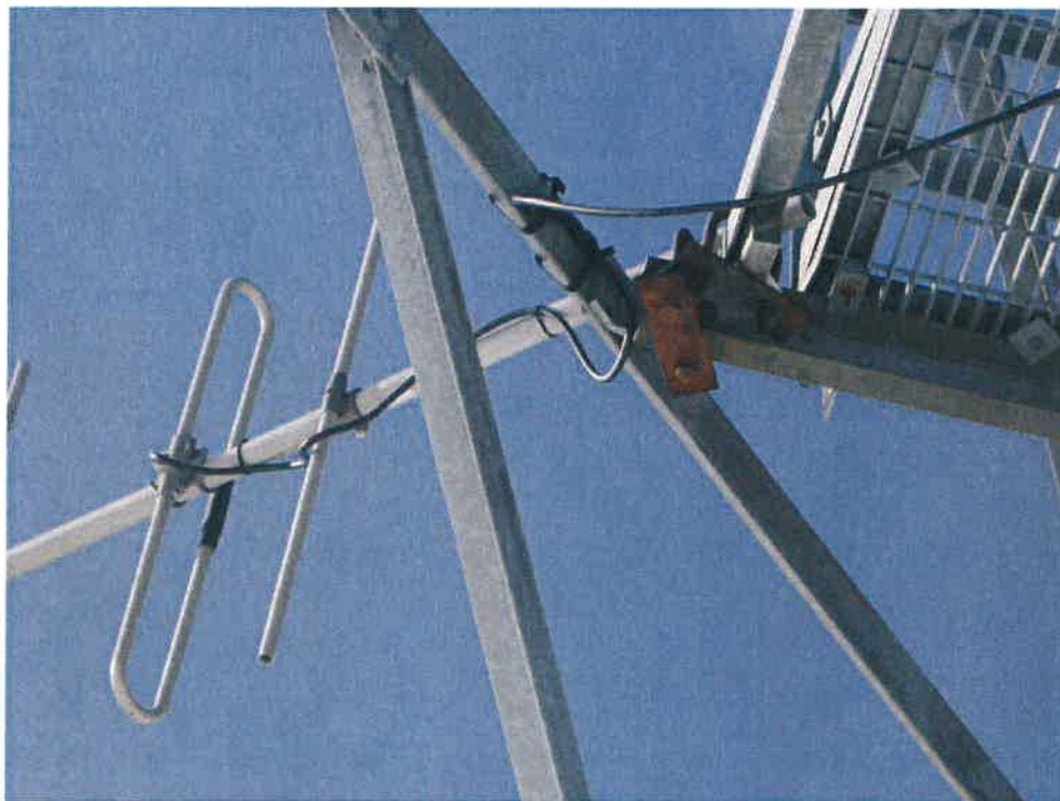
Photo #20: Corroded Antenna Mount
