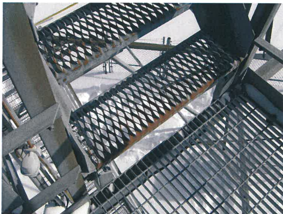
Photo #11: Corroded Steps
