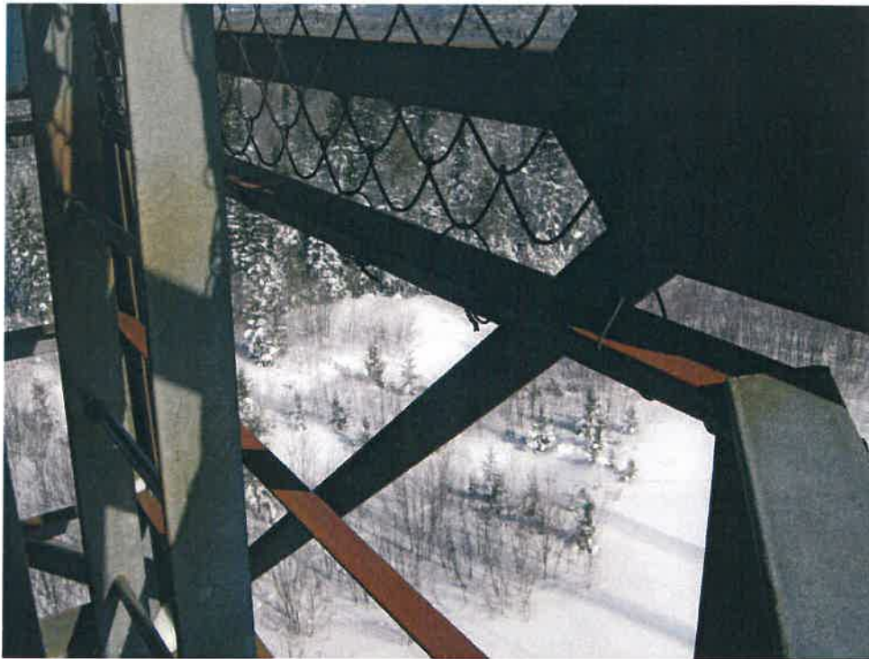
Photo #14: Corroded Tower Members
