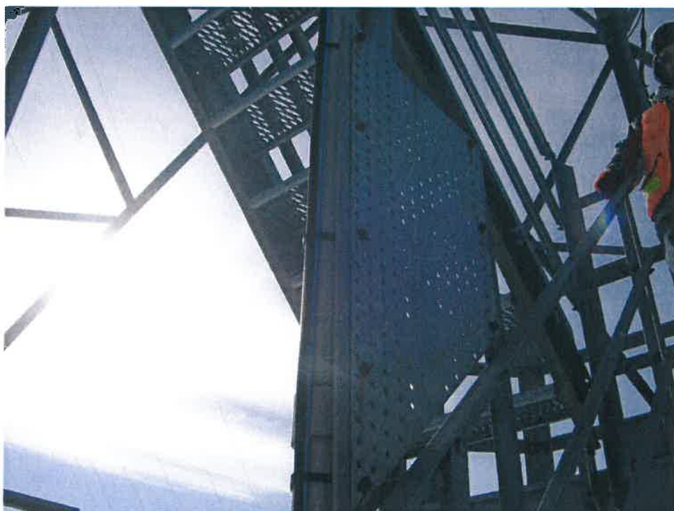
Photo #18: Corroded Plate Bolts
