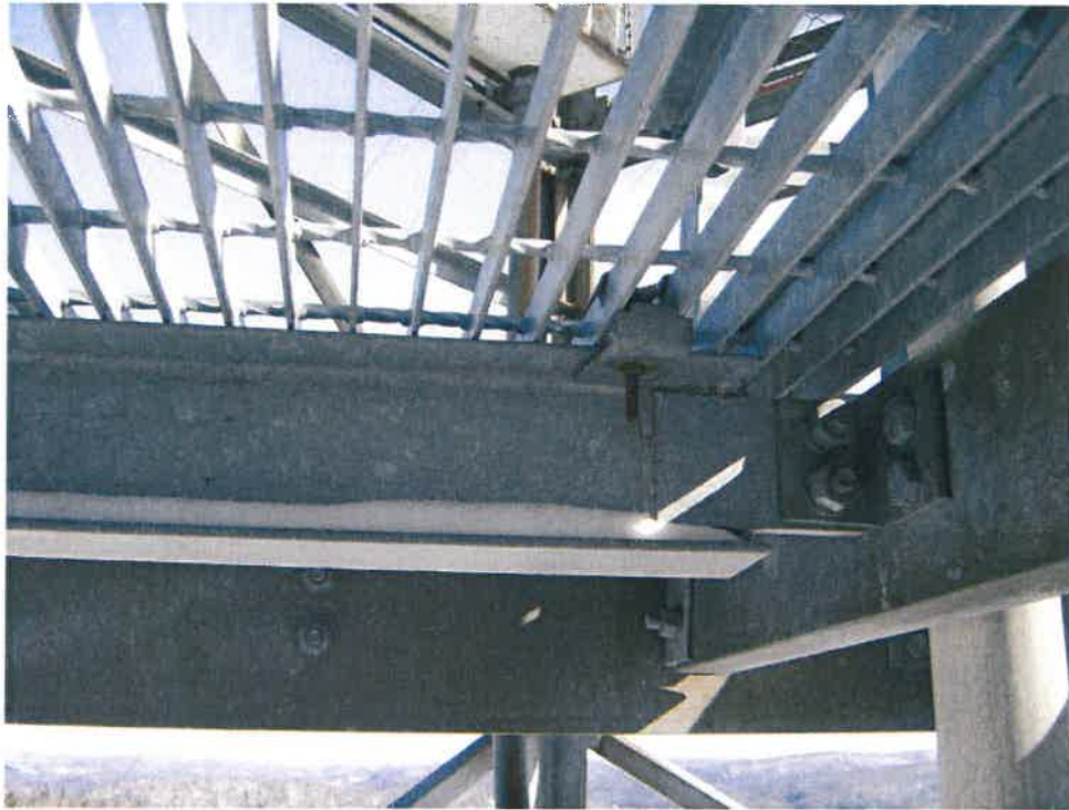
Photo #19: Corroded Grating Bolts
