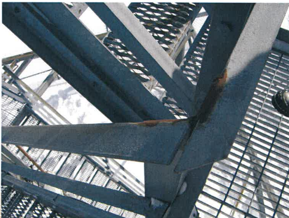
Photo #14: Corroded Tower Members
