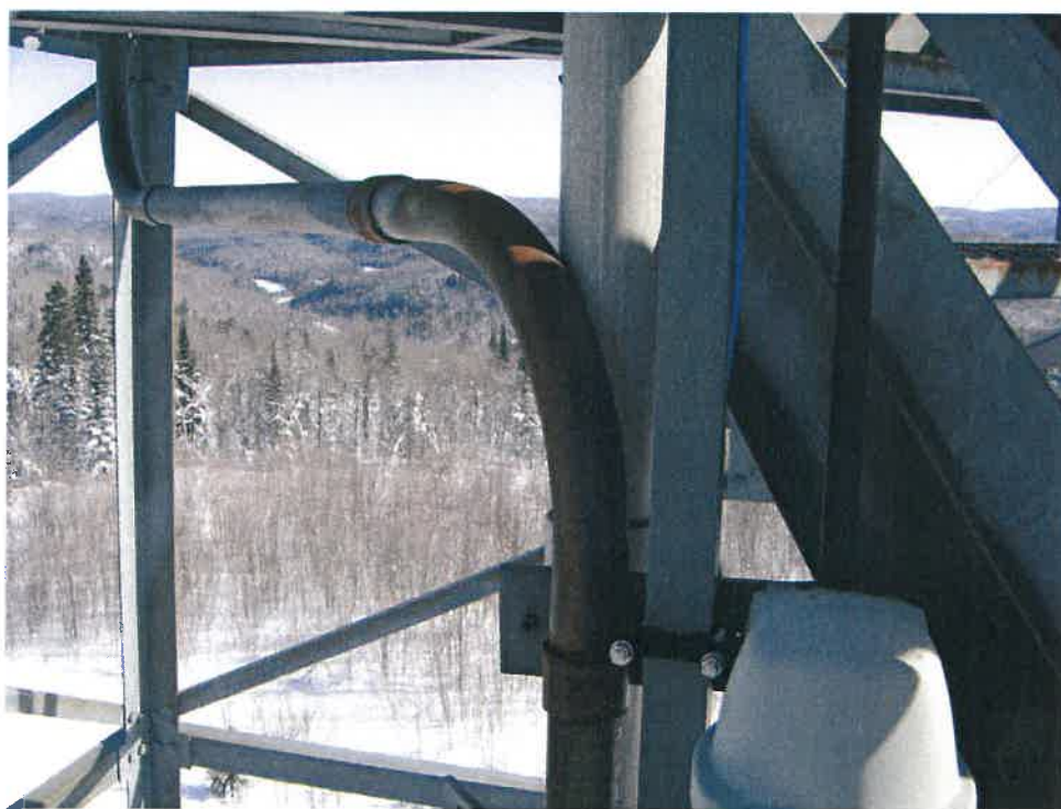
Photo #9: Corroded Electrical Conduit
