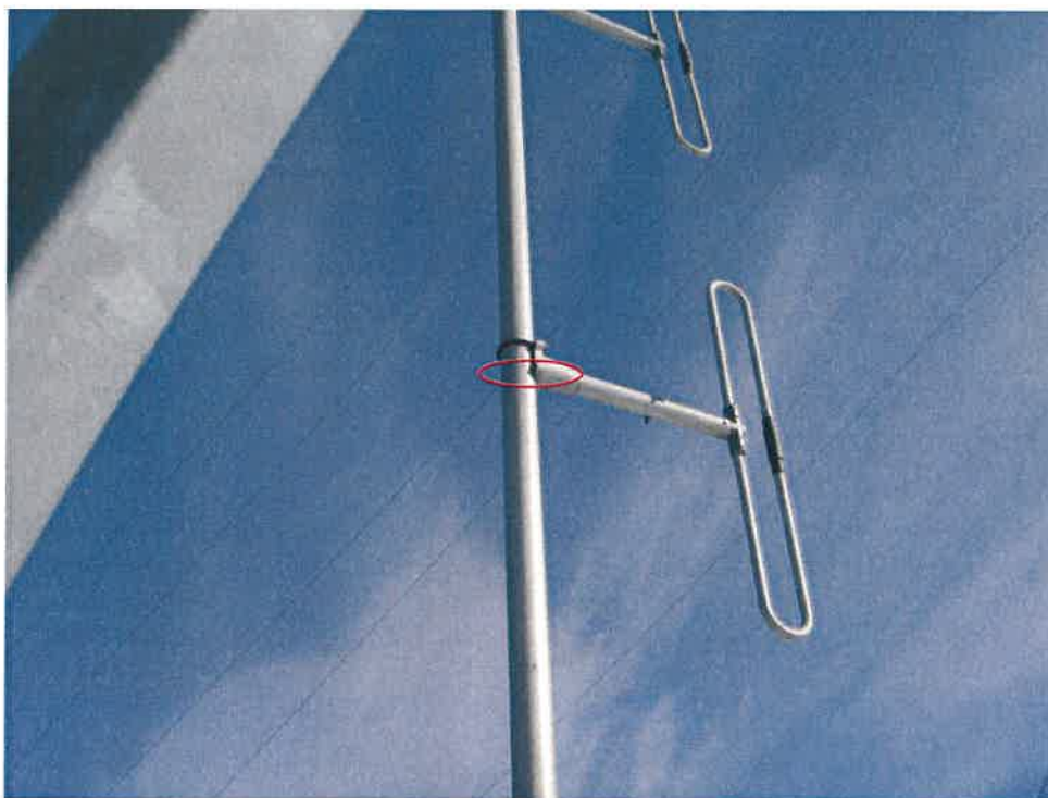
Photo #17: Missing U-Bolt
