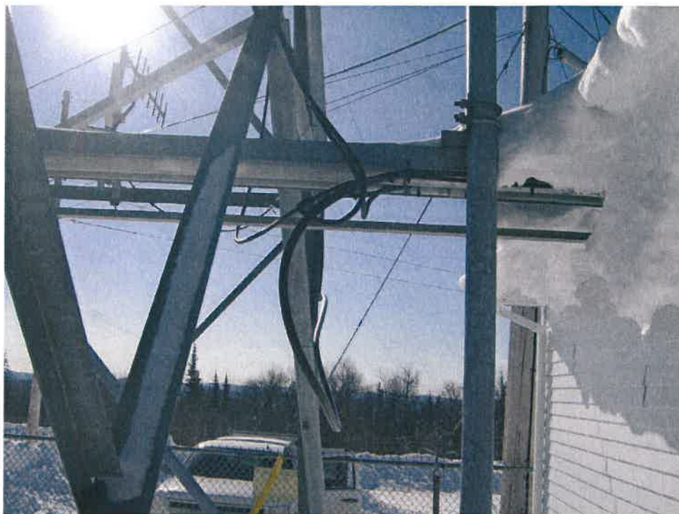
Photo #15: Un-secured TX Lines
