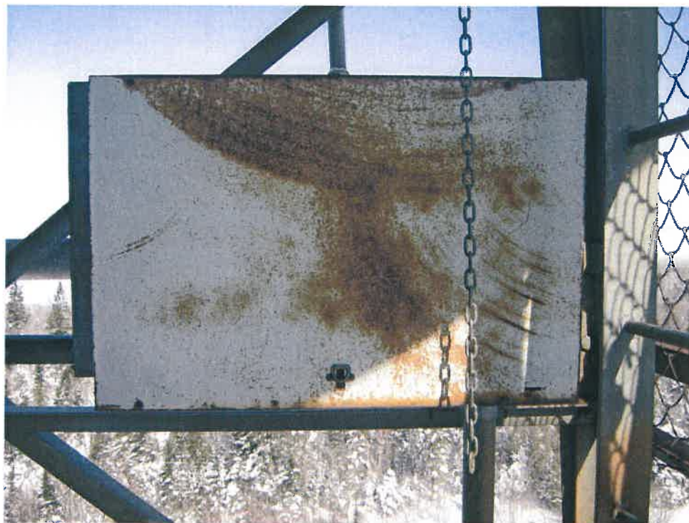
Photo #10: Corroded Electrical Control Box
