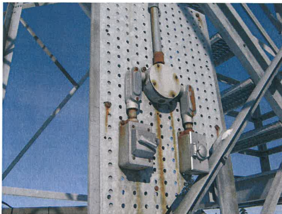
Photo #8: Corroded Electrical Components
