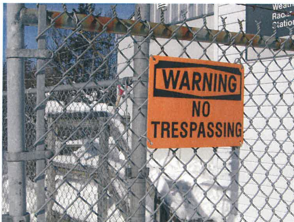
Photo #13: Corroded Fencing Components #2
