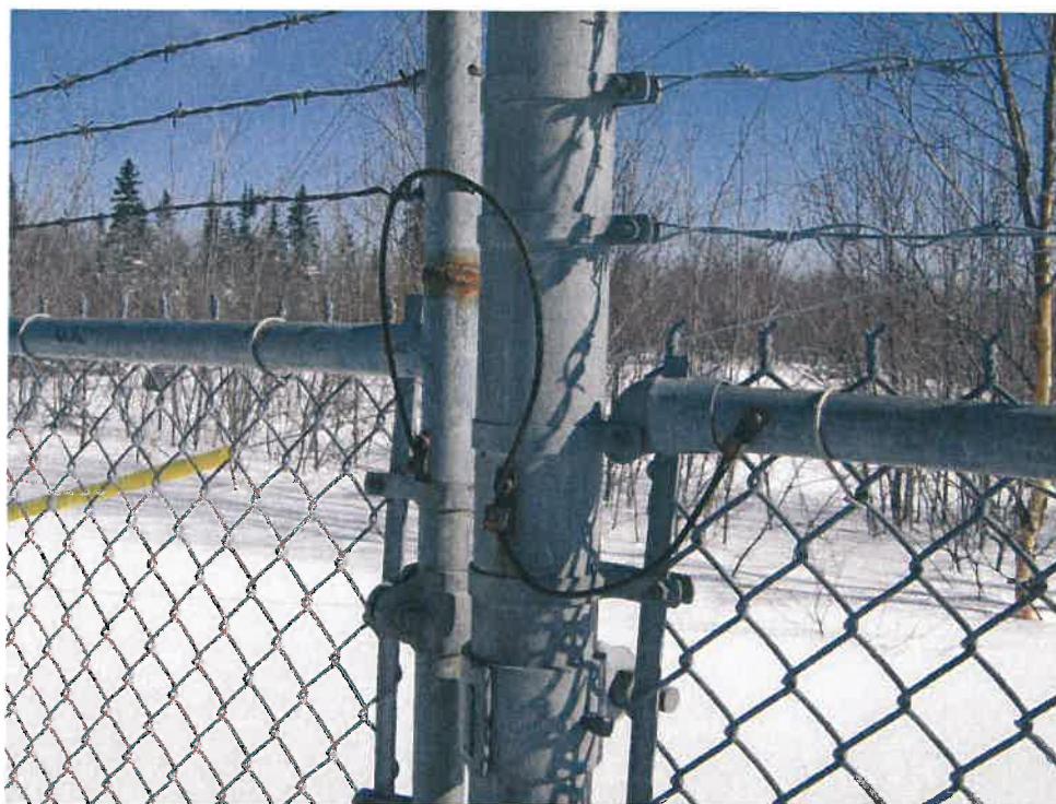
Photo #12: Corroded Fencing Components
