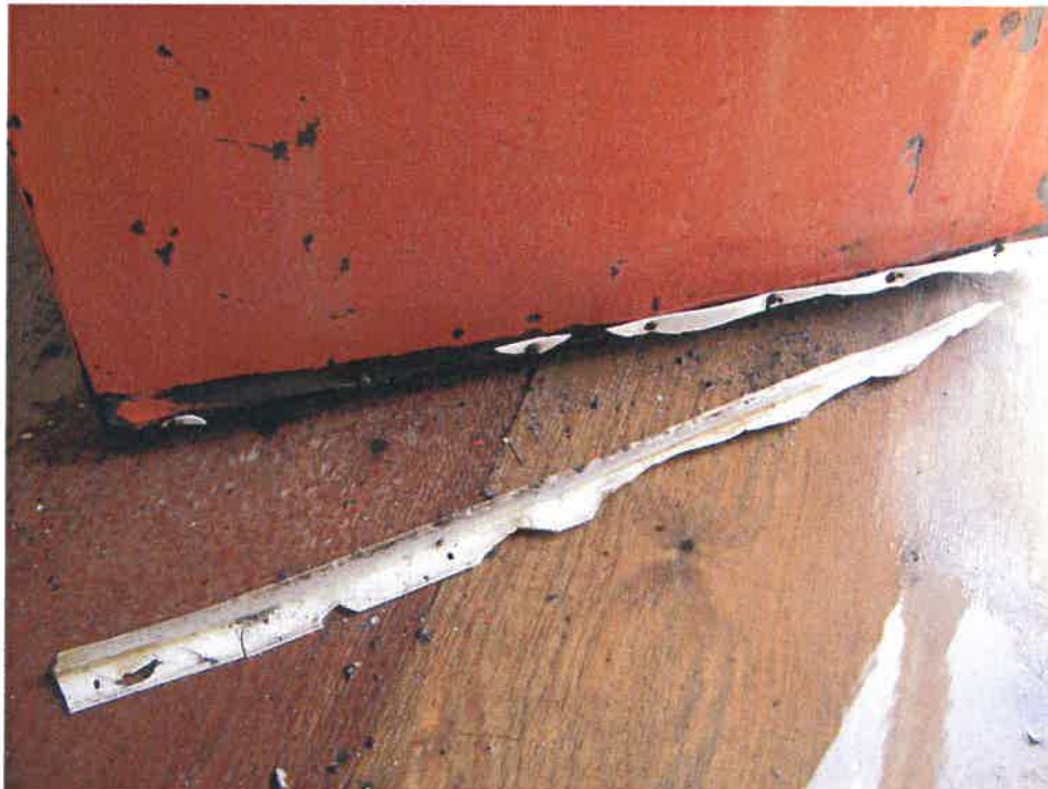
Photo #21: Damaged Door Sweep
