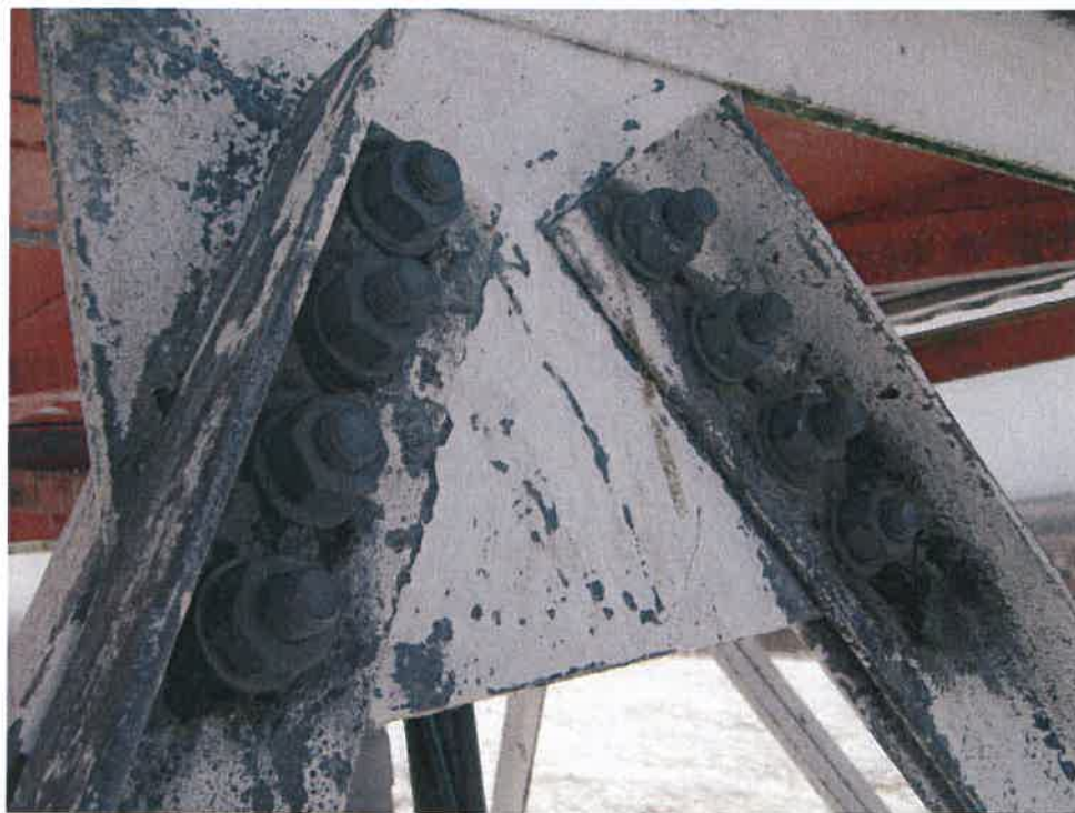
Photo #27: Burned Holes in Diagonals
