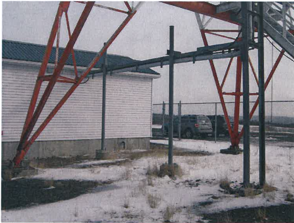
Photo #6: Waveguide Bridge
