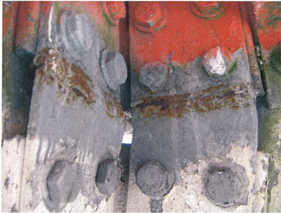
Photo #18: Surface Corrosion Typical 4 Locations
