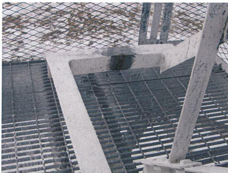
Photo #23: Surface Corrosion on Hand Rail
