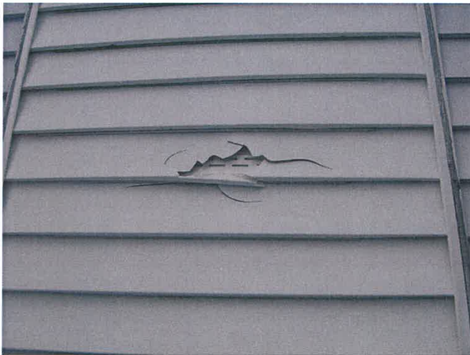
Photo #29: Damaged Siding
