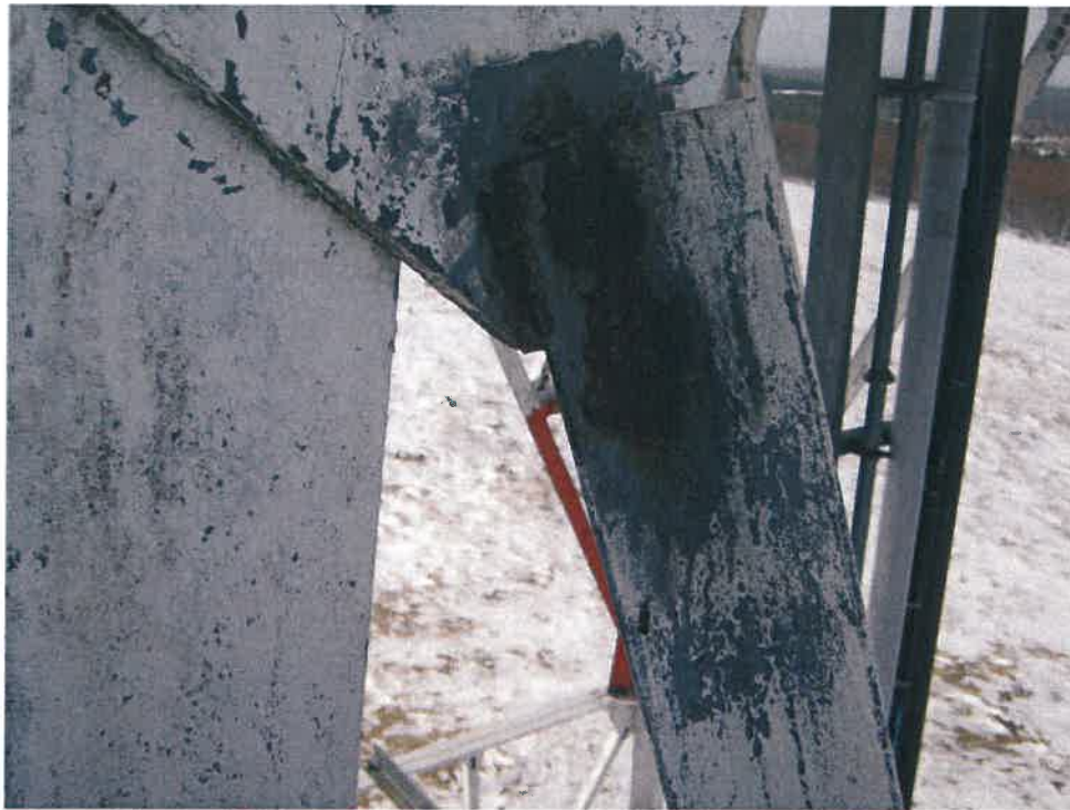
Photo #24: Surface Corrosion on Welded Diagonal
