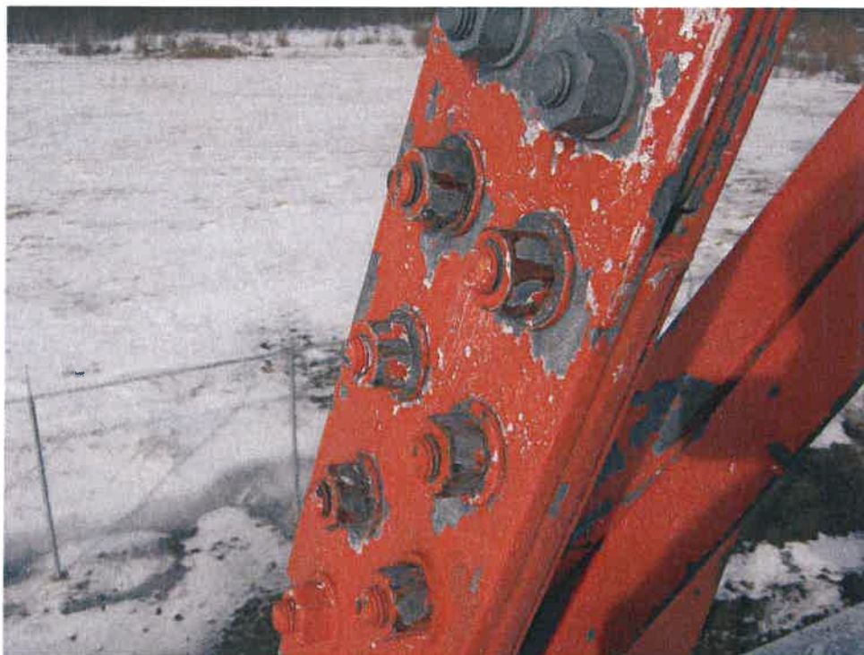
Photo #22: Surface Corrosion on Bolts Typical
