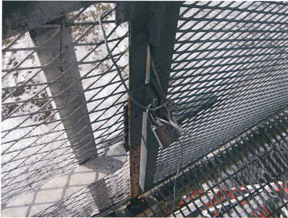
Photo #20: Corroded Rail Connection
