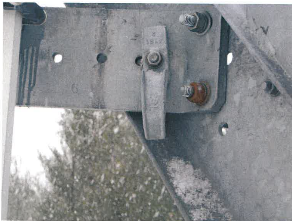
Photo #11: Corroded Nut
