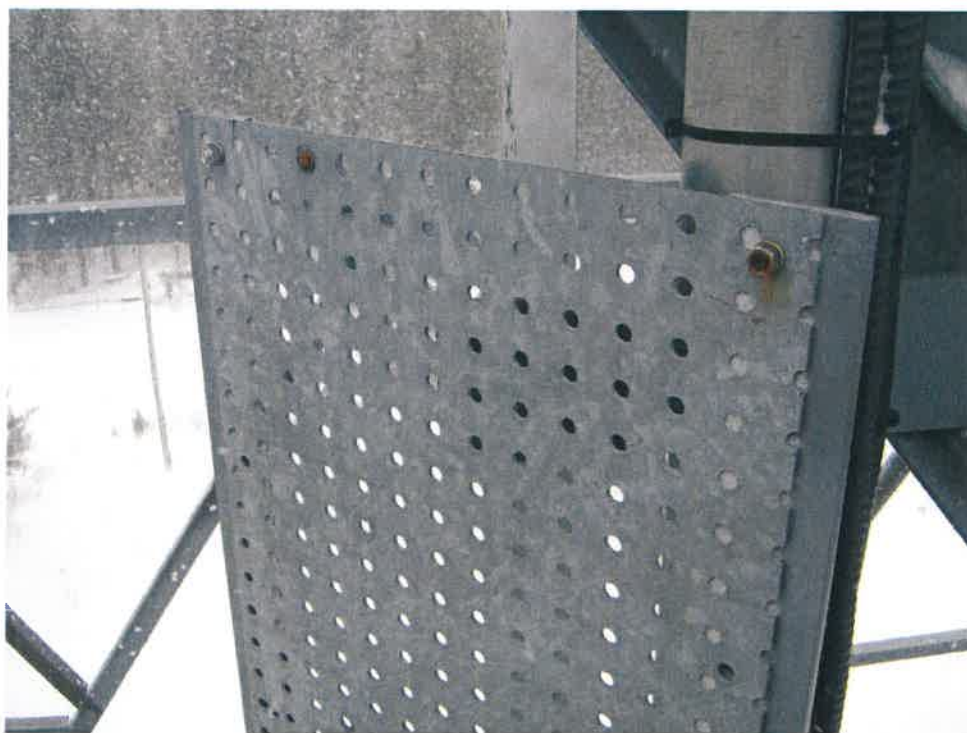
Photo #17: Corroded Bolts
