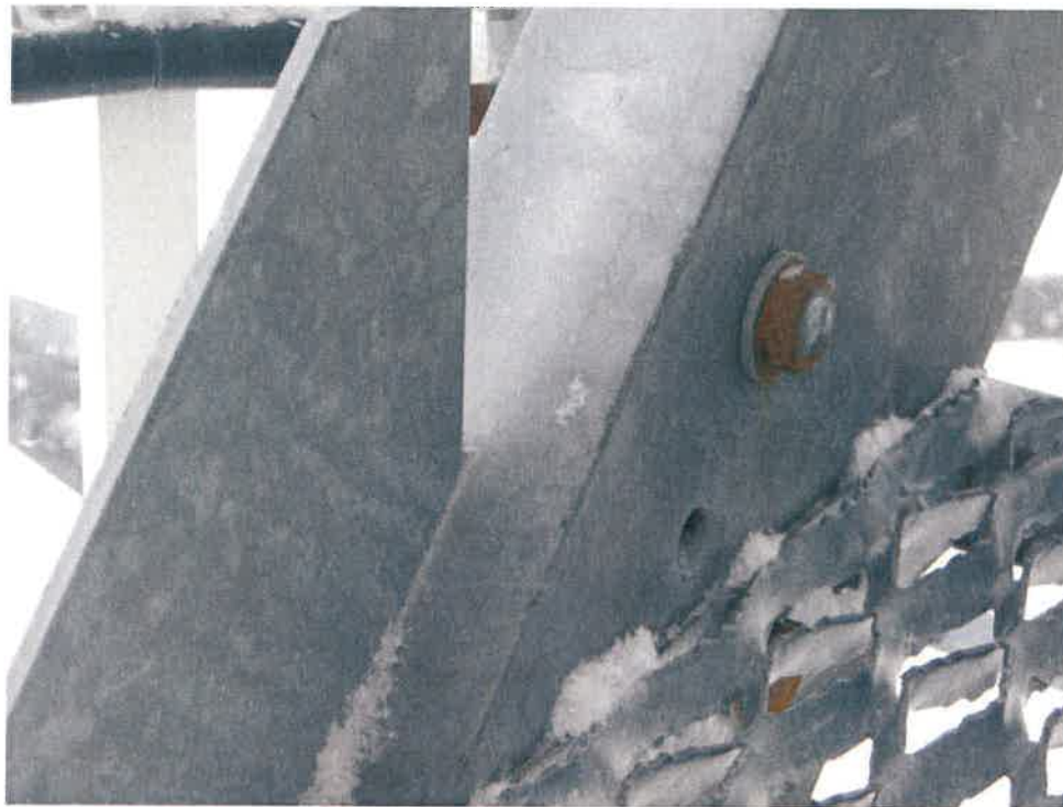
Photo #12: Corroded Bolt In Stairs
