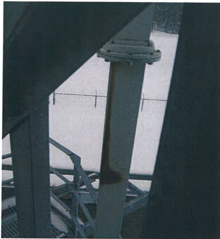
Photo #18: Corroded Hard Line
