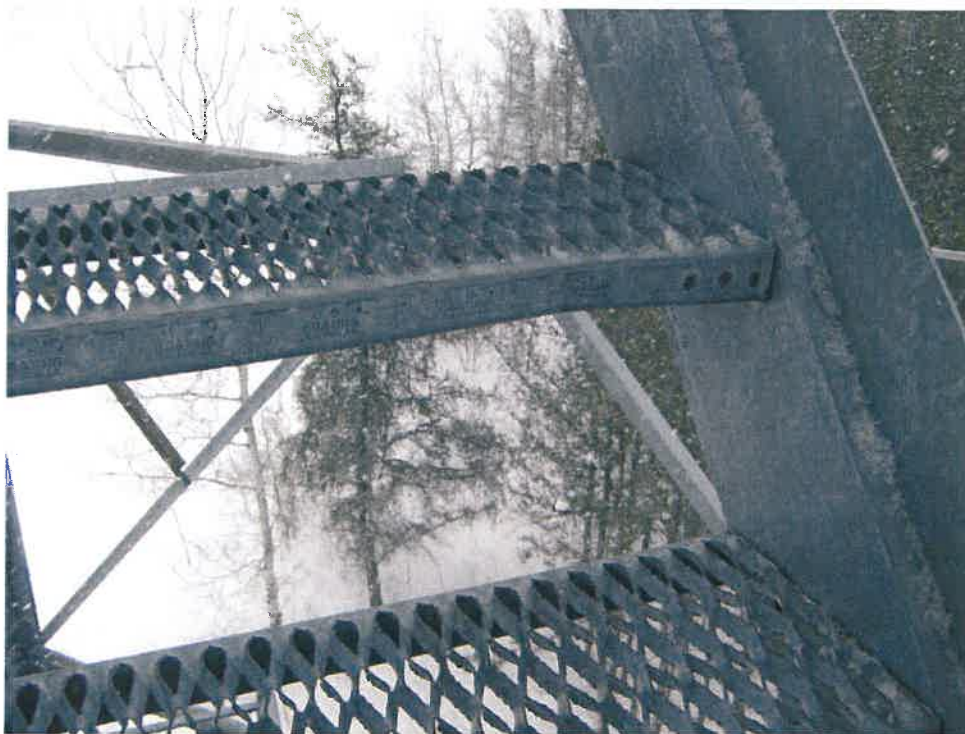
Photo #14: Damaged Step
