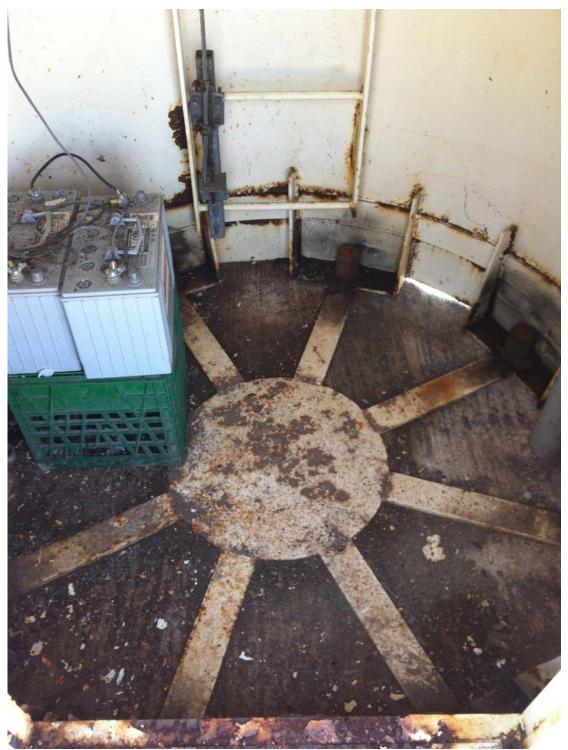
Figure 6 – Inside of tower, showing attachement to concrete.
