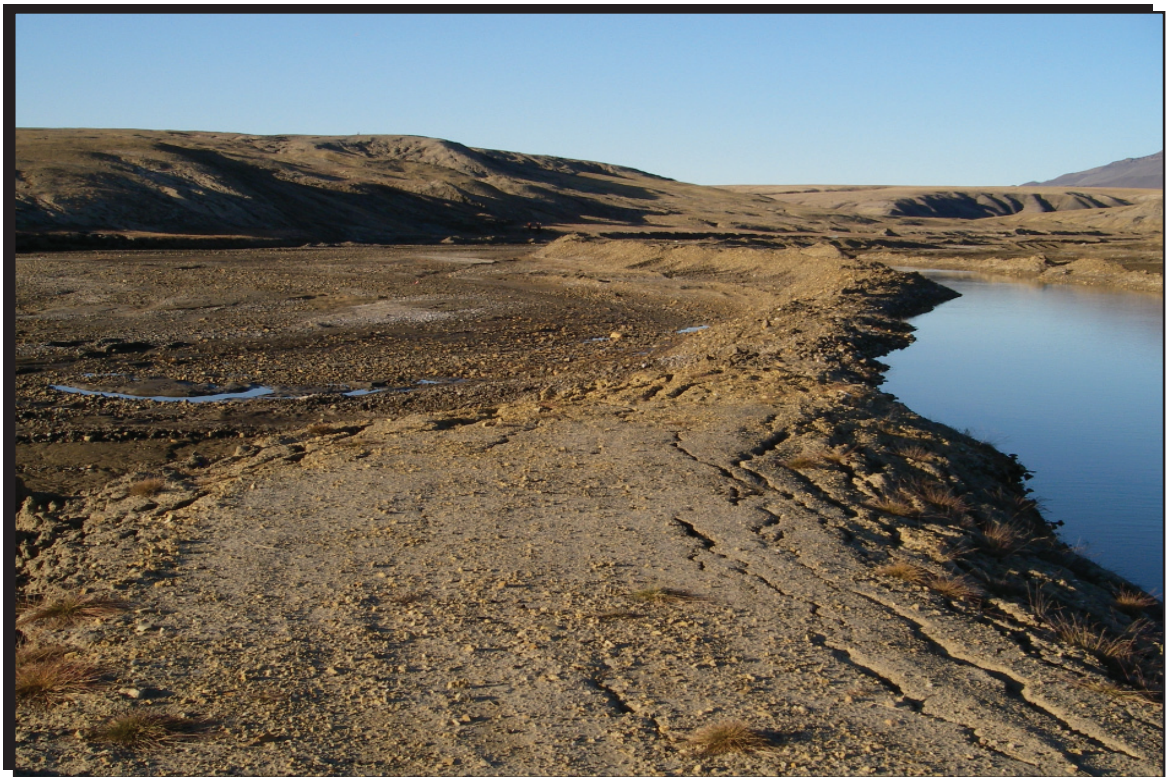
PHOTO 7: Seepage through water reservoir berms.
