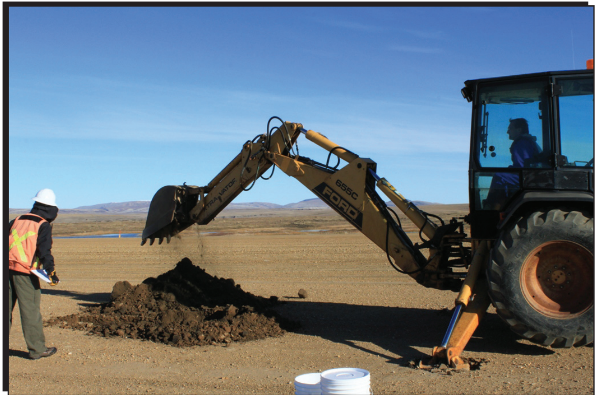
PHOTO 1: Test pit excavation in progress.
