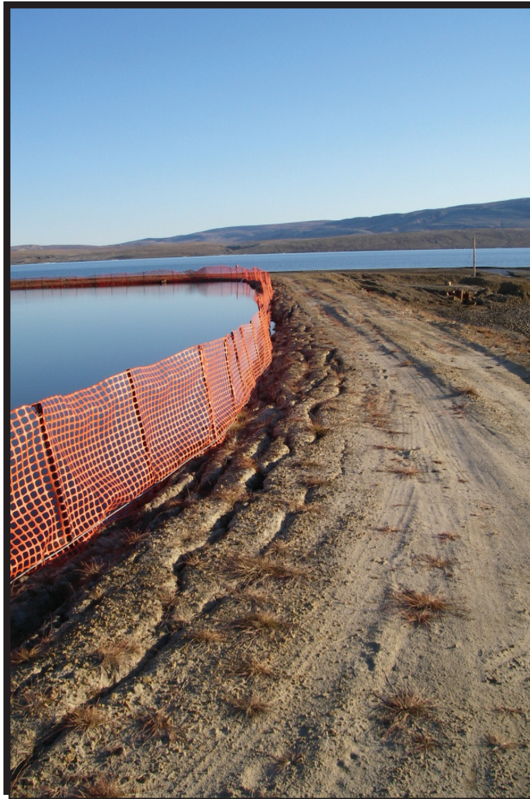
PHOTO 5: Existing reservoir berms showing instability and lack of freeboard.
