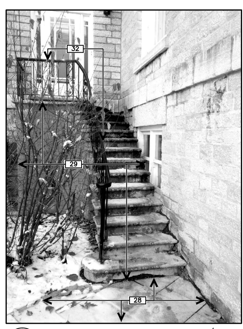
5 EXISTING PHOTO / PHOTO EXISTANT
