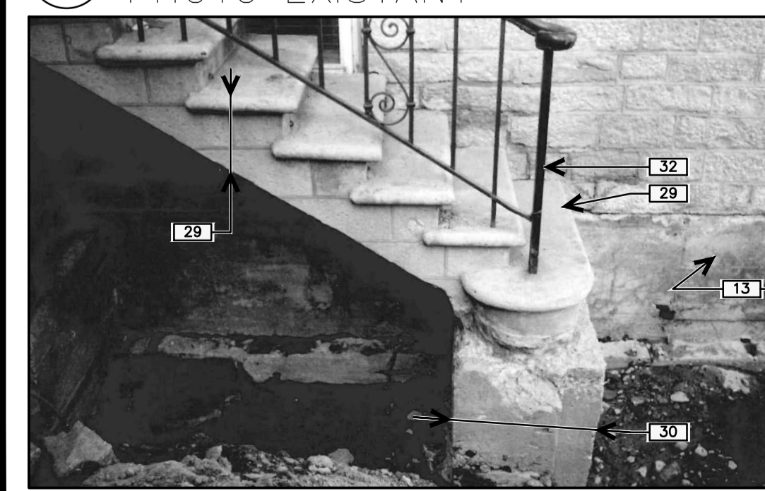
9 EXISTING PHOTO / PHOTO EXISTANT
