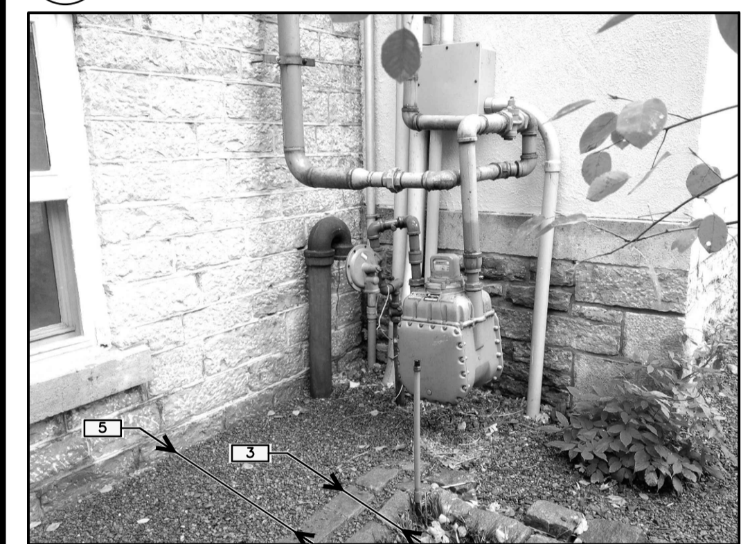
7 EXISTING PHOTO / PHOTO EXISTANT
